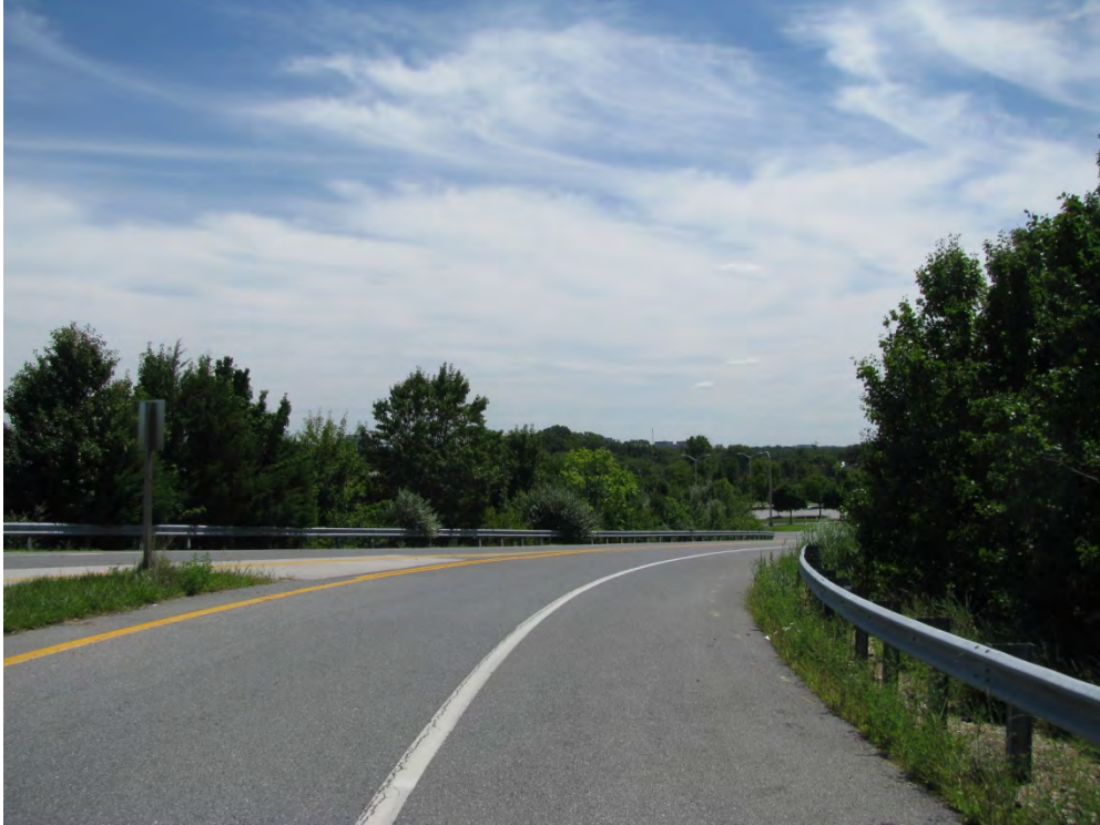
View looking southeast along Henkels Lane from Dorsey Run Road
