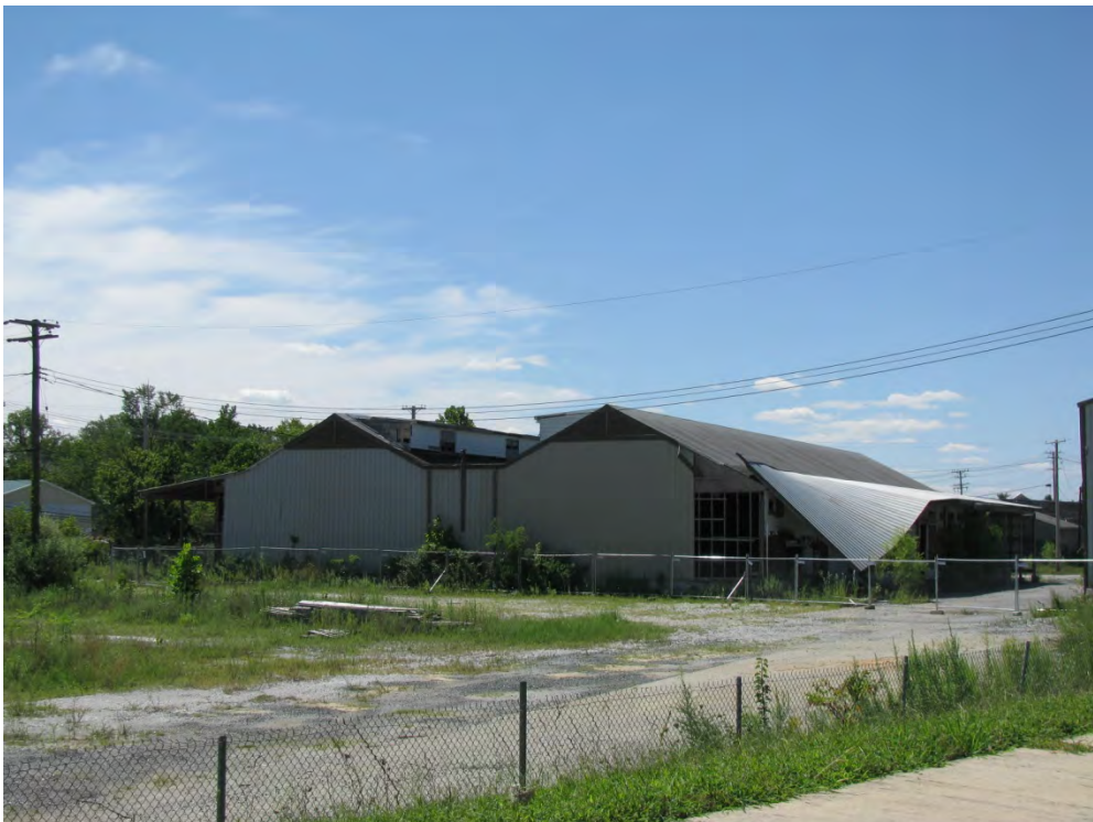
Additional view of existing buildings on the subject property
