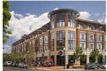
Example of columns overwhelming retail fronts (above)
