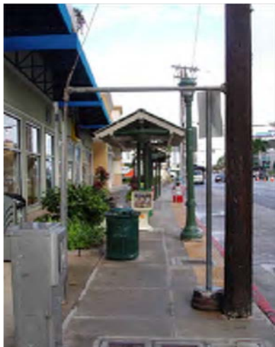
Example of a sidewalk that is narrow and crowded with obstructions (uncoordinated newspaper racks, furniture, street-lights, utility poles, transformers, bus shelters)
