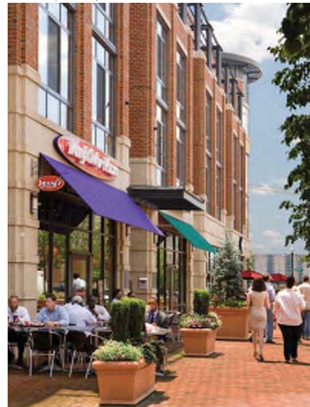
Good examples of ground floor treatments that include retail displays, outdoor dining and awnings for shade.
