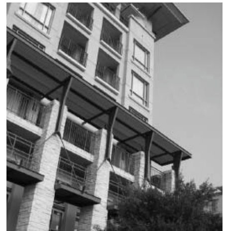
Good example of vertical variation from the street level base to the middle and the top where the building meets the sky with a thin overhang
