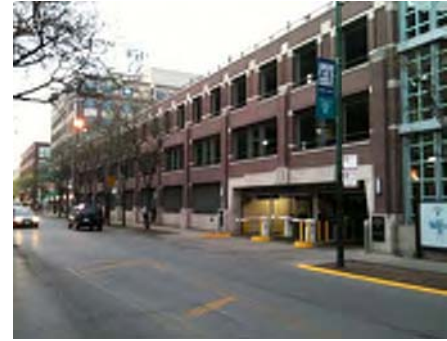
Example above of a parking garage that corresponds to its surrounding architecture.
