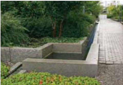
Rainwater is drained into the canal from the surrounding buildings via gutter planter as water feature.
