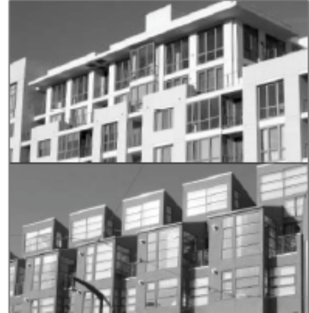
Good example of variety of units stacked vertically to create variation in massing
