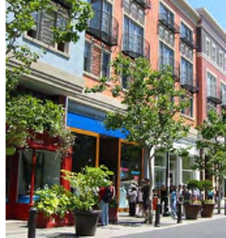
Example of allowing critical building columns to express themselves while balance of column architecture is engaged retail storefronts
