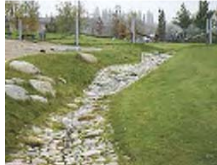
Example of surface Bioswale
