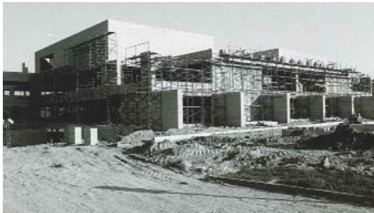
Concrete masonry unit solid walls
