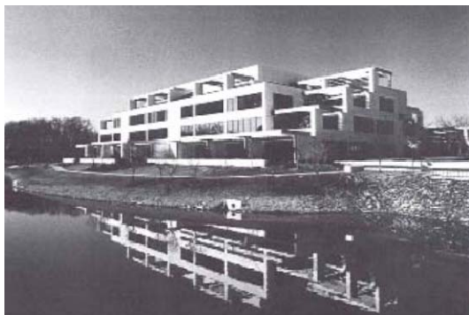
View from North-East
