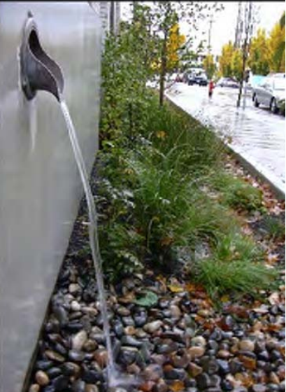
Rainwater is drained into bioswale
