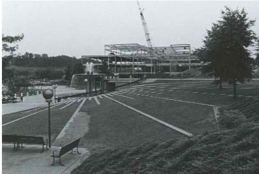
Steel framed building structure, under construction
