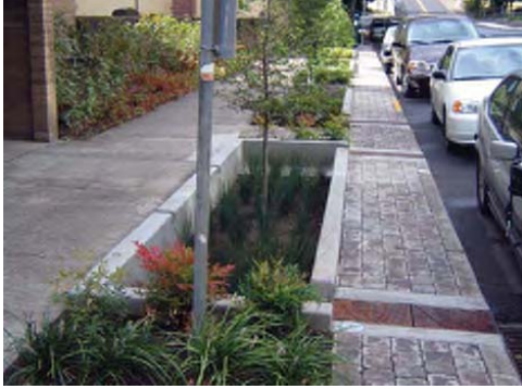
Street edge rainwater planter
