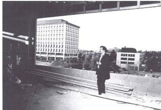
Frank Gehry inspects construction site
