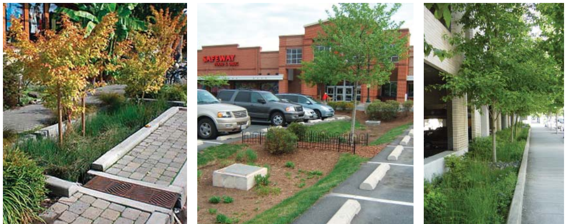
Figure 3Z: The photographs above illustrate a variety of storm water management and bio-retention techniques. The photo to the left shows how these facilities can be integrated into the overall site and planting design. The middle photograph shows a bio-retention swale integrated into a parking lot design. The photo to the right illustrates how street runoff can be captured and filtered in street tree planters.
