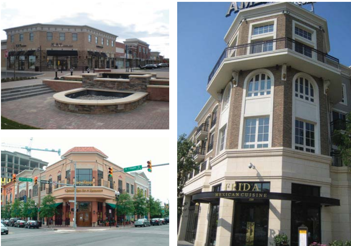
Figure 5C: These photographs illustrate how buildings located at intersections can be articulated to respond to these conditions. The photos also illustrate façades articulated with a “base,” “middle” and “top”.
