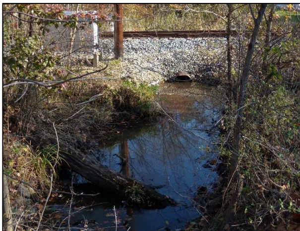
Photo 12. Outfall 3 draining to South Dorsey Run.
