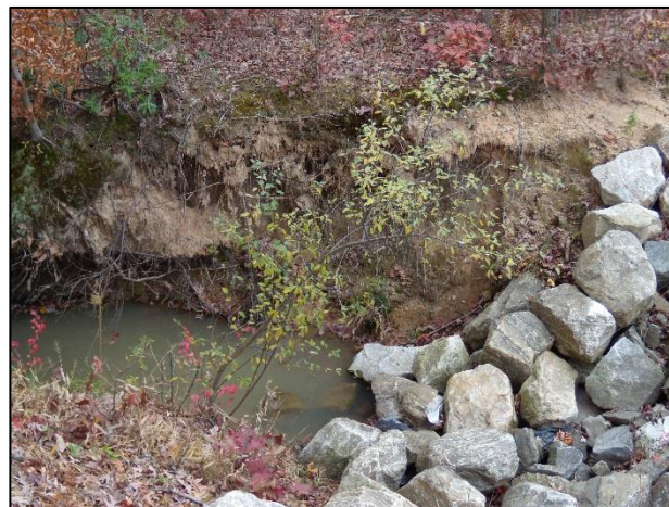
Photo 13. Outfall 4 draining to South Dorsey Run.
