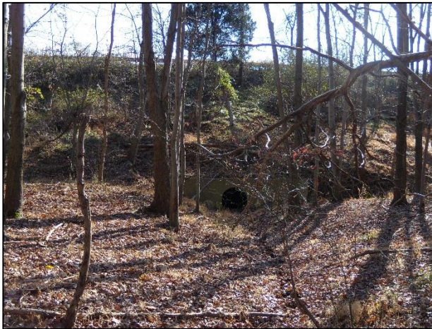
Photo 8: Stand 2 ephemeral channel draining to culvert under I-95.
