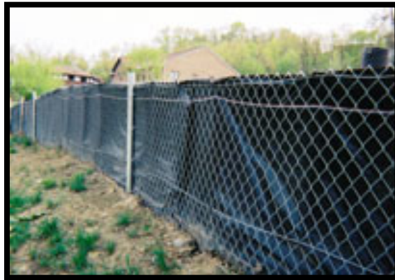
Super Silt Fence
