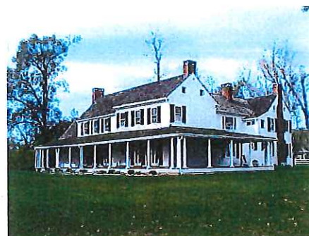
RICHLAND, CLARKSVILLE – white lap siding, gable roofs, divided-lite windows
