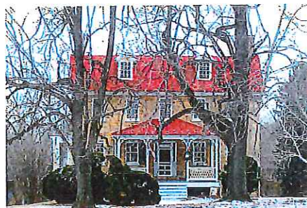
MONTROSE, CLARKSVILLE – stone masonry, red metal roof, roof dormers, hipped roof porch
