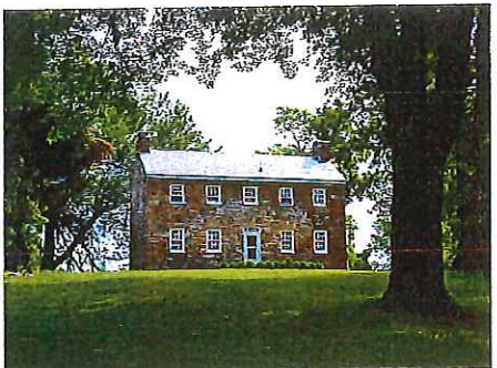
IVY HILL, MARRIOTTSVILLE – masonry, gable roof, divided-lite windows
