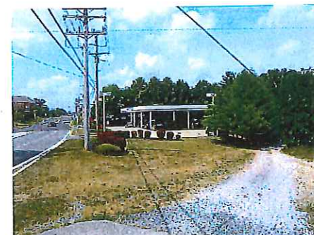
Existing gas station
