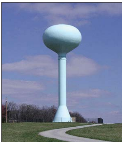
Howard County has nine water storage tanks within the Metropolitan District.
