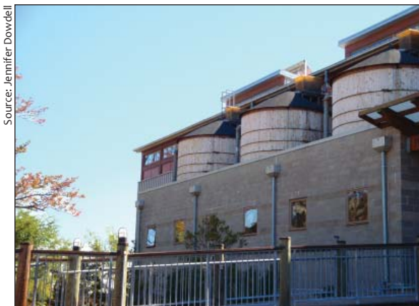
Cisterns at the Chesapeake Bay Foundation collect rainwater for nonpotable indoor uses.
