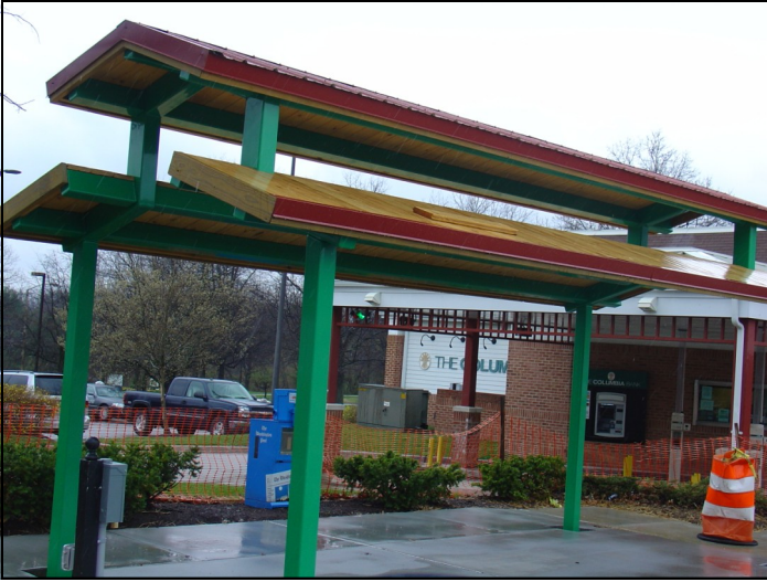
Robert Oliver Place Bus Stop Pavilion
