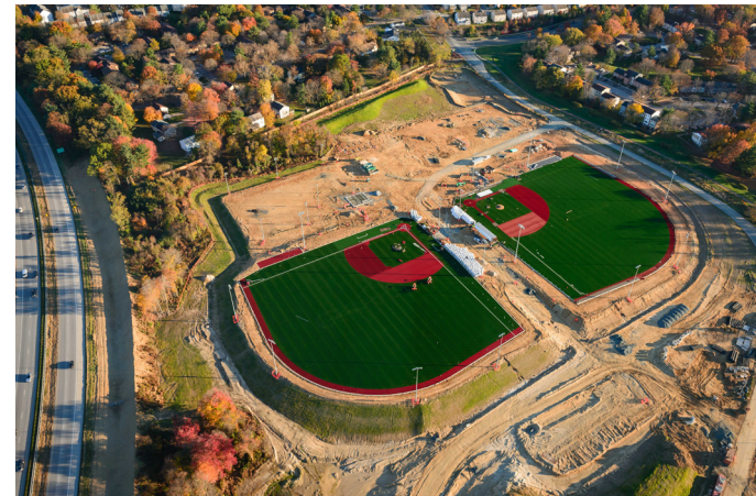
Blandair Park Phase 3 includes the maintenance building, an accessible playground, a backyard games area, shelter and restrooms.
