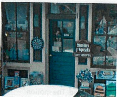
Figure 39 - Previously existing door prior to 2016 flood
