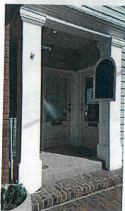
Figure 26 - Doors in April 2016
