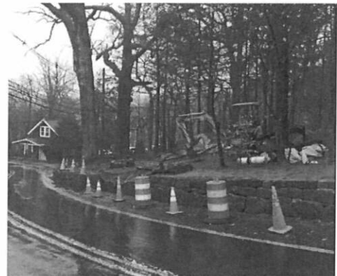
Figure 18 - Realigned wall. Note the increased width of the shoulder.
