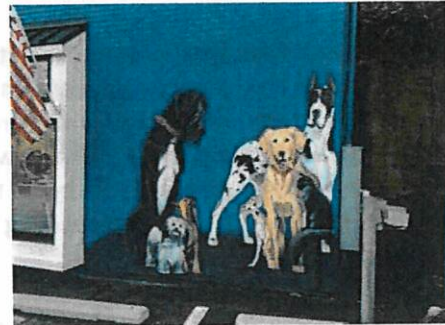
Figure 22 - Mural installed without approval
