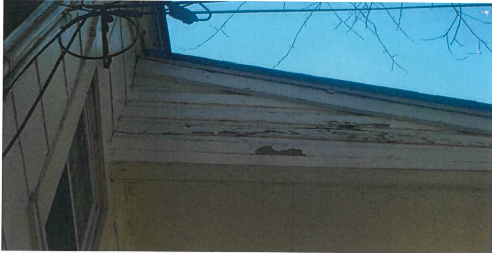
Figure 4 - German lap siding on porch.
