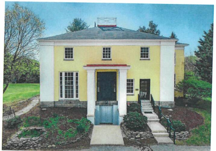
Figure 5 - Northwest elevation facing Mt. Ida and Courthouse parking lots
