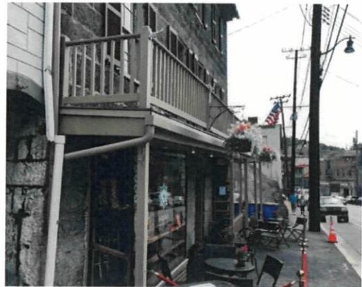
Figure 8 - View looking east
