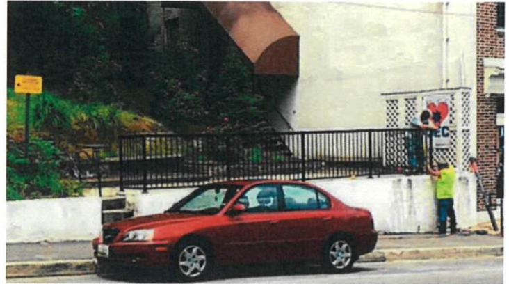
Figure 10 - After fence was installed.
