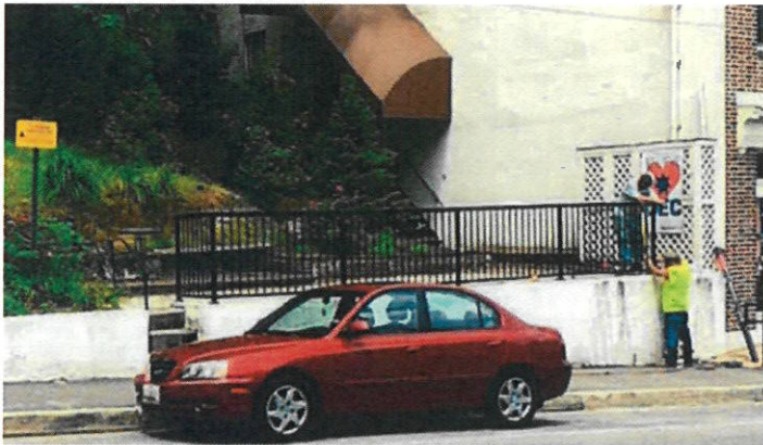
Figure 22 - Fence installed and approved in July 2020.
