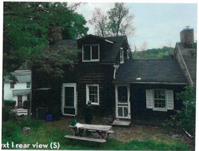
Figure 19 - Existing rear facade.
