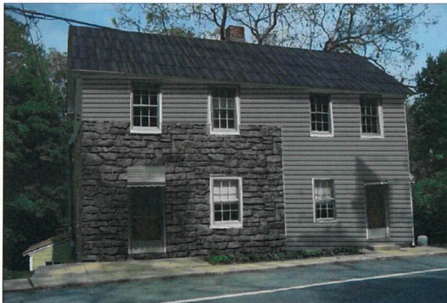
Figure 2 - Rendering of proposed alterations with solar shingles, restored gray siding and gray repointed mortar.
