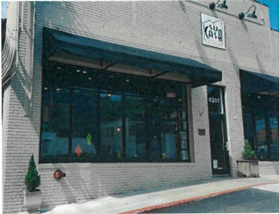
Figure 10 - Example of properly scaled awning.
