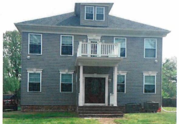
Figure 2 - Current condition of house.
