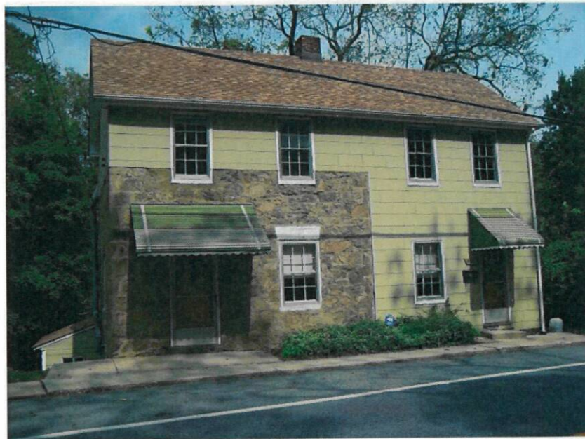
Figure 1 - Photo from application shows existing conditions prior to 2016 flood.
