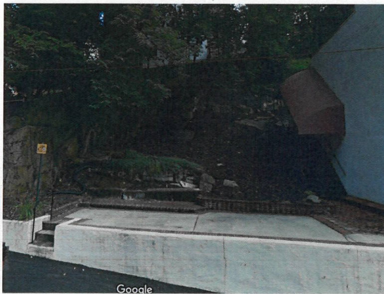
Figure 21 - Google Streetview 2018. Current landscaping did not exist then.
