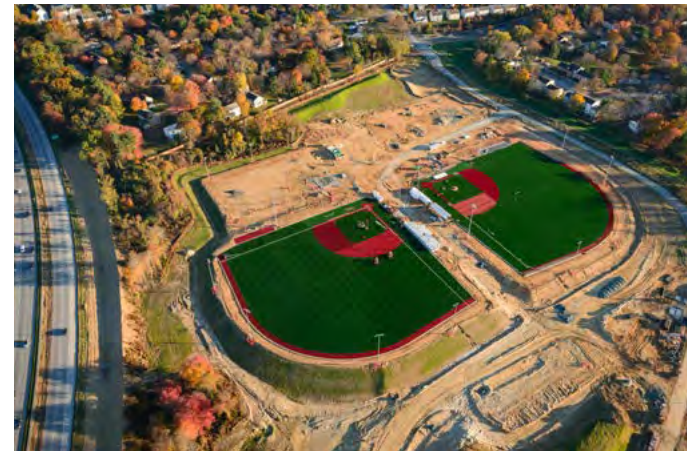
Blandair Park Phase 3 includes the maintenance building, an accessible playground, a backyard games area, shelter and restrooms.
