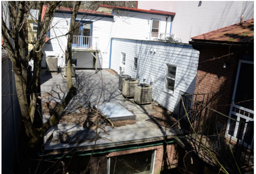
Figure 12 - Rear of 8109-8111, 8113 Main Street
