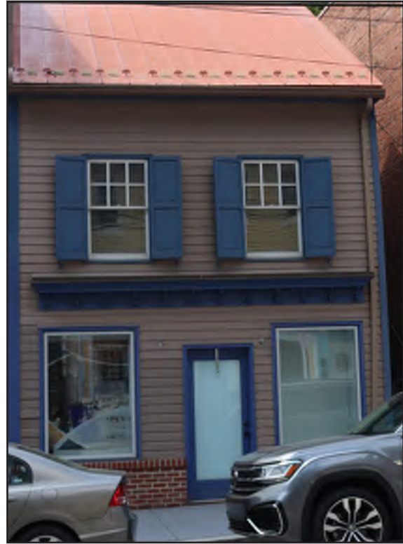
Figure 19: Facade of 8113 Main Street
