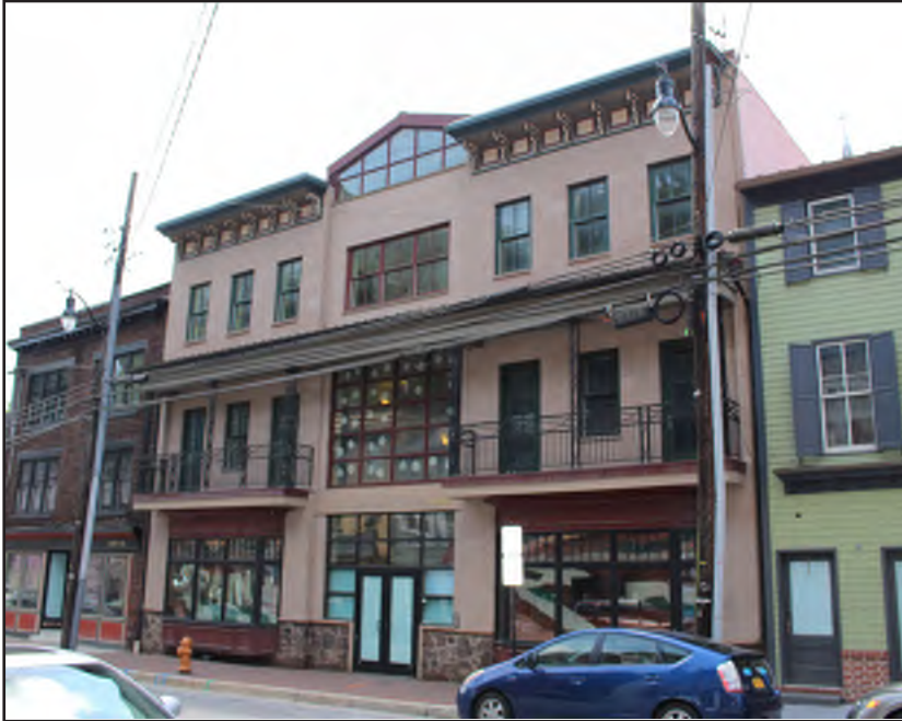
Figure 13: Facade 8095 Main Street
