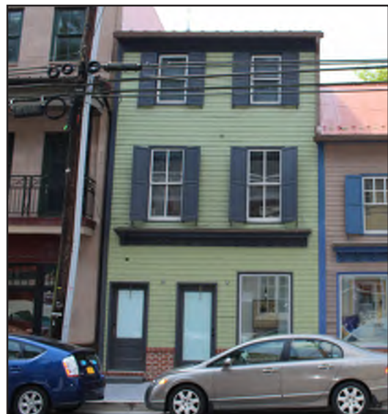
Figure 17: Facade of 8111 Main Street
