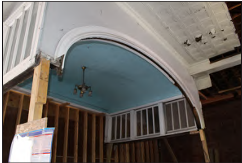
Figure 28: Pressed tin ceiling and remainder of storefront
