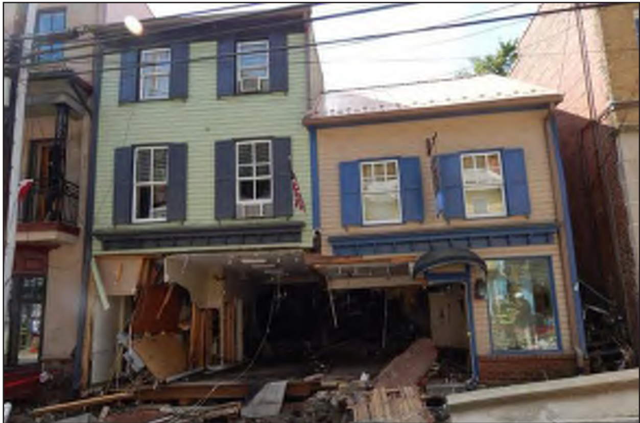
Figure 20: Photograph of 8109-8113 after the flood in 2016 (Ellicott City Patch)
