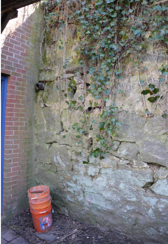
Figure 57 - Historic wall to be repaired
