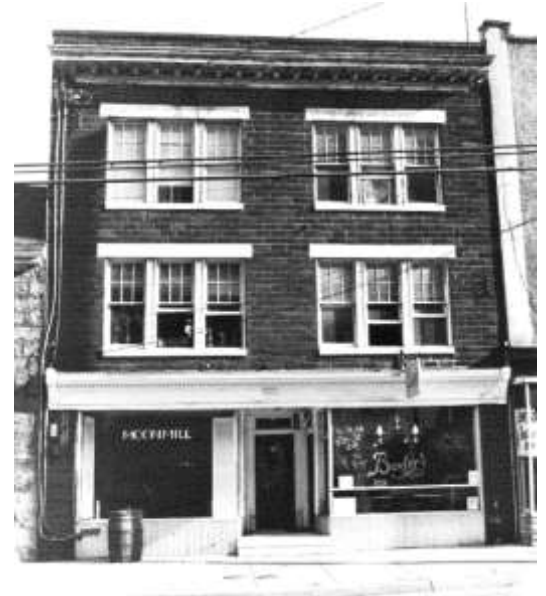
Figure 39 - Front facade in 1983
