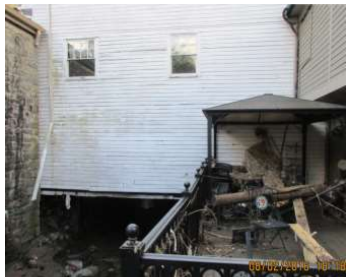
Figure 33 - Existing east side of building
