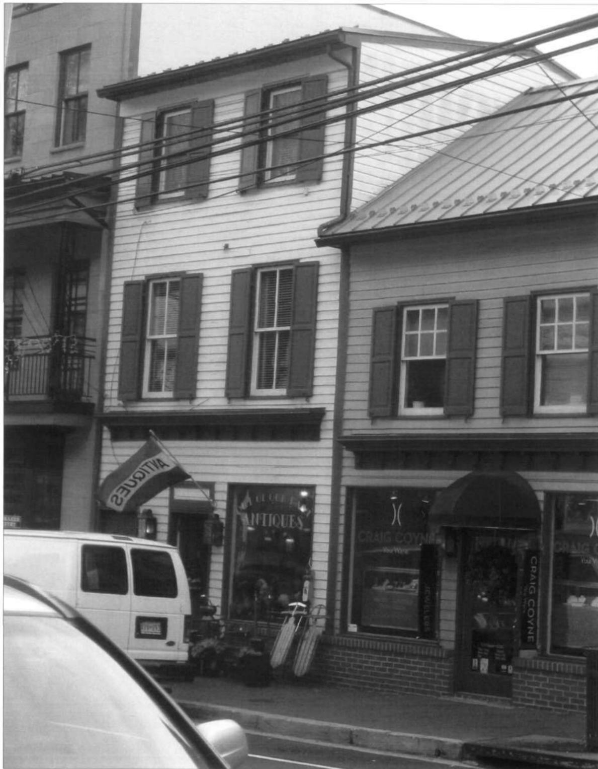
HO-586 Katydid 8109-8111 Main Street (MD 144) Photo by Jennifer K. Cosham, 12/5/2012 Northwest elevation
