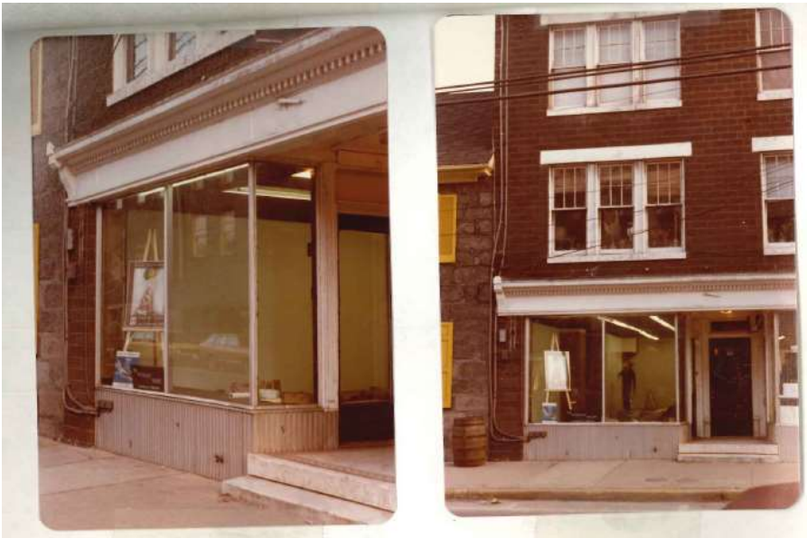
Figure 38 - Front facade in 1983
