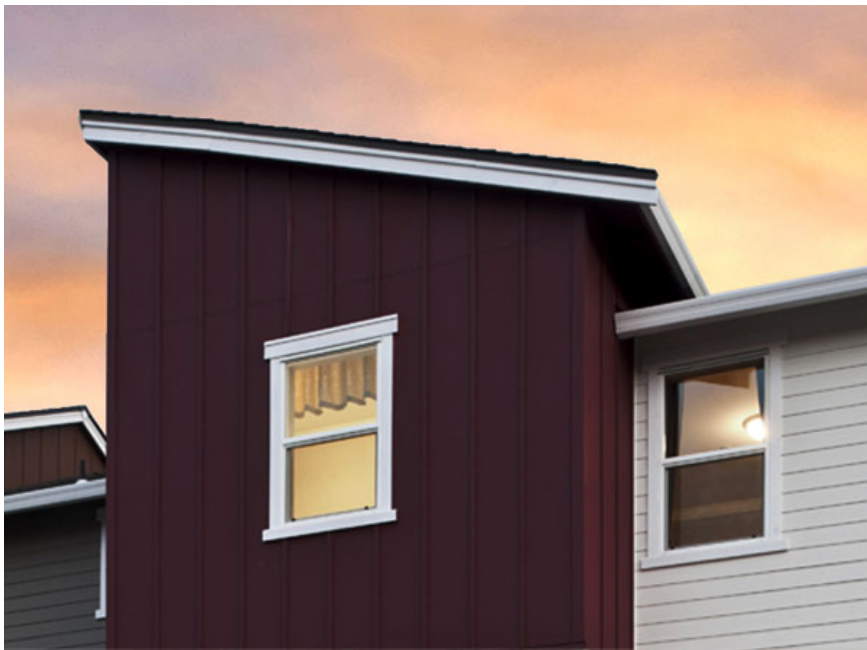
Image 8125.1 – Board and Baton composite siding, painted dark in color.
