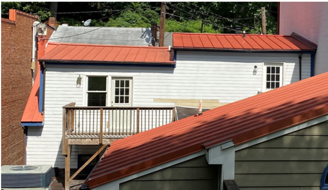
Image 8111-8113.1 – Rear Façade (currently wood siding)
