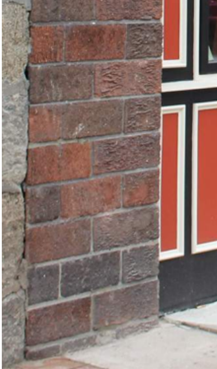
Image 8085.1 – Existing Terra Cotta
