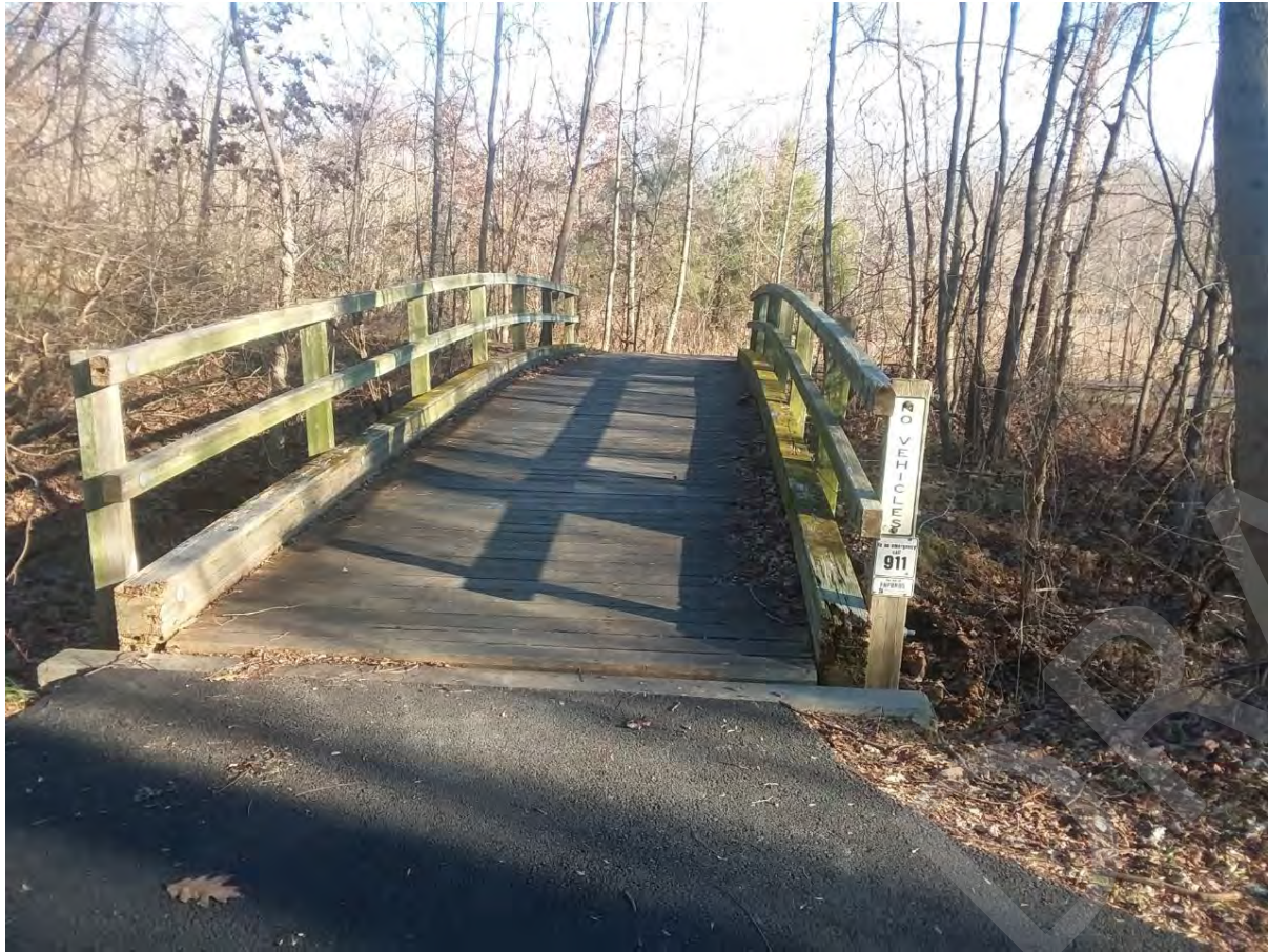
OPEN SPACE BRIDGE DECK & RAILING REPLACEMENTS
