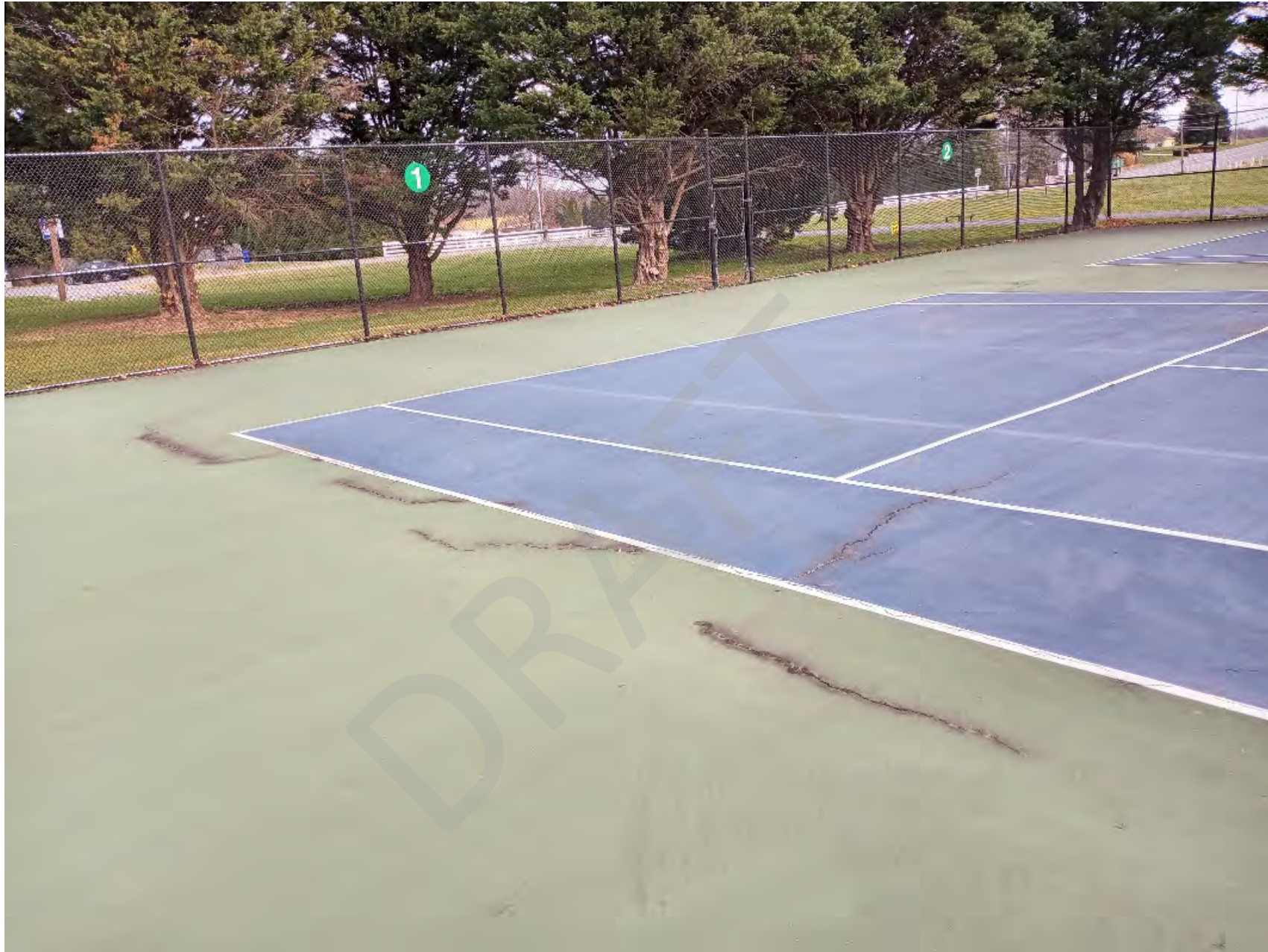
WESTERN REGIONAL PARK TENNIS COURT RESURFACING
