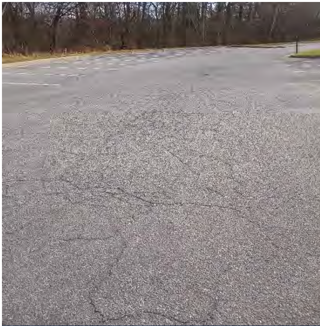
ATHOLTON PARK ROADWAY & PARKING LOT ASPHALT PAVING
