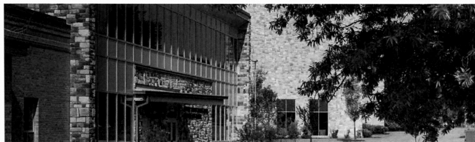
Current Building, c. 2021
