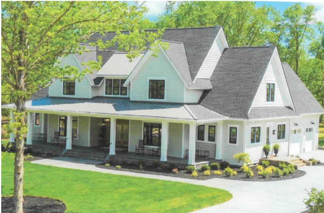
Figure 35 - Side view of house showing location of garage
