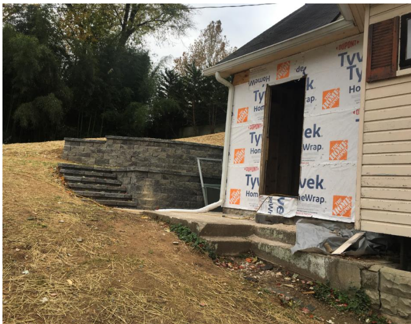
Figure 19 - View from the side of the house.
