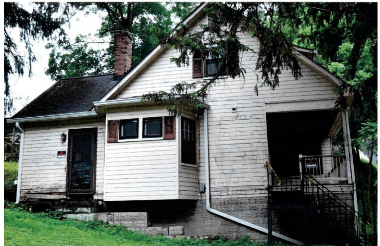
Figure 28 - Location of some existing gutters and downspouts on building.
