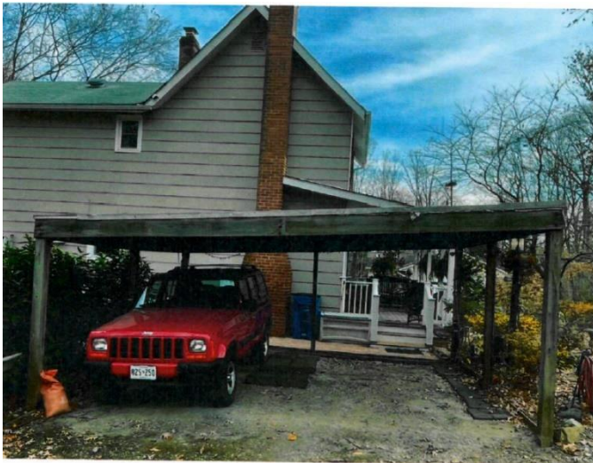
Figure 1 - Existing carport located to the rear of house.
