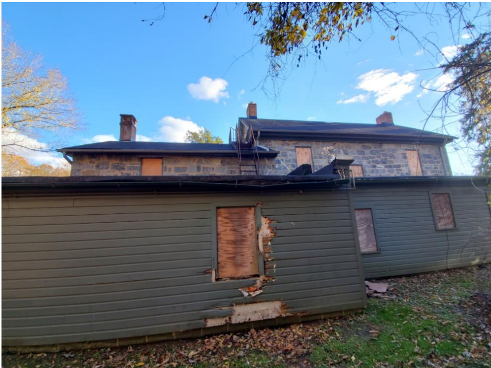
Figure 7 - Existing rear of structure.
