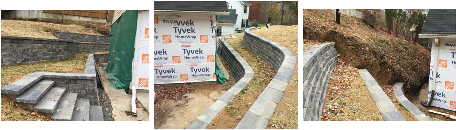
Figure 20, 21, 22 - Rear retaining wall views.
