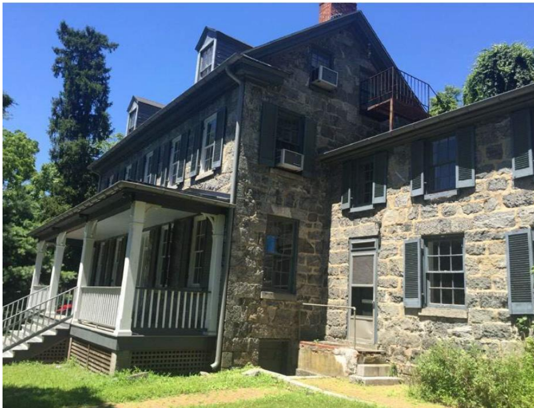
Figure 4 - Front (south) facade with porch.
