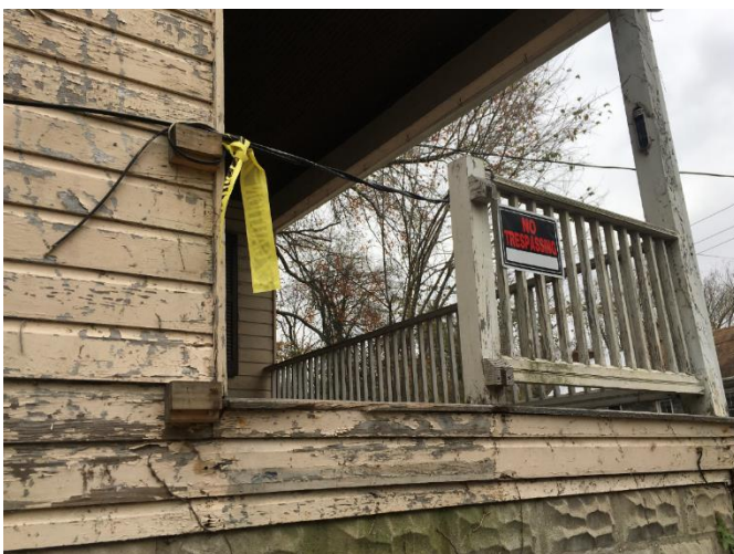
Figure 23 - Side view of front porch where steps would connect.
