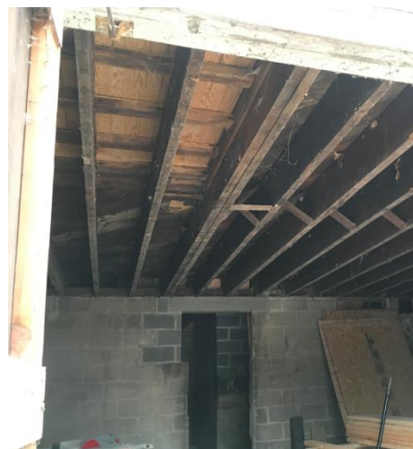
Figure 24 - View of porch from garage below.
