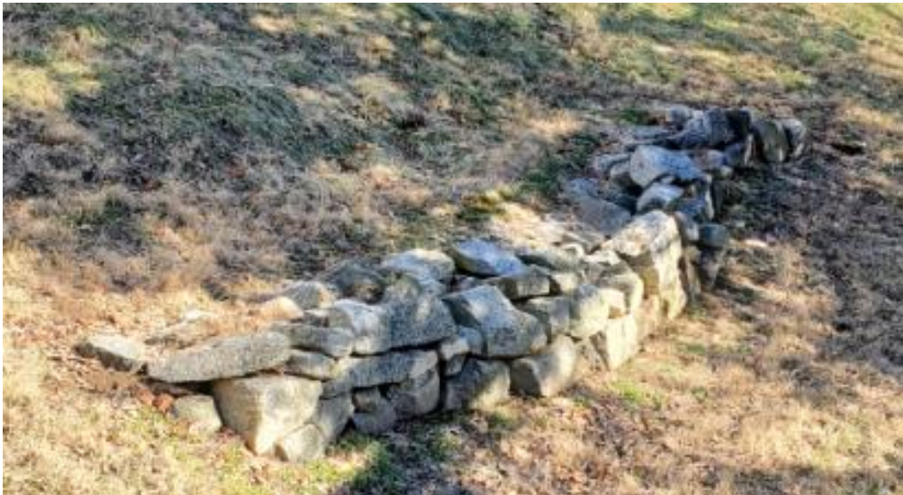
Figure 18 - Stone to be used in a stacked retaining wall at Court Avenue.
