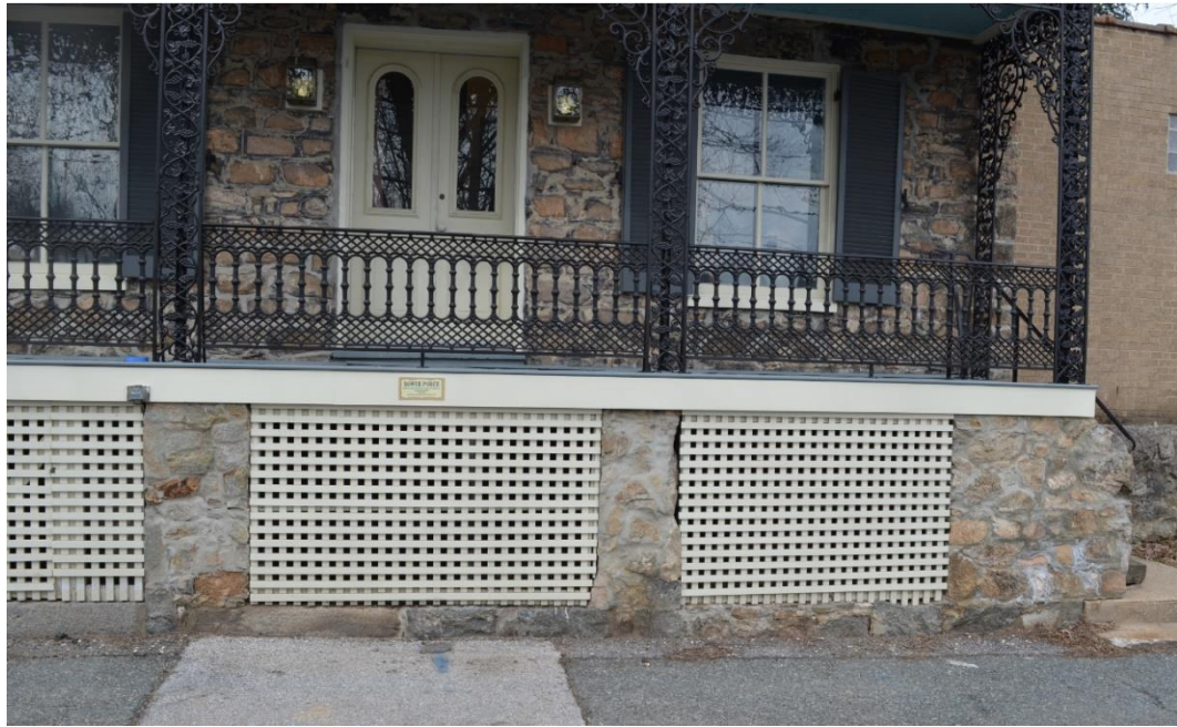
Figure 13 - Sign is taped temporarily on building to demonstrate installation location.
