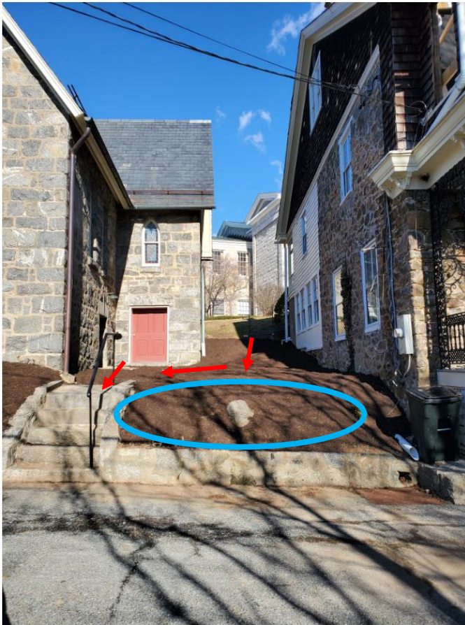
Figure 17 - View from Court Avenue looking up to Park Avenue staircase. Red arrows show approximate location of stepping stone pathway. Blue circle shows area to be retained with stone from property. Black metal railing to be added in this area to prevent someone from falling on to the street.
