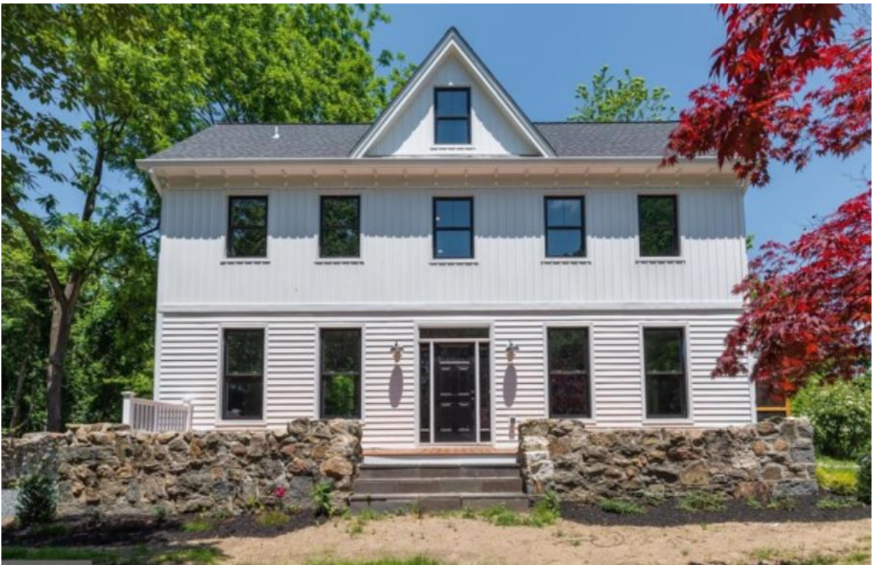
Figure 2 - Current condition of historic house after renovation.
