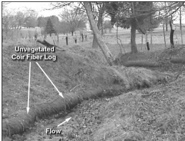
Figure 1: Coir fiber log prior to plant installation
