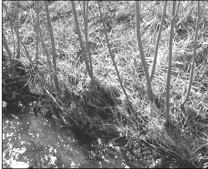
Figure 3: Fascines installed behind a coir fiber roll
