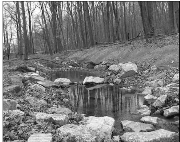
Figure 2: Streambank shaping in combination with boulder revetment and rock vortex weirs
