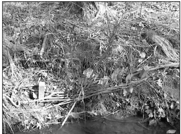
Figure 2: Fascines installed along a streambank
