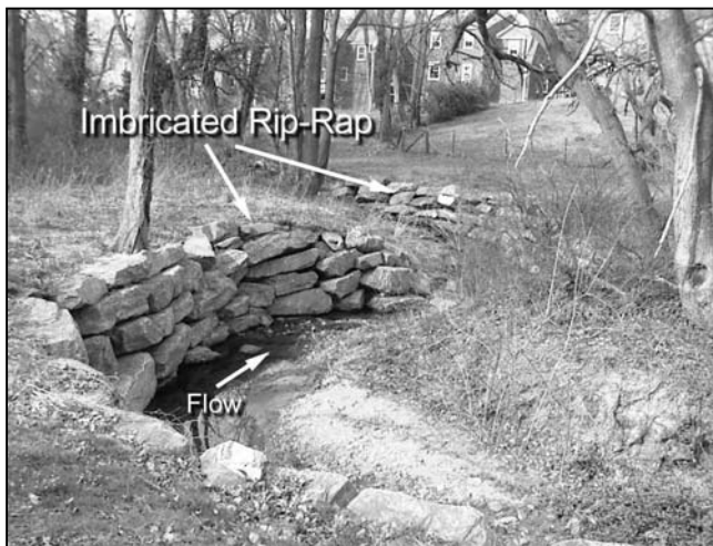
Figure 1: Imbricated rip-rap revetment protecting utility infrastructure
