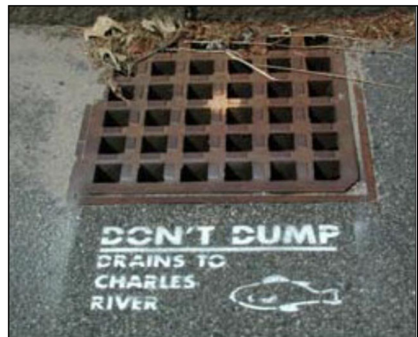
Figure 1: Storm Drain Marking
