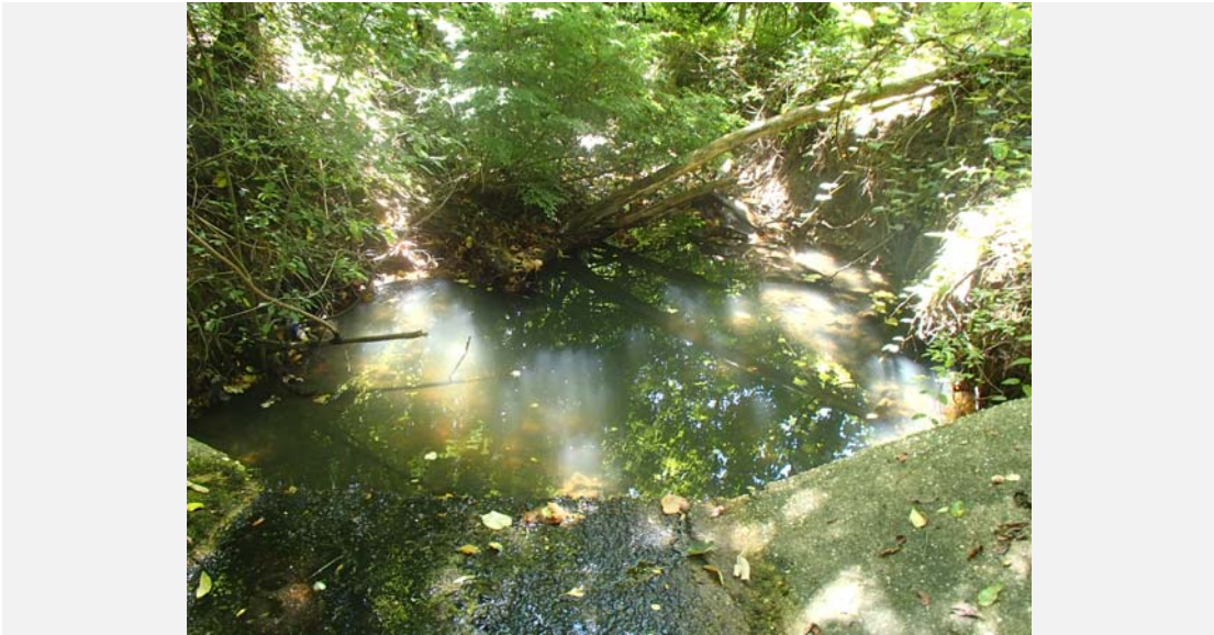
At outfall pipe looking downstream.
