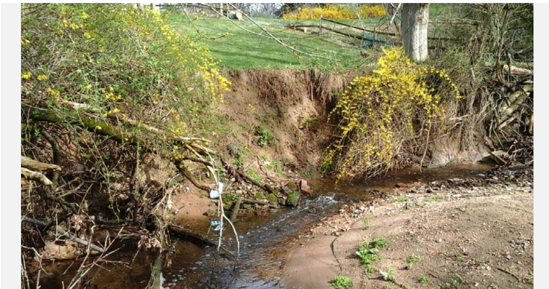
Erosion occurring along the right bank. Mowing is occurring along the bank in a private residential yard abutting the stream. Bank height is approximately 4.5 ft.
