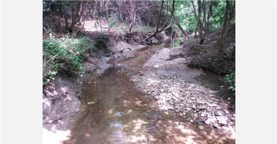
Undercut and eroding banks with no surface protection and shallow root depth; deposition as bar deposits.
