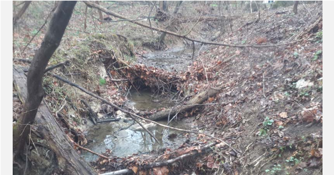
Facing upstream towards headcuts and debris jams.
