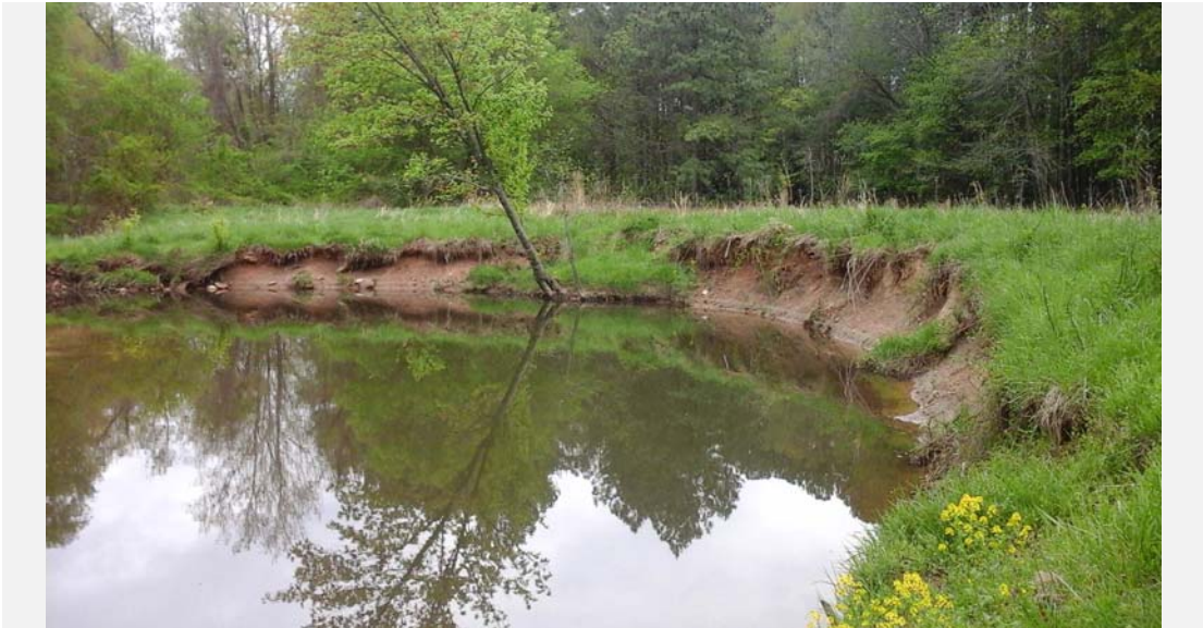
SR-59 facing downstream at severe bank erosion.
