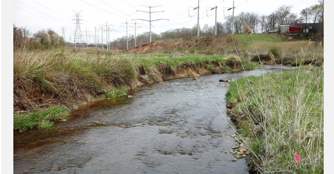
Facing downstream from the assessed channel. Downstream channel was not assessed, but should be considered as part of the stream restoration.
