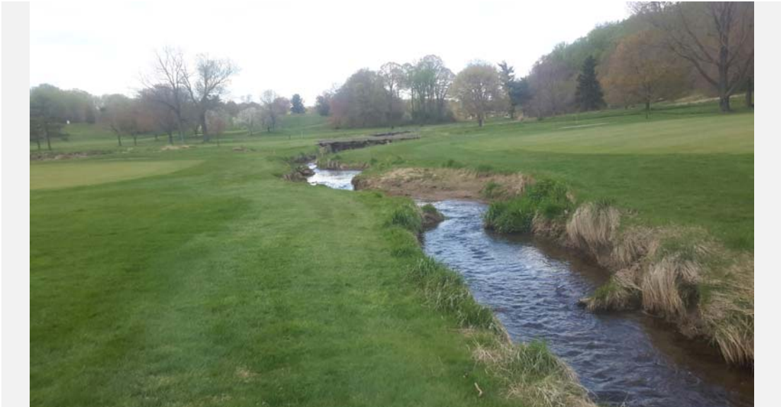
Facing upstream, poor root density and no cover.
