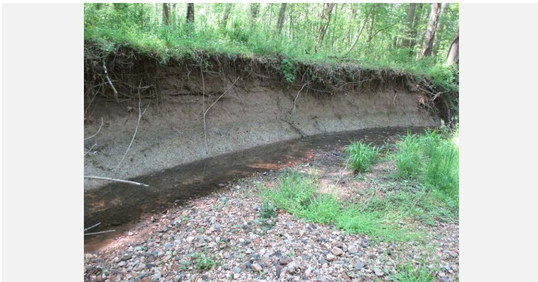
Erosion occurring along the right stream bank. Bank height is approximately 5 ft. Photo taken approximately 250 ft. upstream of the stream's confluence with the main stem of the Little Patuxent River.
