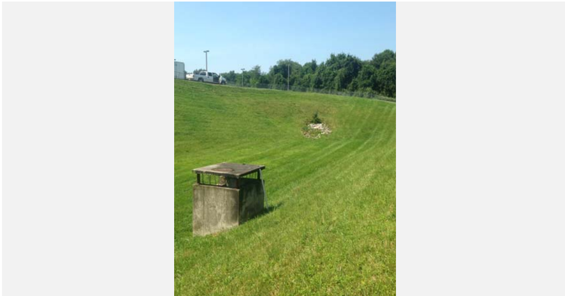
View south from embankment behind riser.
