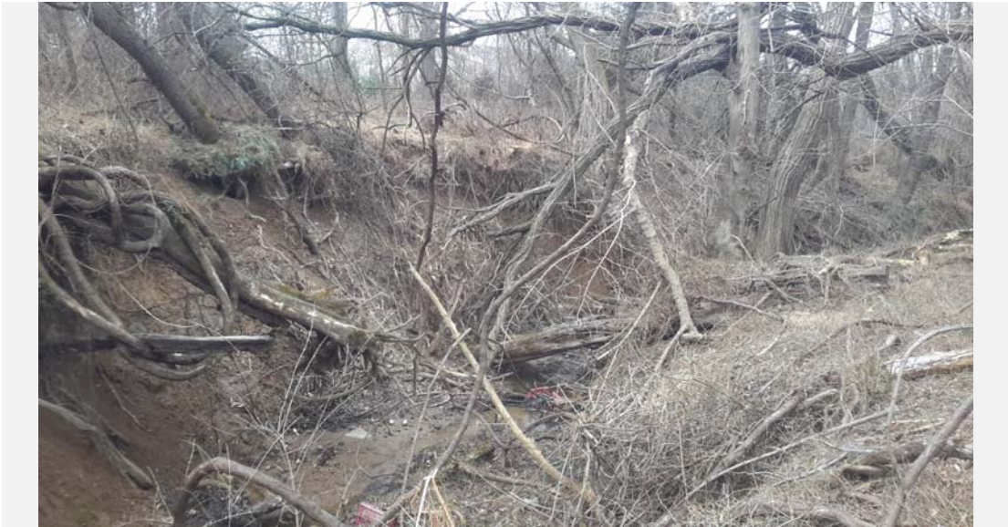
Facing downstream: channel erosion and debris.
