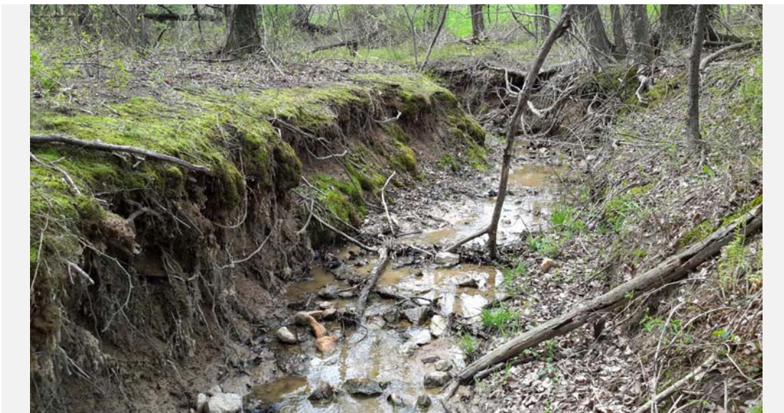
Facing upstream, little protective cover on the right bank (looking downstream).
