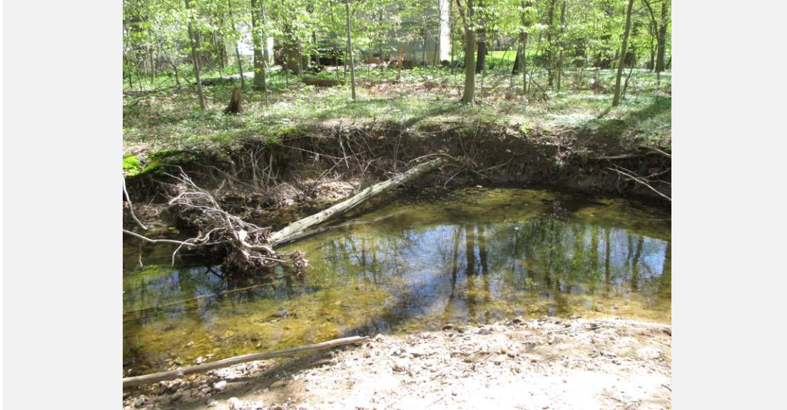
Cut bank erosion occurring along the left bank. Photo taken approximately 250 ft. upstream of Hesperus Drive. Bank height is approximately 4 ft.
