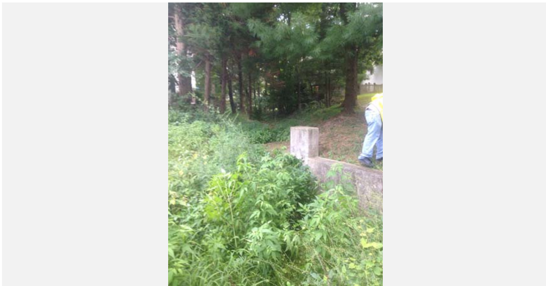
Standing at south end looking downstream.
