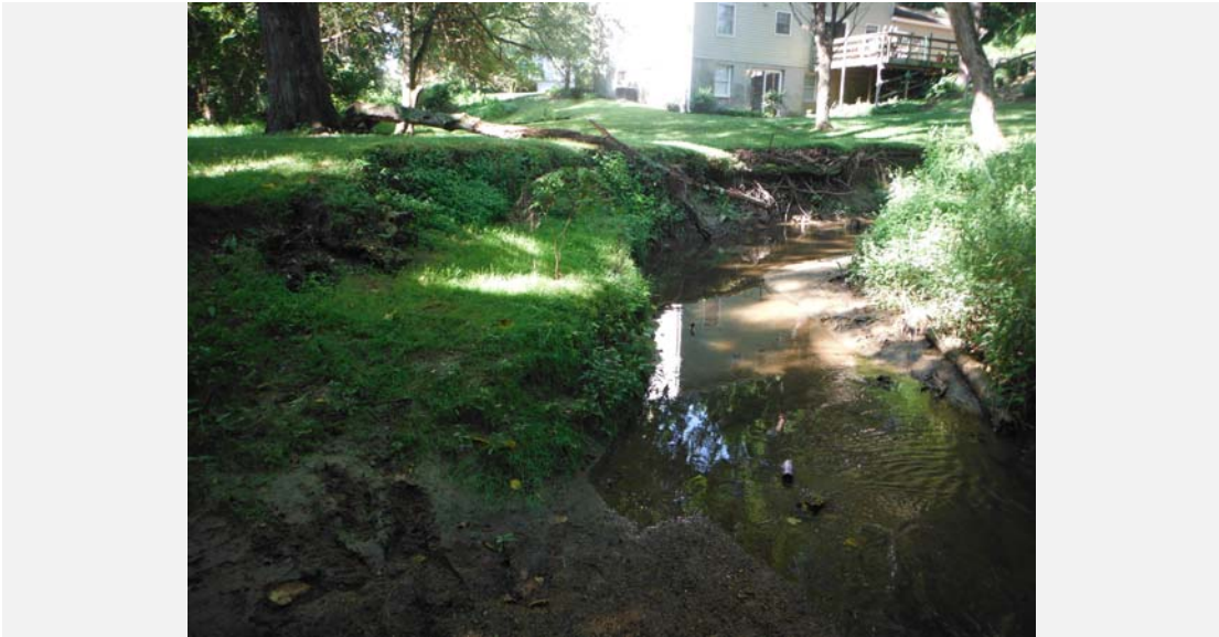
Bench establishment at approximately 2 ft. in height.
