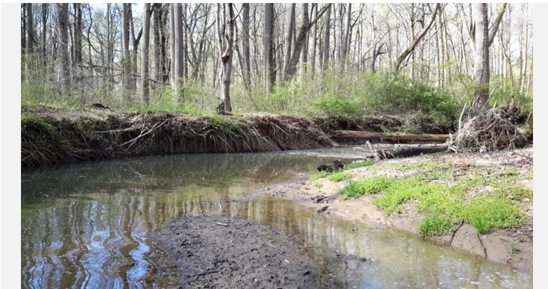
Facing downstream at a tight bend in the stream, a deep pool forming with little to no protection on the left bank (looking downstream).
