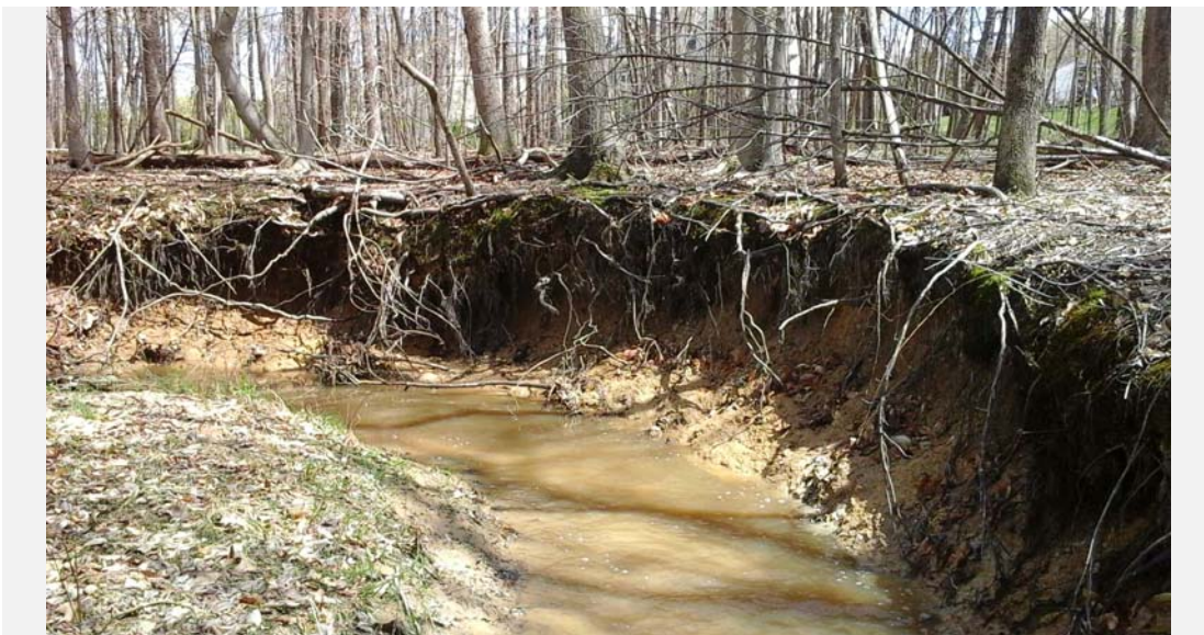
Facing upstream showing a high, raw eroded left bank (looking downstream).
