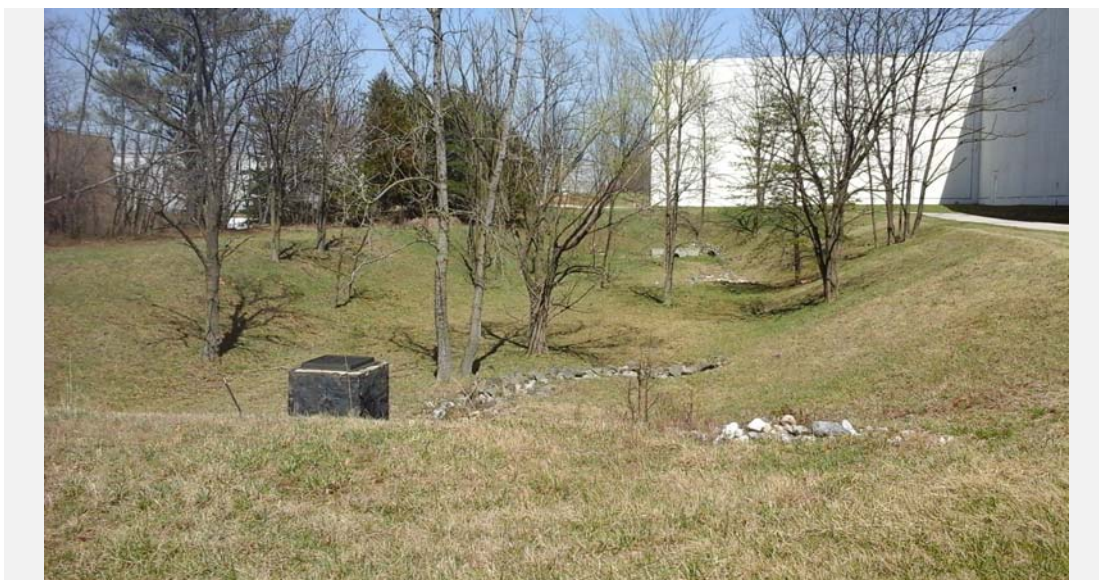
Looking north toward the facility from the embankment.
