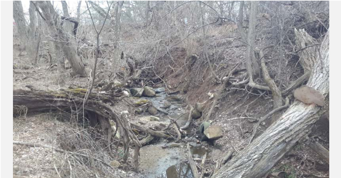
Facing upstream: steep bed slope, fallen trees, and eroded banks.
