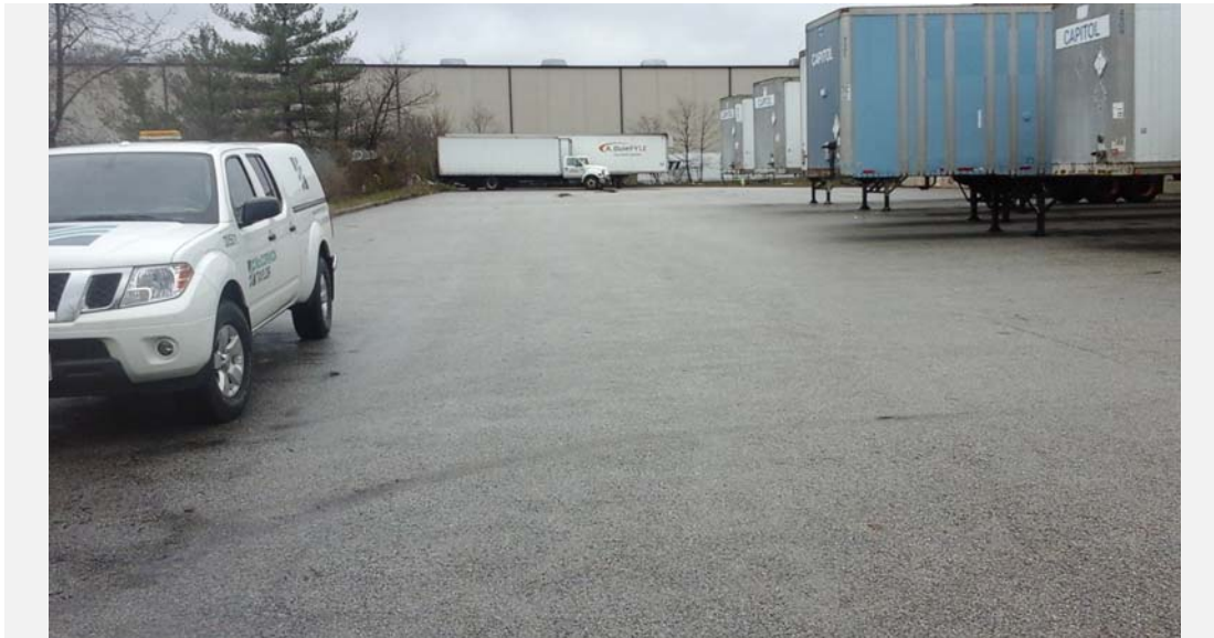
Looking east toward the existing clogged inlet to be used as the facility outfall.
