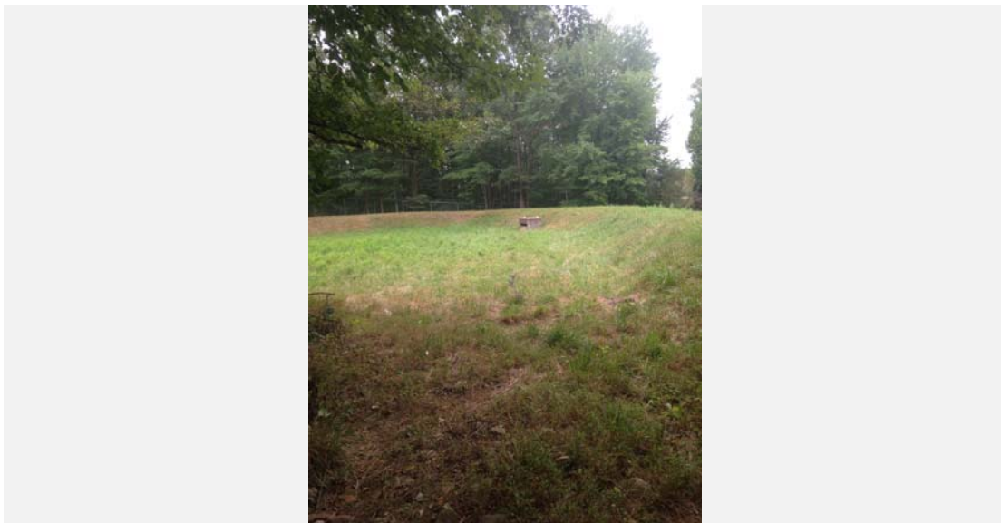
The facility bottom and outlet riser from the access.
