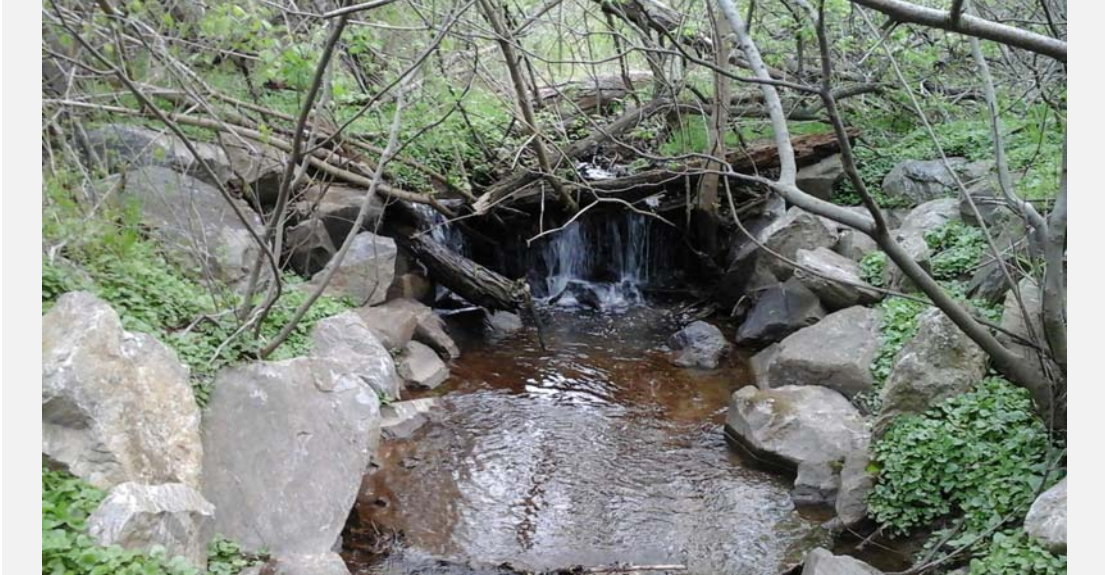
SR-55 facing upstream at riprap channel alteration and 3.5 ft. tall headcut.
