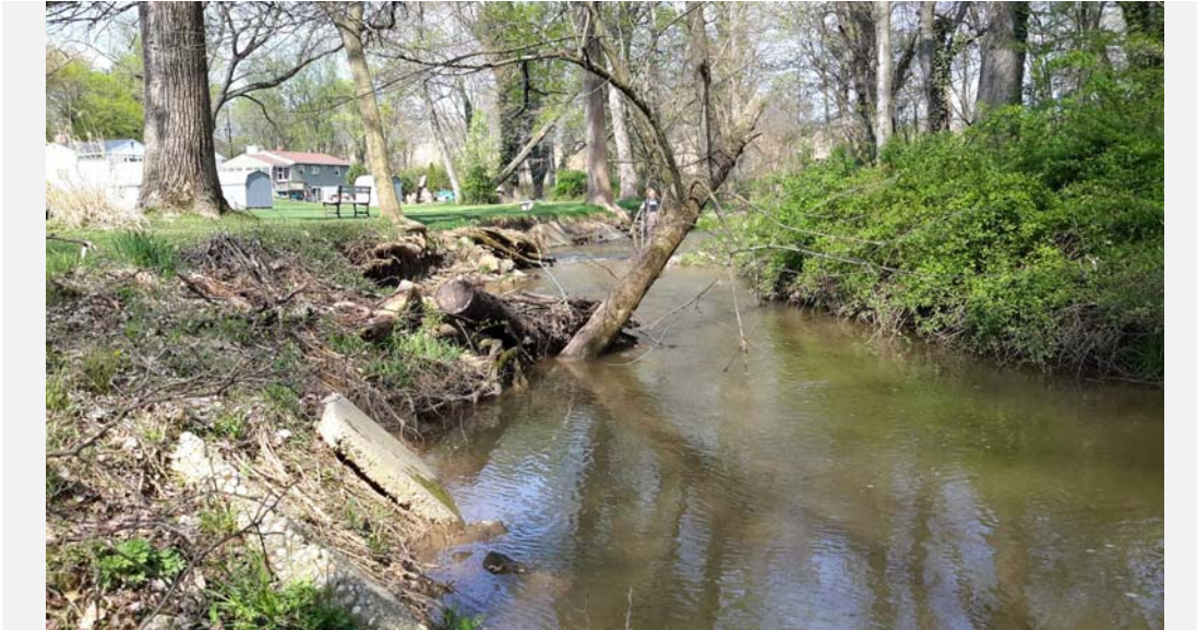
Facing upstream, concrete rubble presumably acting as bank protection.
