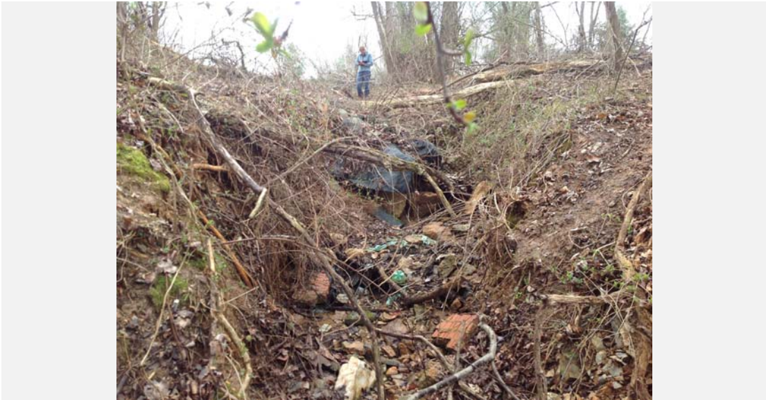
Upstream view of eroded channel.
