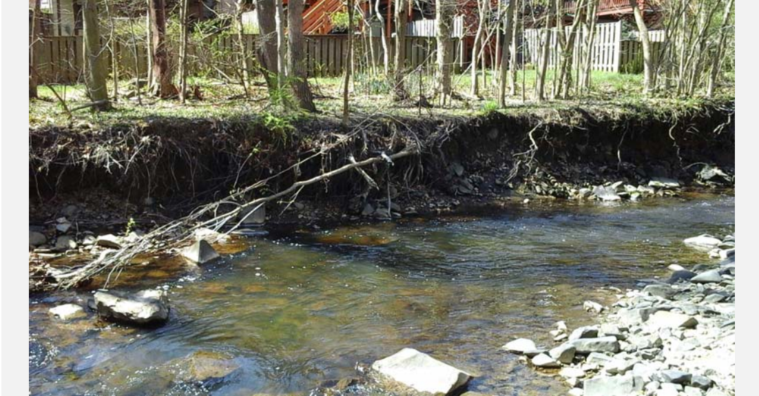
Facing upstream, erosion occurring on the right bank (looking downstream) with homes and properties close to the stream.
