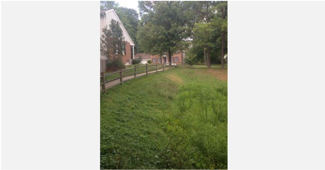
Standing on outlet headwall looking upstream.
