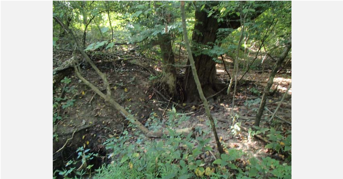
The 20 in. diameter box elder at the top of the eroded section, looking upstream.
