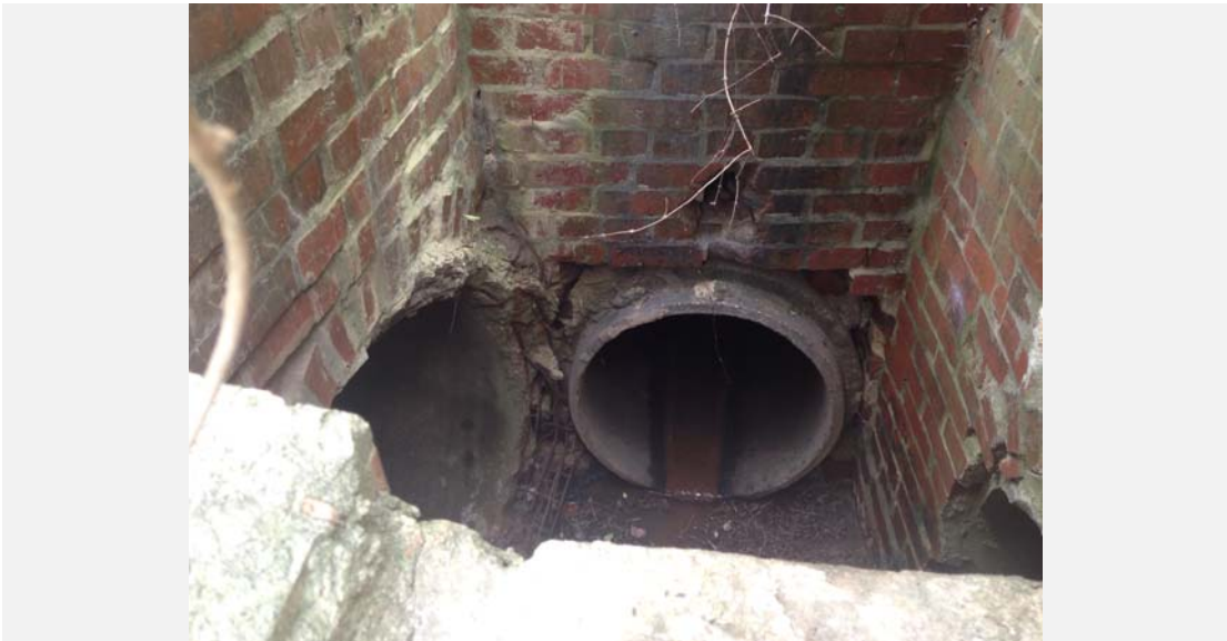
Brick junction box downstream of site.
