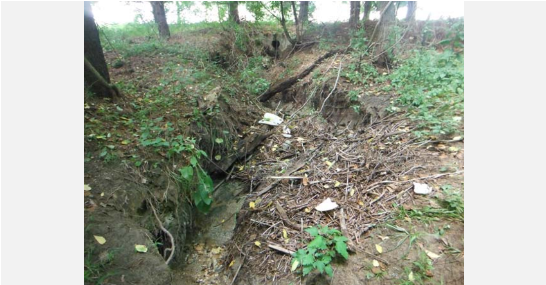
Incised and eroding outfall channel.
