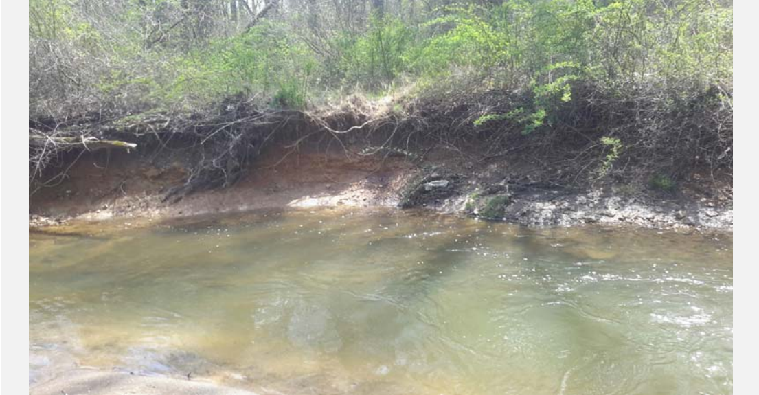
Erosion on right bank, vertical banks with poor root depth.
