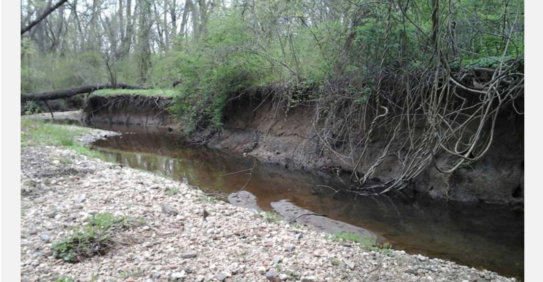
SR-54 facing downstream at severe bank erosion.
