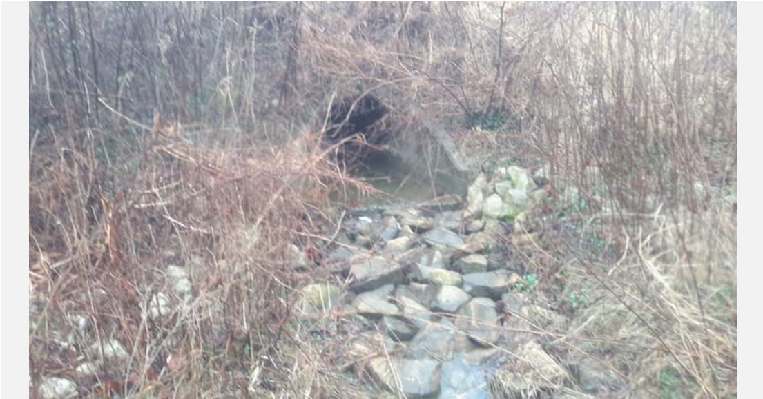
Facing upstream towards outfall.
