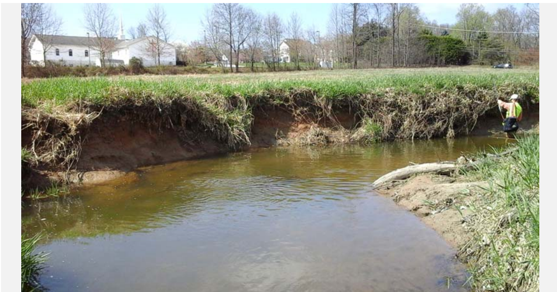
Looking upstream at a tight bend in the stream creating a deep pool with high banks with little to no cover.
