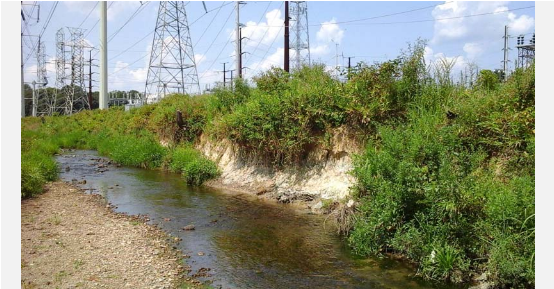
Facing upstream, recent bank failure and surrounding overgrown vegetation.
