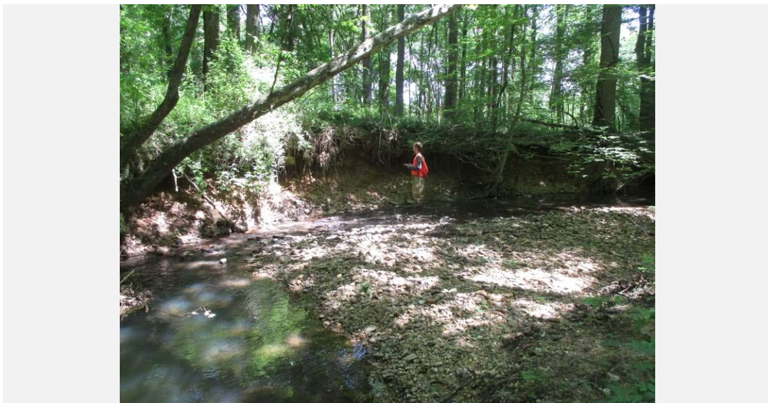
Erosion occurring along the right stream bank. Bank height is approximately 6.5 ft. A large cobble bar is present on the left side of the stream.
