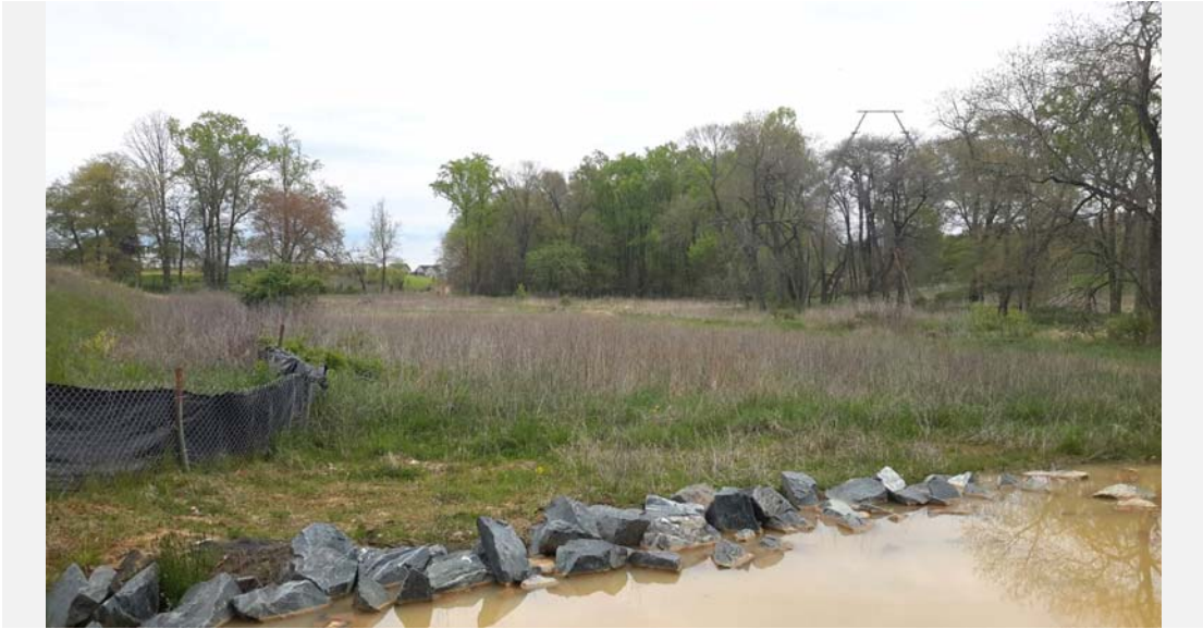
Tree planting area looking east. Riprap lined outfall from stormwater pond to the left visible in foreground.
