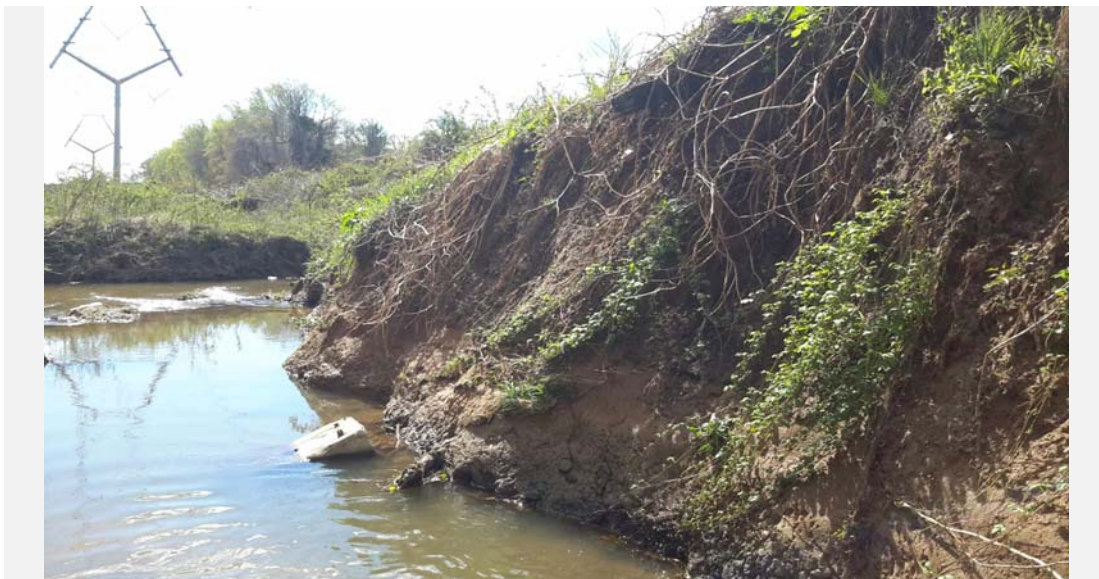
Facing downstream, very high eroded banks cutting into the hillslope near the school.
