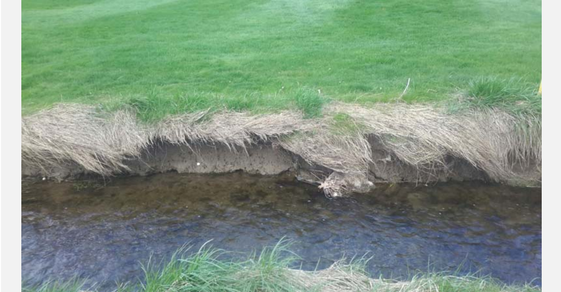
Erosion on left bank with poor root depth.
