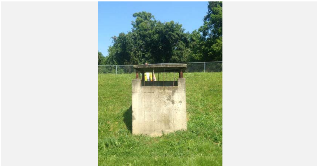
Facility looking west from embankment.
