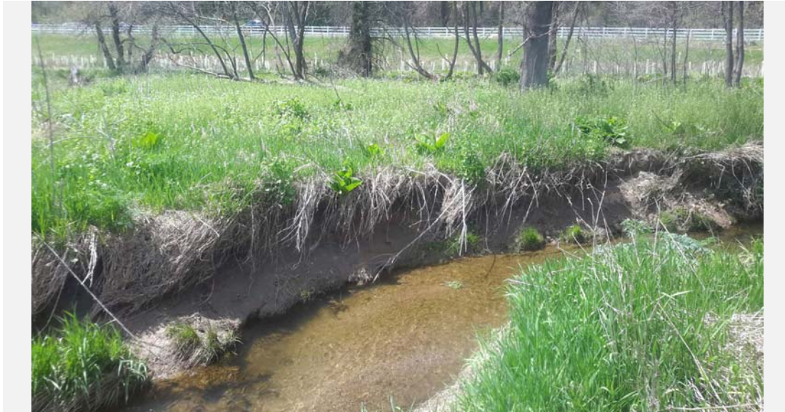
Facing right bank, erosion with poor root depth and stream has poor epifaunal habitat availability.
