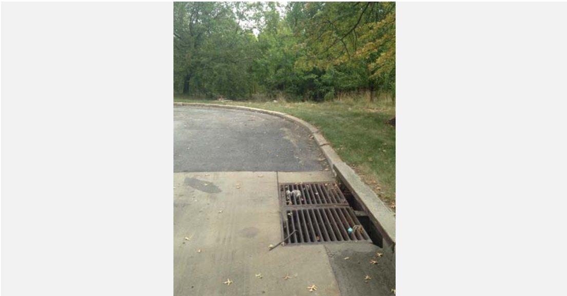
Grate inlet looking into area for proposed extended detention wet pond.
