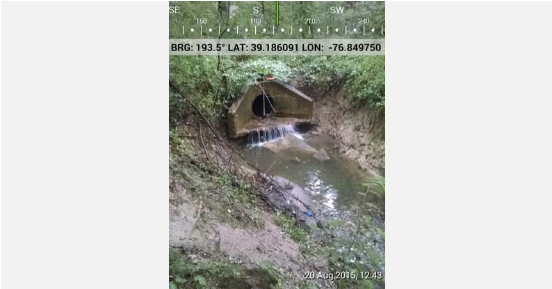
Looking at outfall pipe from top of bank.
