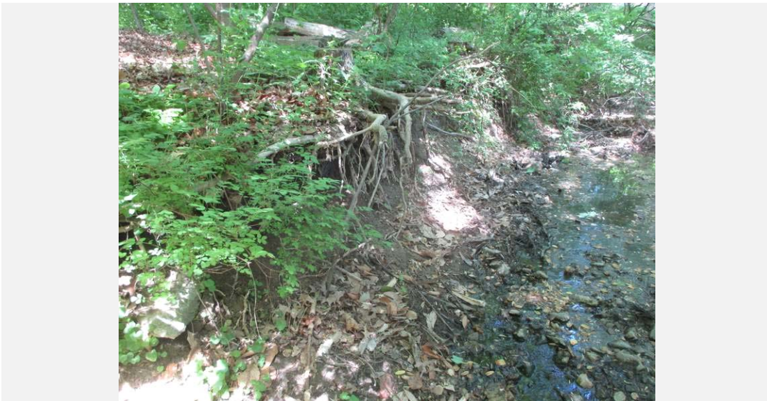
Erosion occurring along the right stream bank. Photo taken just downstream of failing outfall headwall.
