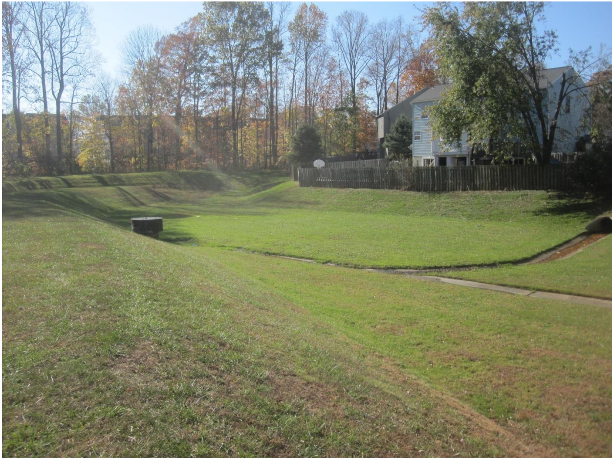
Figure 2. SWM pond at 9518 Jaclyn Court, access via Fens Hollow Court, SMP-BC-D332
