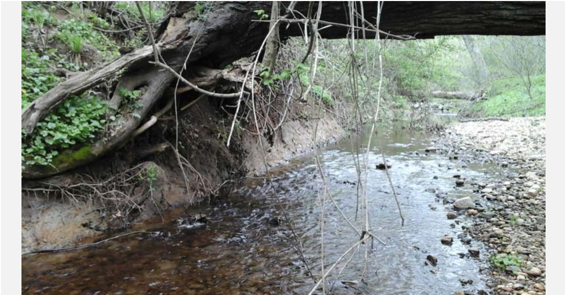
SR-55 facing upstream at severe bank erosion.
