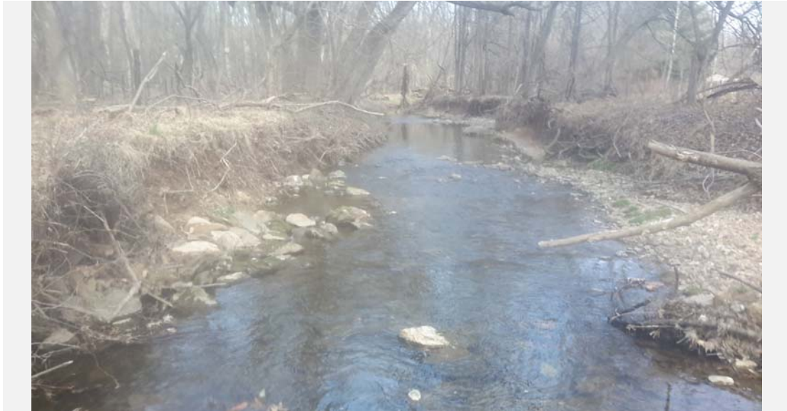
Reach 2 facing downstream, vertical banks with moderate root depth.
