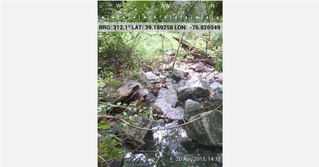
At outfall pipe looking downstream.
