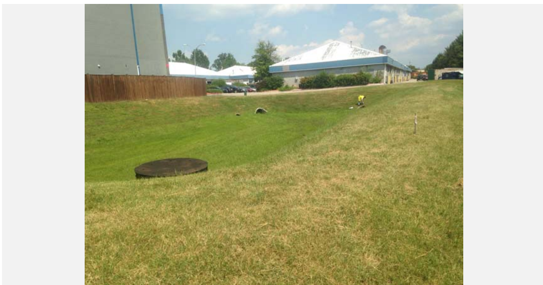
Over principal spillway looking northeast.
