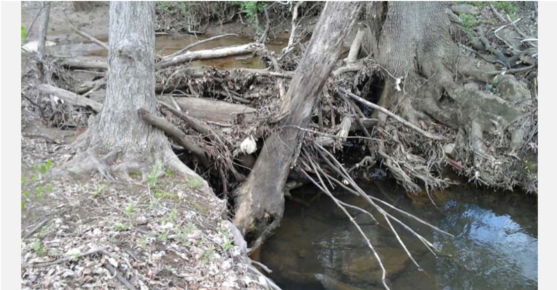
SR-53 facing upstream at a 4 ft. tall headcut.
