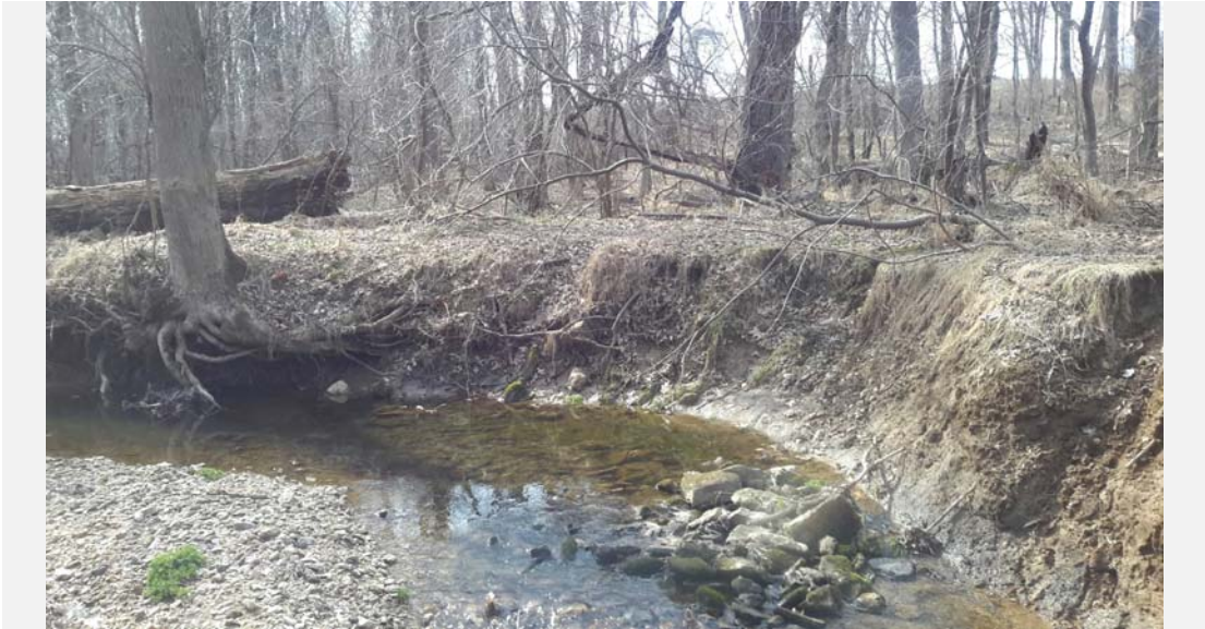
Reach 2, erosion on right bank. Undercut tree and point bar formation.
