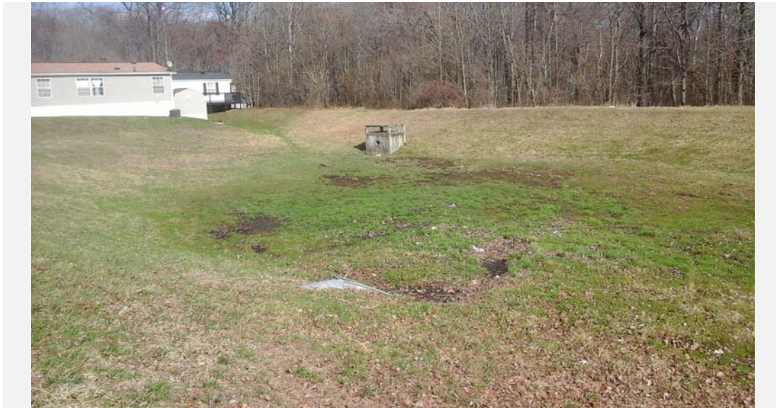
Looking east toward the facility and riser from near Gatewood Drive.
