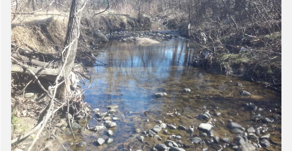
Eroded banks, good riffle material.
