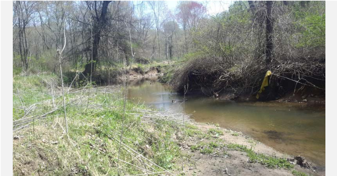
Undercut banks with falling trees and poor root depth.
