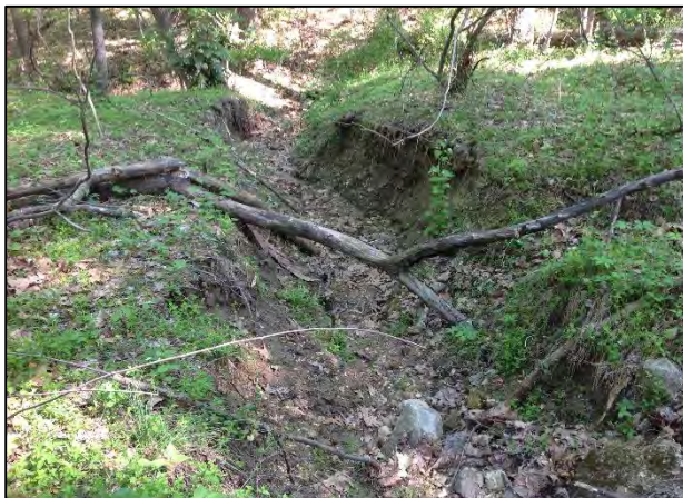
Figure 4-6. Typical degraded outfall channels observed during Outfall Stabilization Assessments
