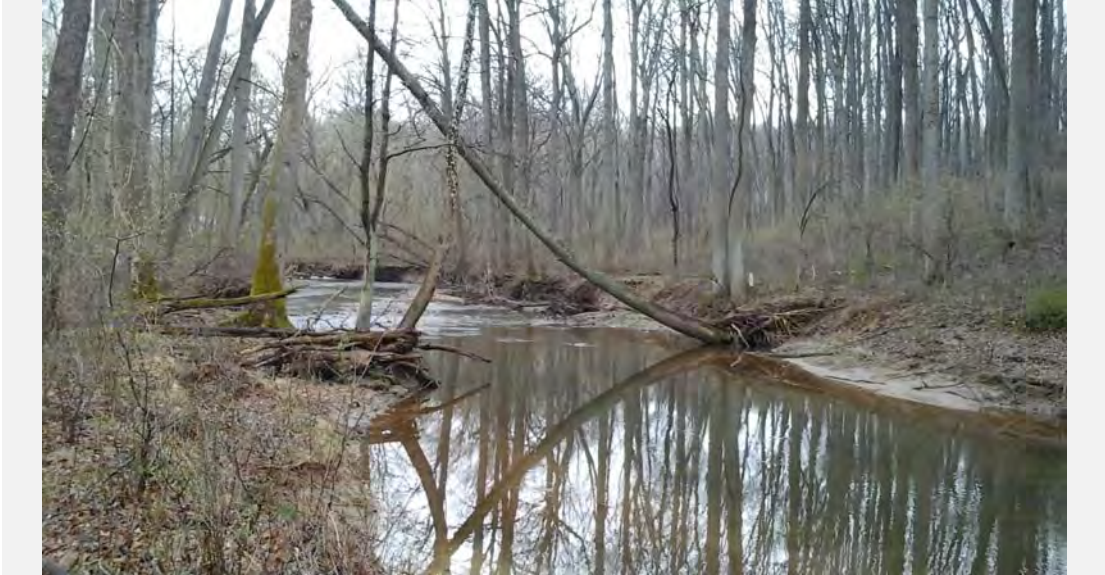
SR-13 facing downstream at severe bank erosion.
