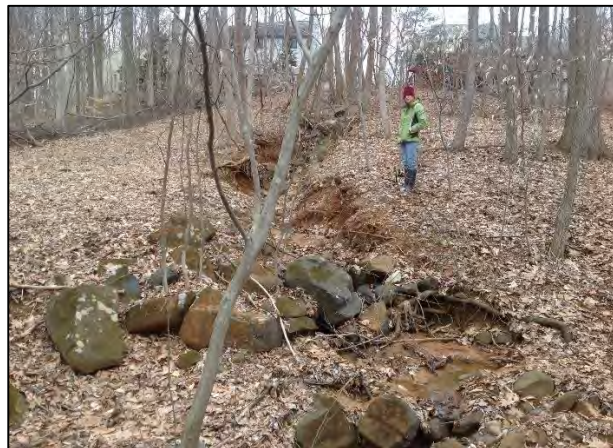
Figure 4-6. Typical degraded outfall channels observed during Outfall Stabilization Assessments
