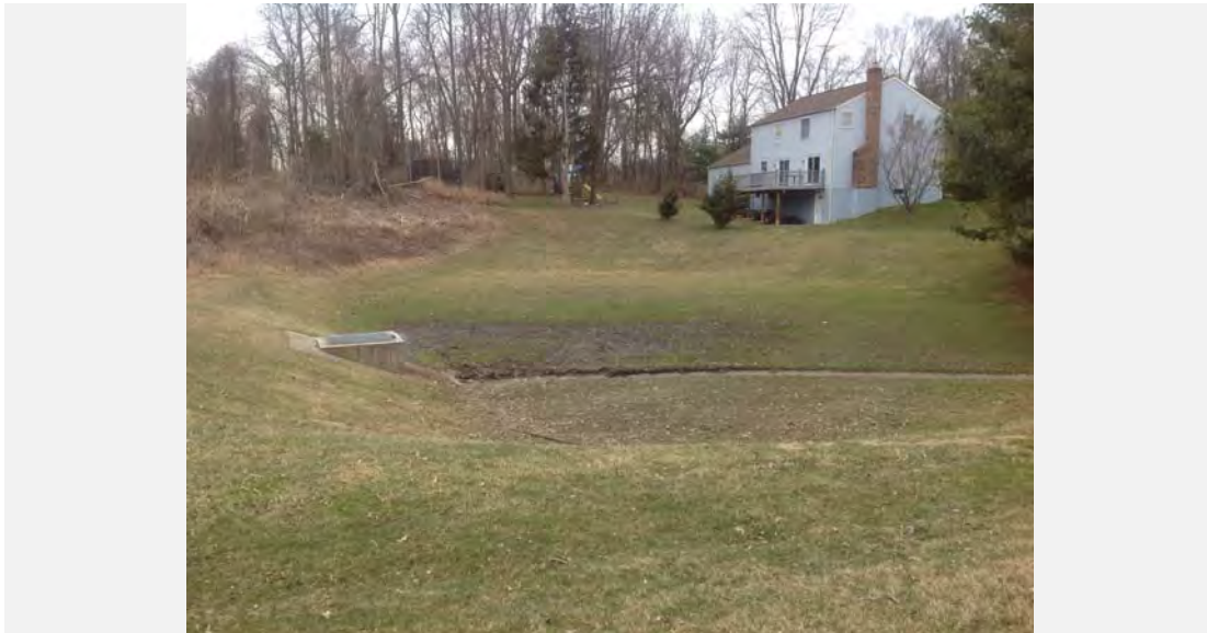
Basin overview looking west.
