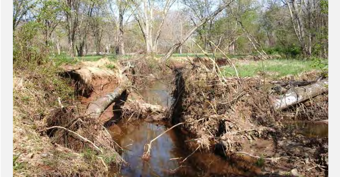
SR-12 facing upstream at severe bank erosion.
