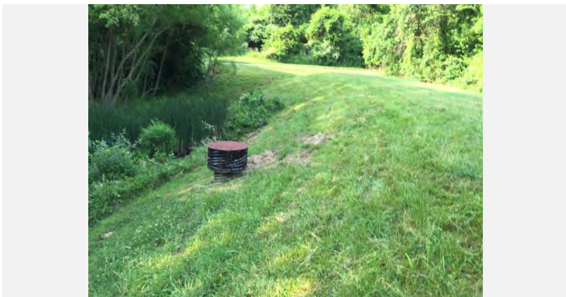
Riser structure looking south.
