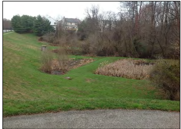
Figure 4-2. Typical Dry Pond (left) and Extended Detention Dry Pond (right) evaluated during BMP Conversion Assessments
