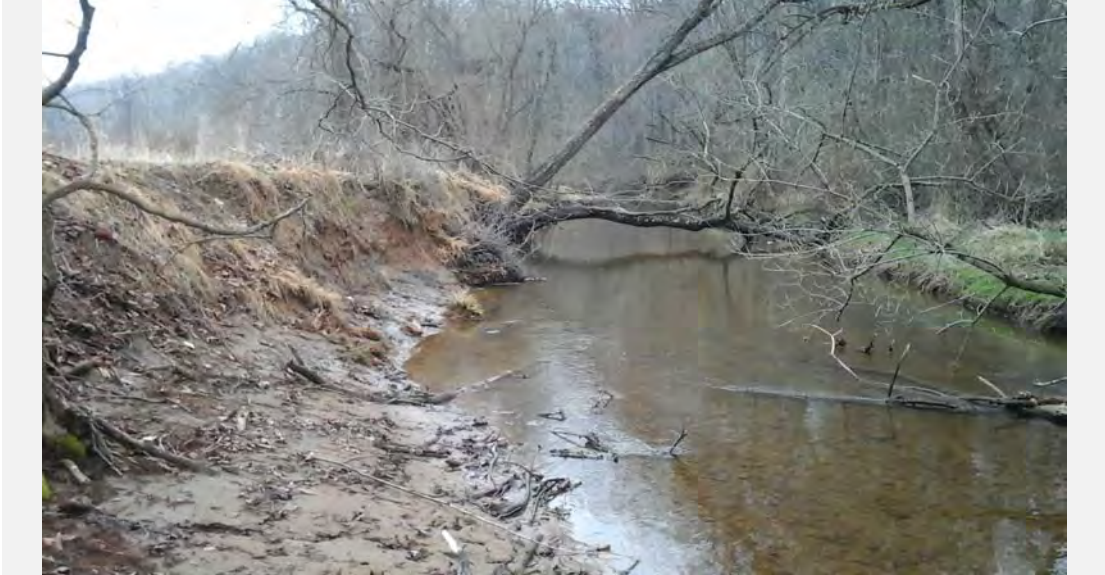
SR-7 facing downstream at severe bank erosion.
