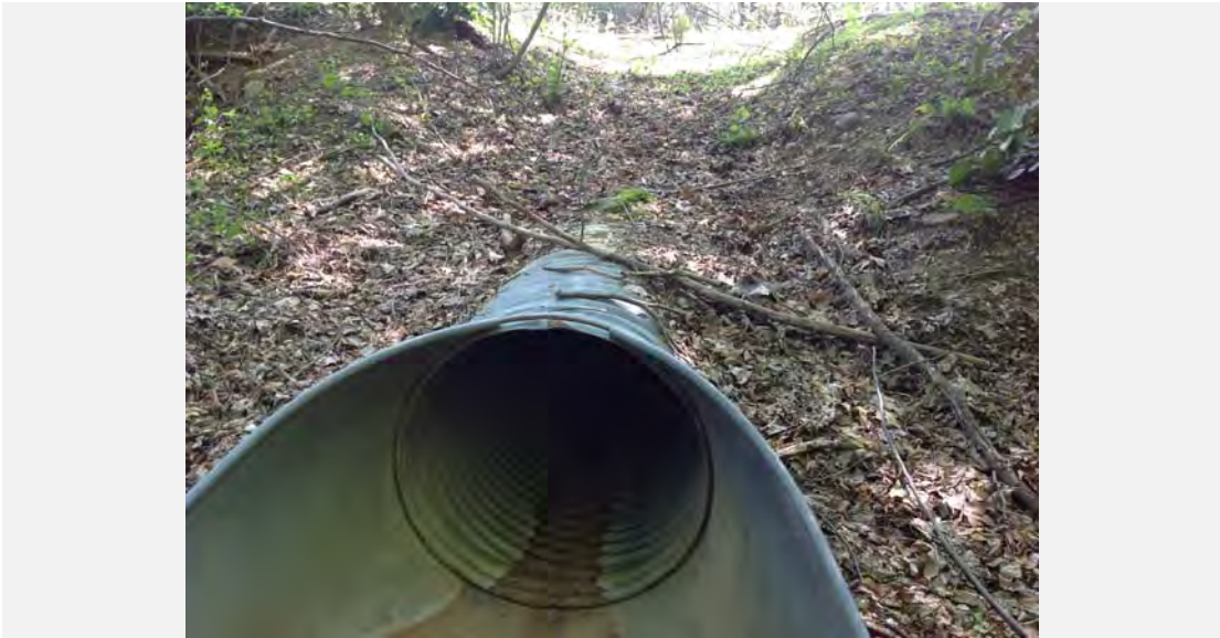
Upstream View of 36 in. CMP.
