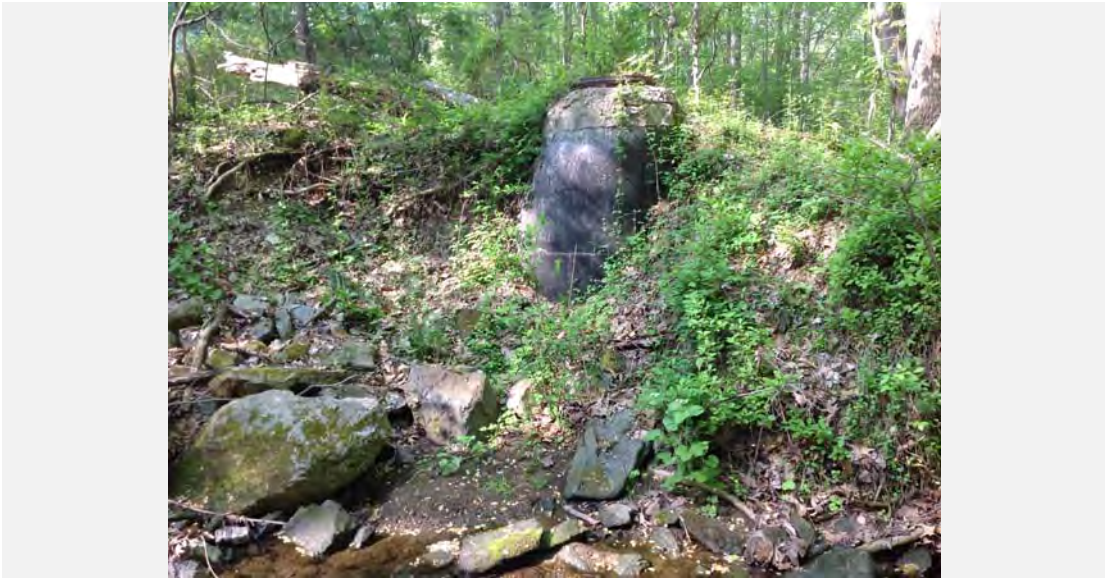
View of outfall channel and exposed sewer manhole.
