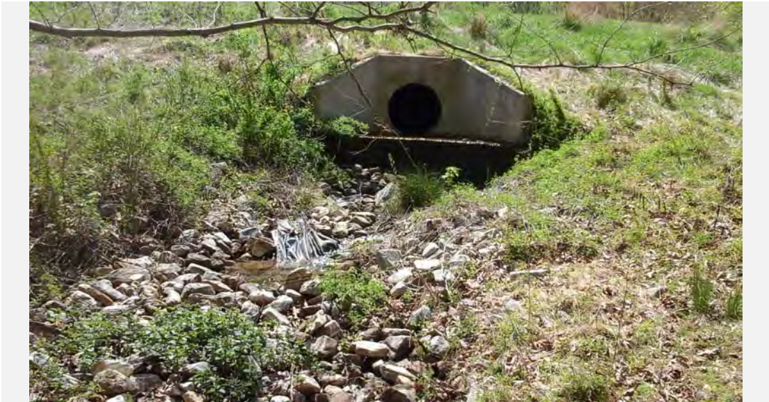
NMP-OF-F102 facing upstream at stormwater pond outfall and pipe outfall channel.
