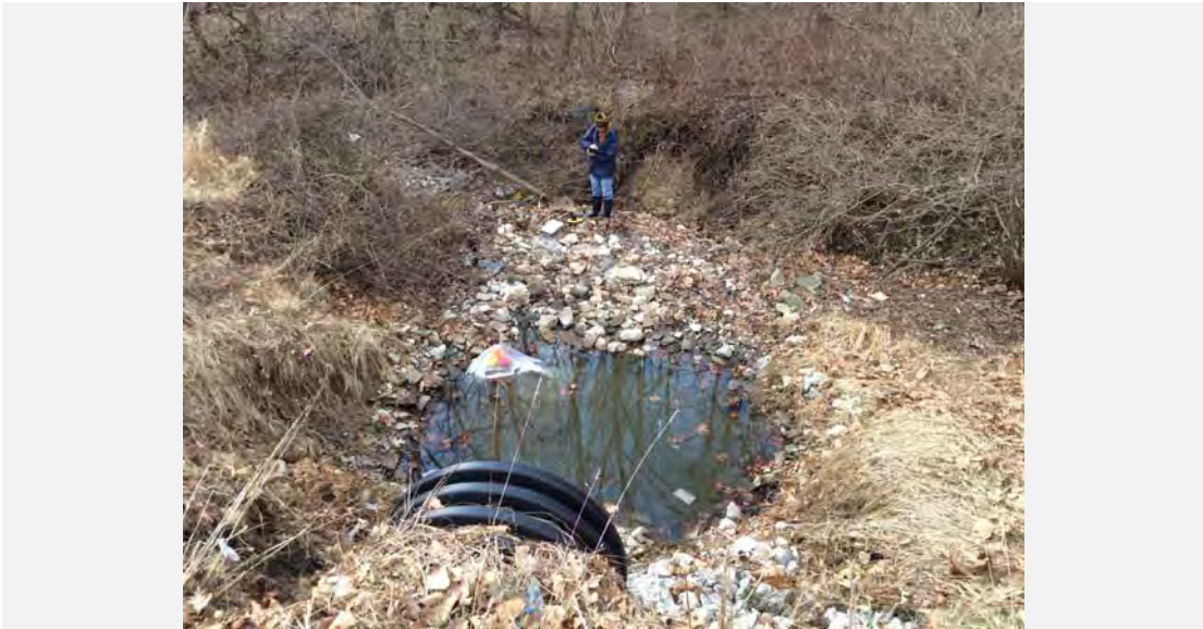
Downstream view of outfall barrel and incised channel.
