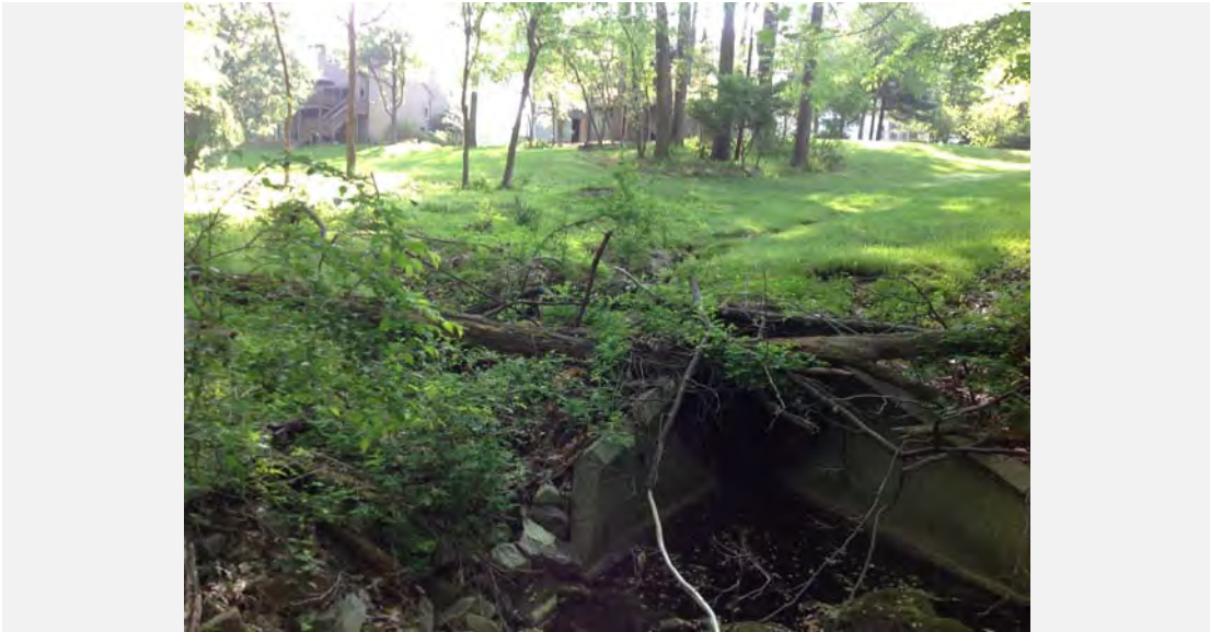
Upstream view of 48 in. outfall and portion of the access.
