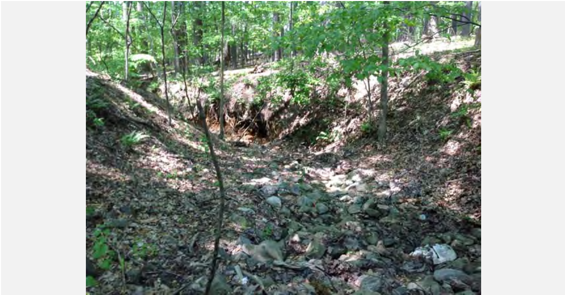
Downstream view of outfall channel.
