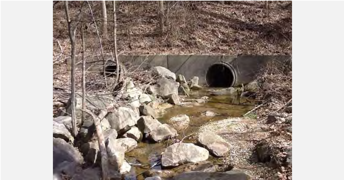
Upstream view of 30 in. and 42 in. culverts at upstream end.
