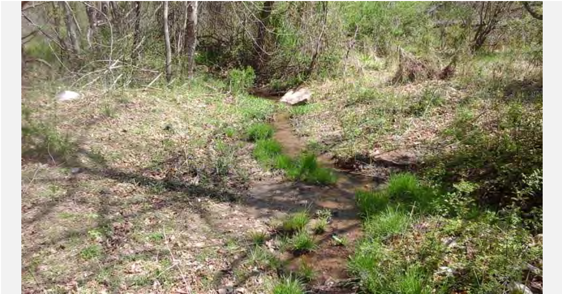
NMP-OF-F102 facing downstream at pipe outfall channel.
