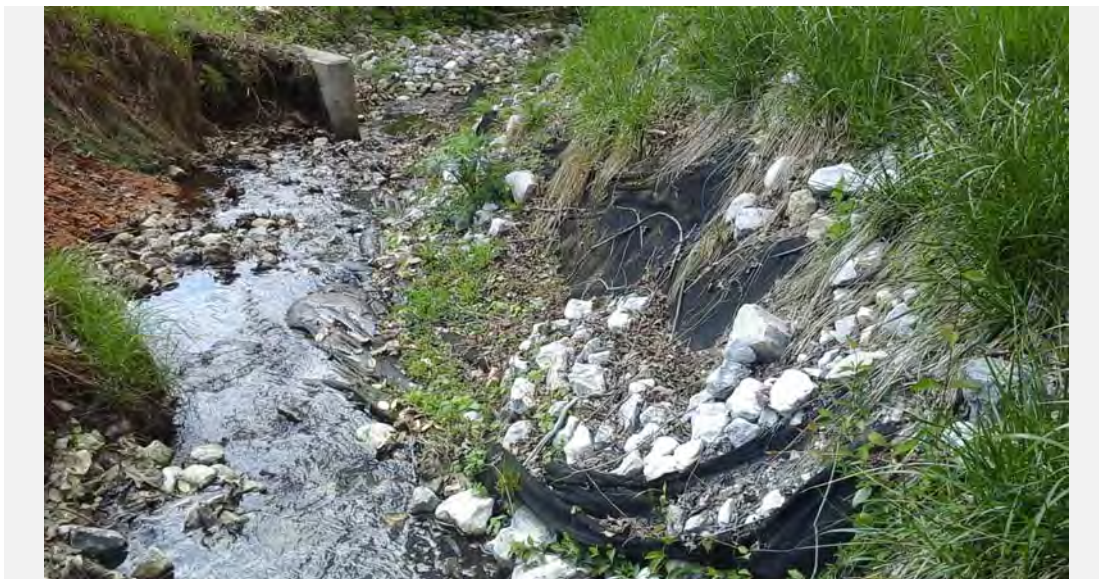
Facing downstream on SMP-SR-F355A where the stream converges with a pipe outfall creating a knickpoint. Recent left bank (looking downstream) erosion is evident where the pipe outlet and geotextile is exposed.
