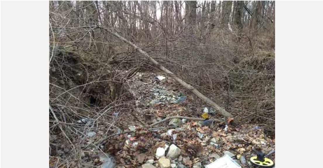
Downstream view from outfall bottom.
