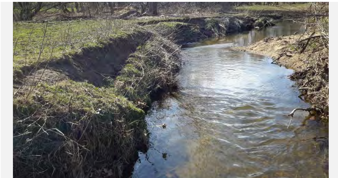
Facing upstream at a recent bank failure. Poor vegetative protection and heavy grazing up to the stream bank is also evident.
