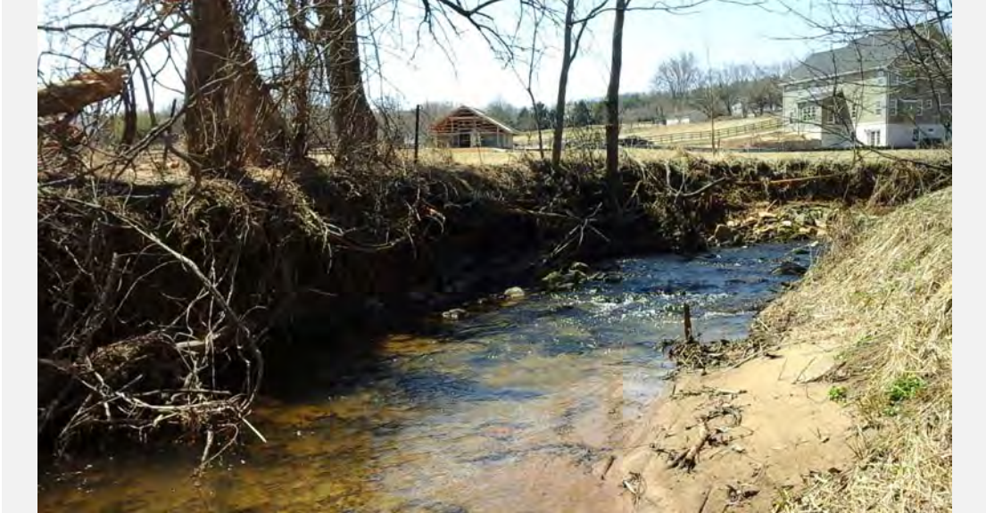
SR-5 facing upstream at moderate bank erosion.
