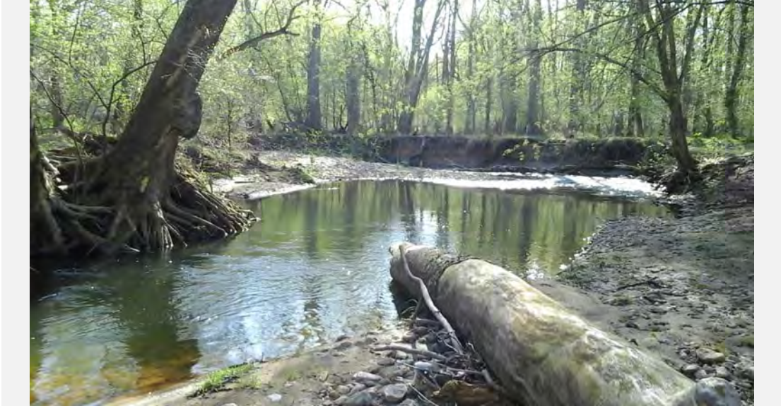
SR-16 facing upstream at severe bank erosion.
