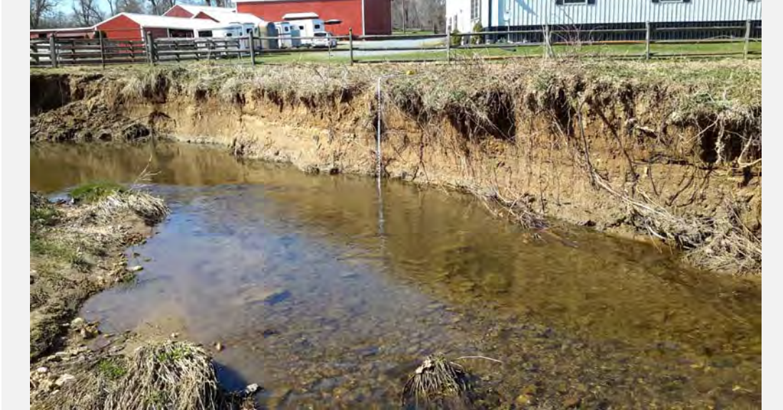
Facing upstream at a tight bend within the existing channel displaying the poor bank protection.
