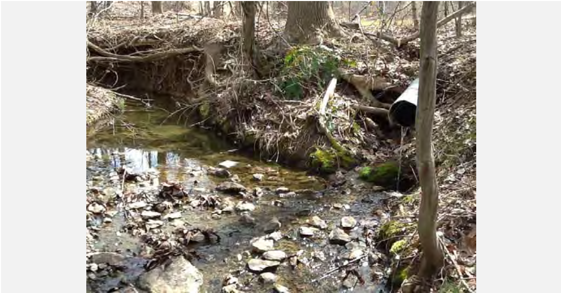
Upstream view of 8 in. outfall.
