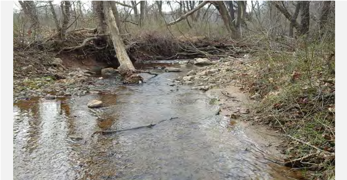
SR-11 facing downstream at moderate bank erosion.
