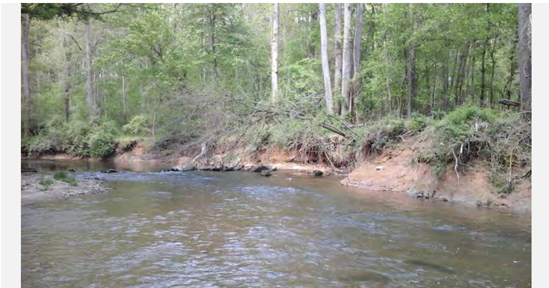
Facing upstream along the downstream mainstem (SMP-SR-F353A) showing patchy bank erosion due to loss of vegetative bank protection.
