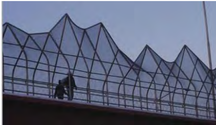
Photo 17: Special Framing Shapes Using Chain Link Fabric to Mimic Mountains on a Bridge in Denver
