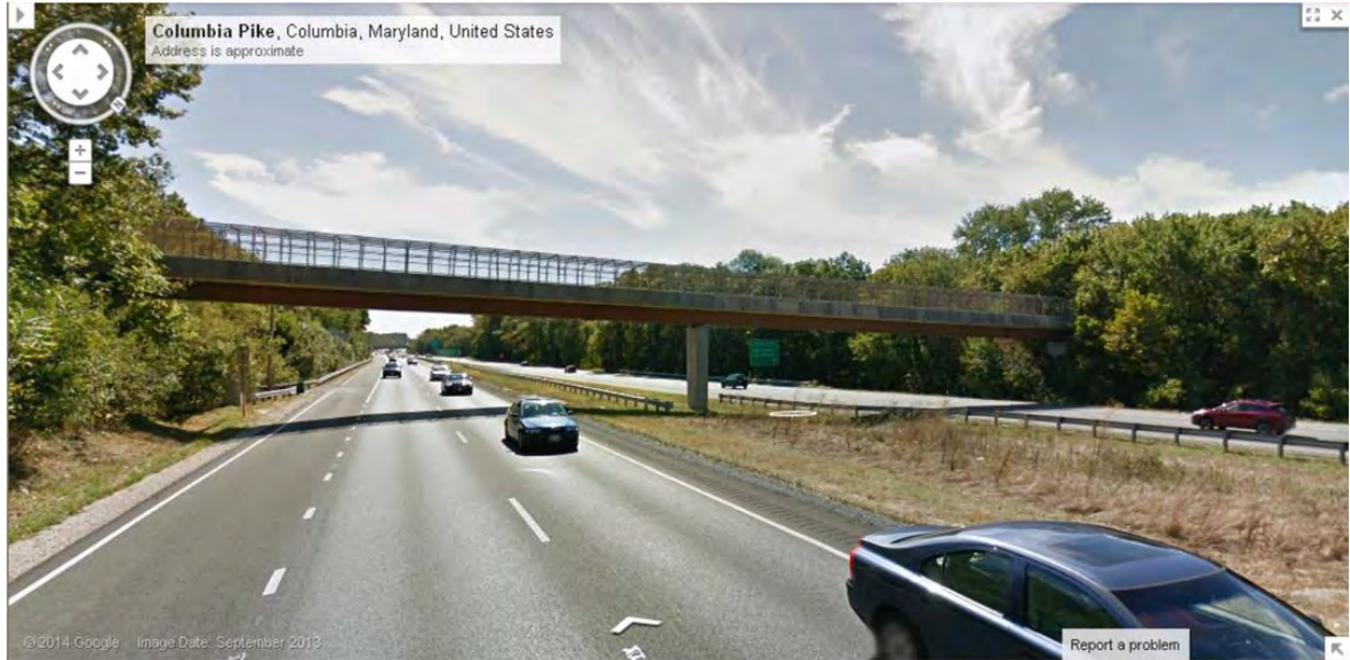
Photo 1: Existing Pedestrian/Bicycle Bridge, Looking South
