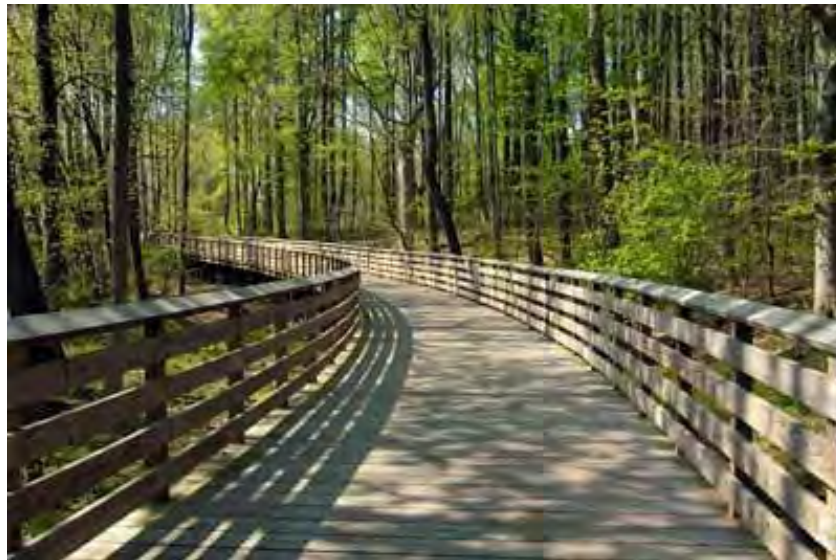
Photo 27: Boardwalk in Montgomery County on Matthew Henson Trail
