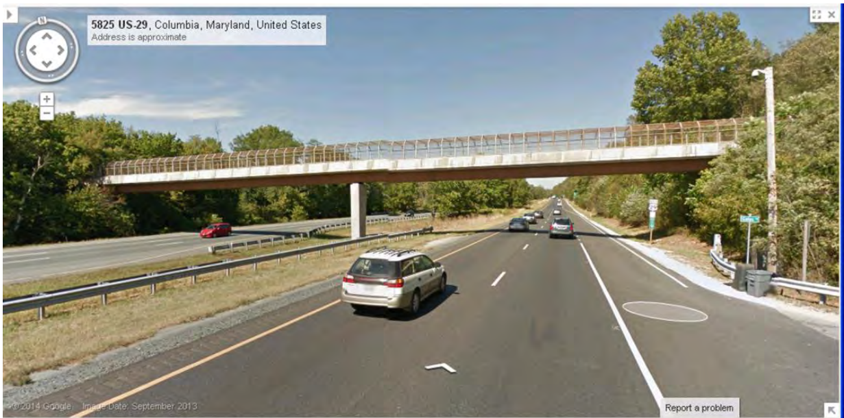
Photo 2: Existing Pedestrian/Bicycle Bridge, Looking North
