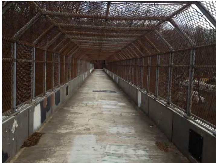
Photo 13: Existing Bridge Barrier
