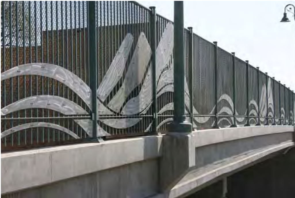
Photo 18: A Bridge in California Featuring Artwork Bolted to the Barrier
