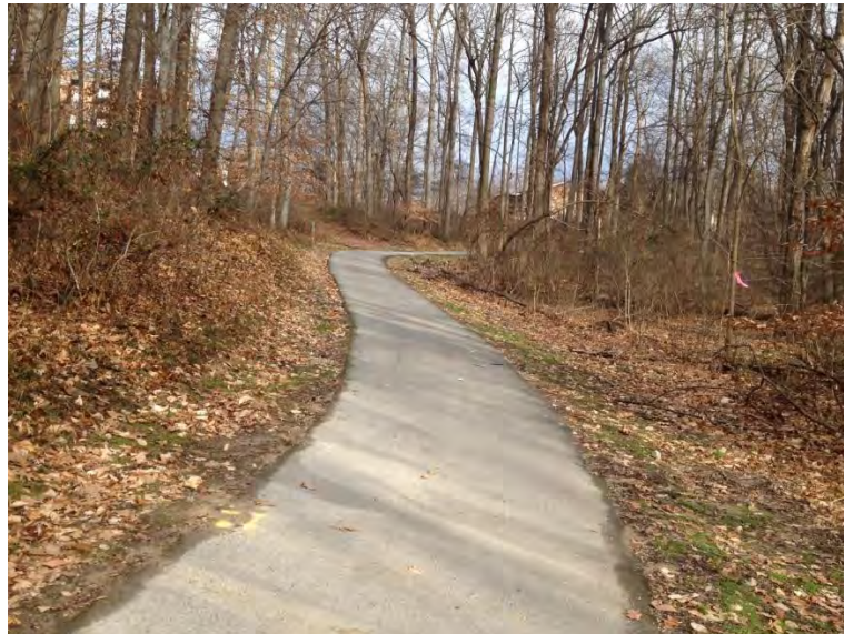
Photo 4: East Side Trail Steepens and Has Significant Cross-Slope (Facing East)
