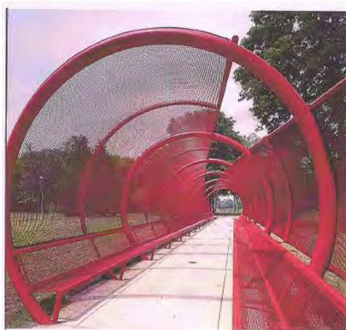
Photo 15: Example of a Steel Tube Enclosure (Source: Dorton Design)
