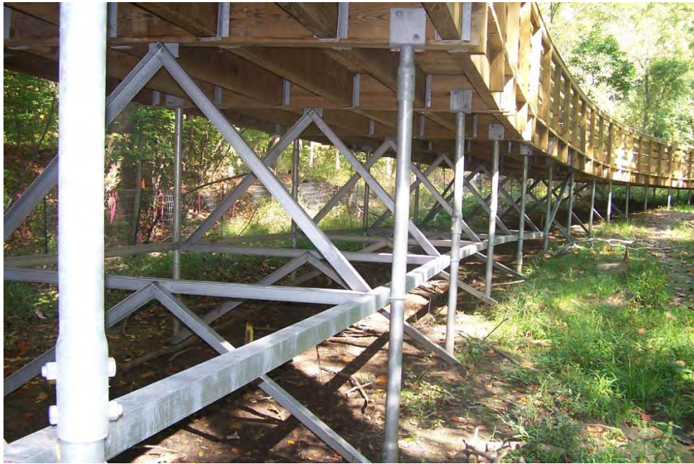
Photo 28: Boardwalk Using Helical Piles
