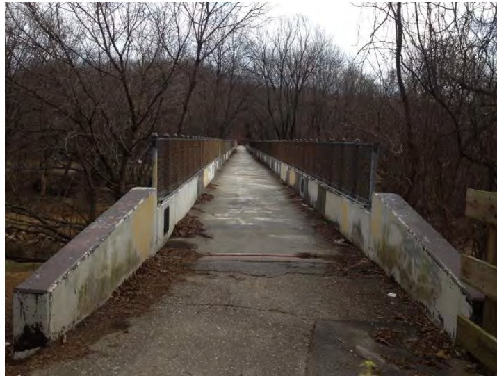
Photo 8: West Side Trail Looking East Across Bridge
