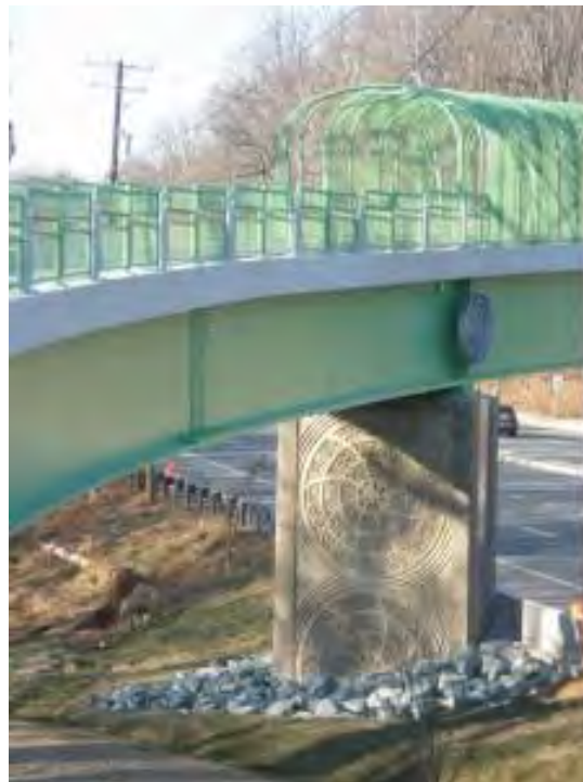
Photo 21: The Rock Creek Trail Bridge Utilizing an Artist's Design for Barrier and Railing (Designed by URS Corporation)
