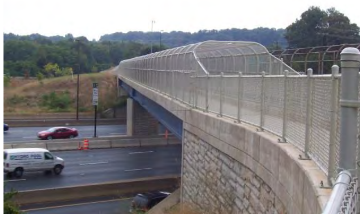
Photo 16: A Traditional Barrier Approved by SHA (I-270 at MD 28 Bike & Ped Crossing in Rockville, MD; designed by URS Corporation)
