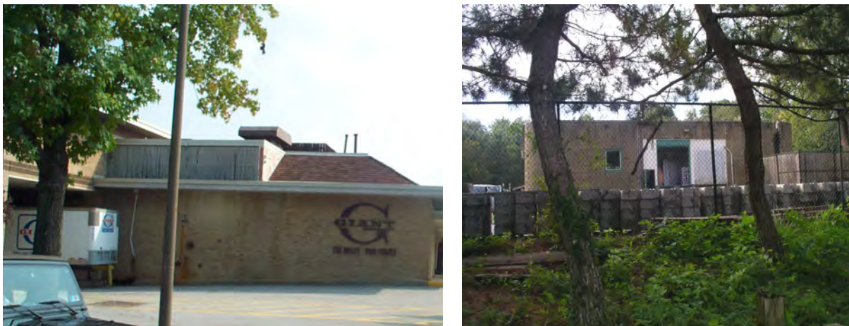
Figure 3.14 Poor loading/unloading practices were found at Giant Supermarket in Wilde Lake, while unlabeled storage drums without secondary containment were found at Centennial Lake Park (right).
