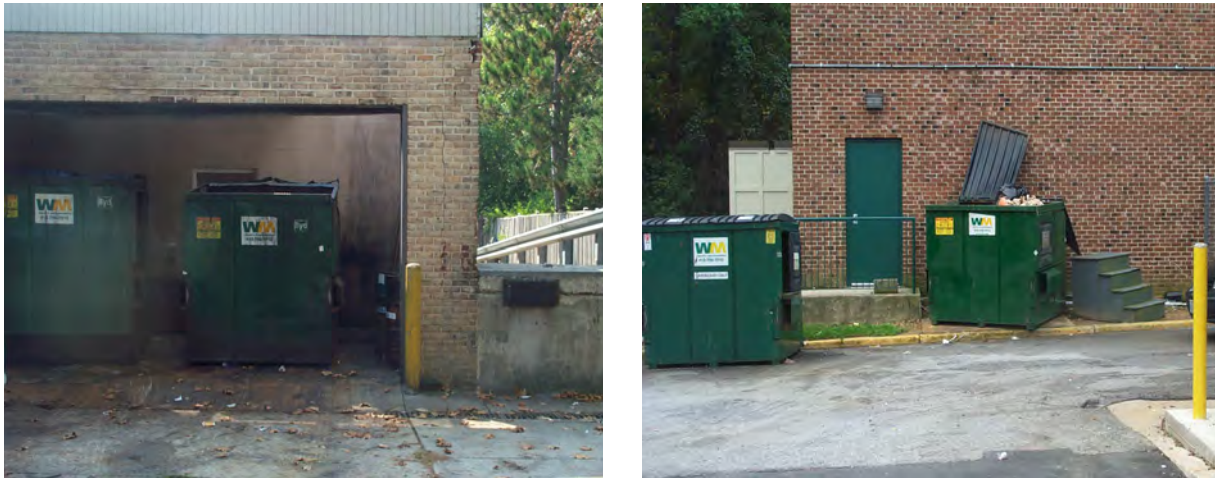
Figure 3.13 Dumpsters throughout both watershed were frequently located on concrete or asphalt and had no secondary containment present.
