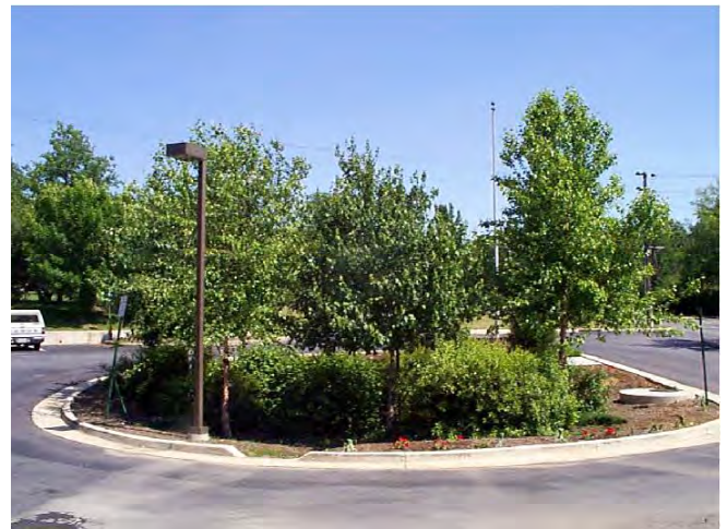
Figure 4.20 Examples of bioretention in parking lots with curb cuts and mixtures of tree and shrub plantings.
