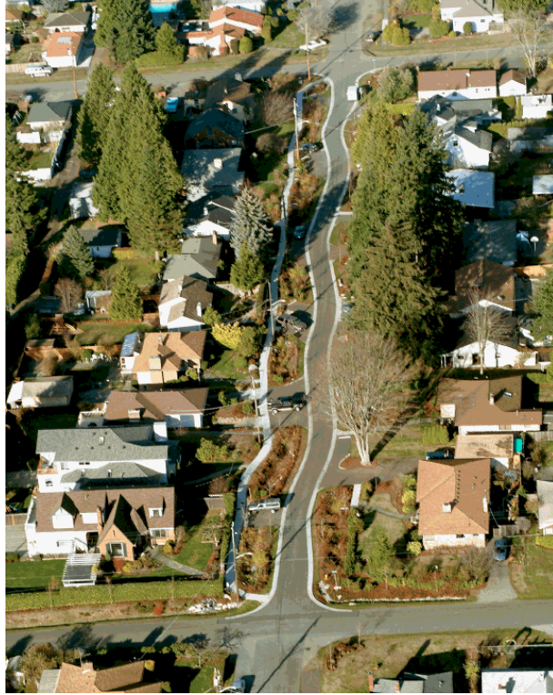
Figure 4.44 SeaStreets aerial photo postconstruction.
