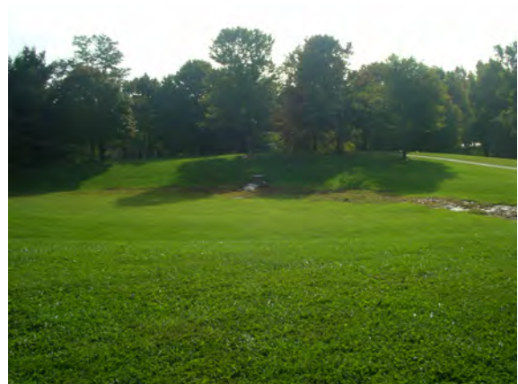
Figure 4.48 View of riser from opposite embankment.
