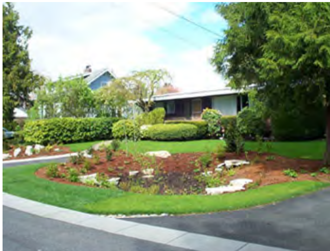
Figure 4.42 Example streetscape stormwater filtration (Seattle, WA).
