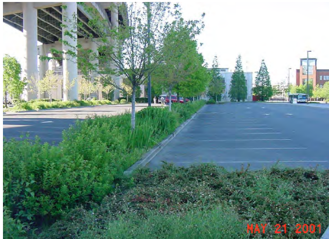
Figure 4.20 Examples of bioretention in parking lots with curb cuts and mixtures of tree and shrub plantings.
