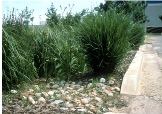
Figure 4.22 Typical inlet with rock-lined entrance to provide energy dissipation and pretreatment.
