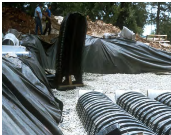
Figure 4.49 Typical perforated plastic half pipe used for recharge.
