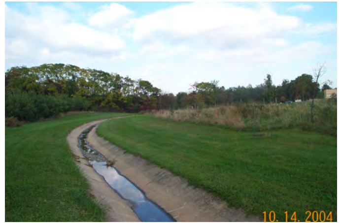
Figure 4.14 Existing concrete channel looking down channel.
