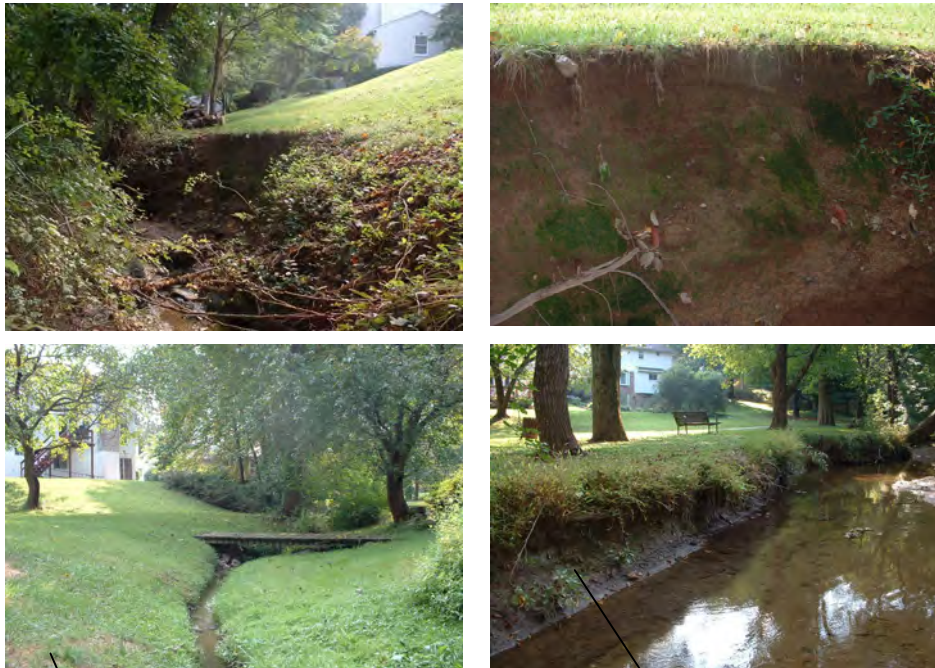
Figure 4.51 Typical inadequate buffer and streambank repair areas.
