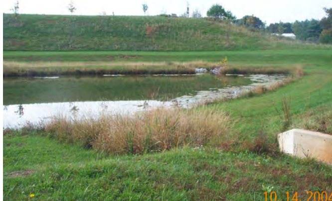
Figure 4.12 Stormwater pond at the Homewood School.
