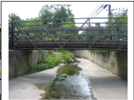
Point # 1038 Location: -76.810154 39.268894 Description: Road crossing. Foot bridge to historical school building.
