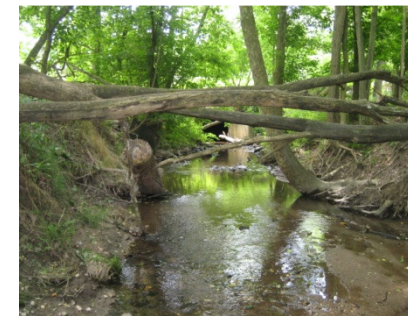
Point # 115 Location -76.840667 39.278438 Description: Potential debris blockage.
