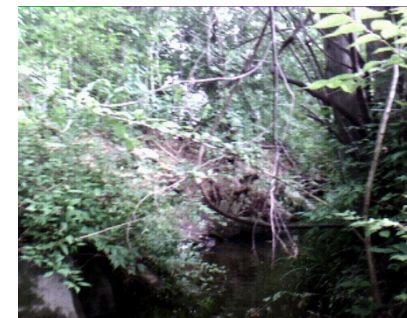
Point # 104 Location -76.840632 39.279754 Description: Bank height transition point. 4-6 ft banks to 8 ft banks.
