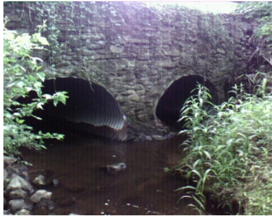
Point # 101 Location: -76.840812 39.279565 Description: Road crossing. Stacked stone headwall, ~8 feet above culvert inlet.
