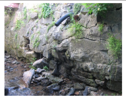
Point # 1012 Location: -76.799508 39.268230 Description: Failing rock wall.
