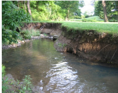
Point # 1063 Location: -76.820501 39.272305 Description: Erosion site. Mowed lawn up to top of bank.
