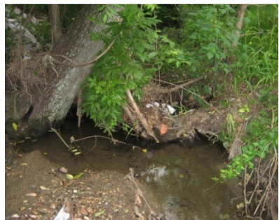
Point # 1077 Location: -76.821750 39.271887 Description: Debris blockage. Leaning tree and root ball blocking channel.
