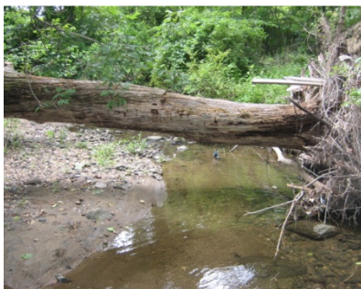
Point # 1047 Location: -76.814724 39.270583 Description: Debris blockage. Tree across channel. Tree is ~24" DBH and ~ 2' above water surface.
