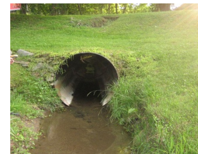
Point # 1072 Location: -76.820626 39.272273 Description: Road crossing. Pipe culvert.
