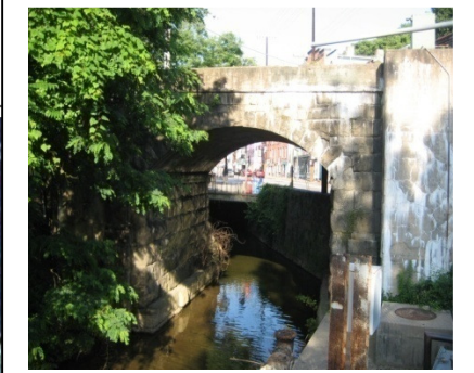
Point # 1001 Location: -76.794685 39.267801 Description: Rail road crossing. Bridge; beginning of study area.
