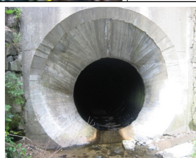
Point # 1032 Location: -76.807700 39.268890 Description: Road crossing. Pipe culvert near West End.
