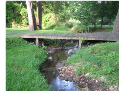
Point # 1071 Location: -76.820460 39.272208 Description: Road crossing. Foot bridge on small tributary.
