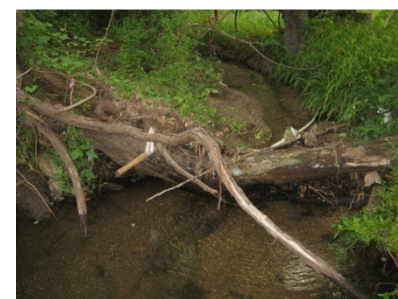
Point # 1076 Location: -76.821417 39.272015 Description: Debris blockage. Tree across channel, backing up sediment.
