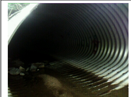
Point # 1016 Location: -76.800255 39.268813 Description: Downstream end of large culvert.
