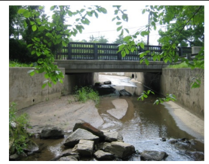
Point # 1037 Location: -76.809738 39.268635 Description: Road crossing. Bridge, 18.5'W x 5'H
