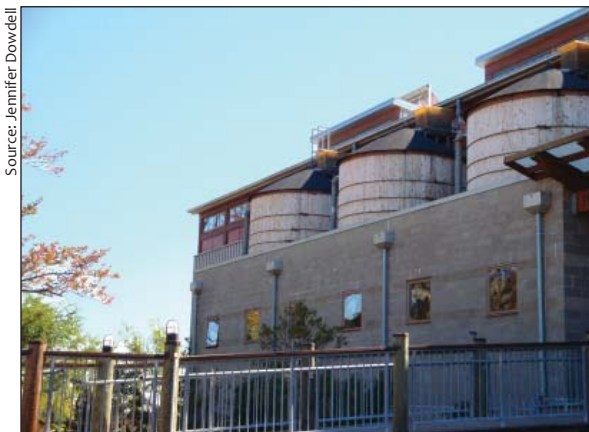
Cisterns at the Chesapeake Bay Foundation collect rainwater for nonpotable indoor uses.
