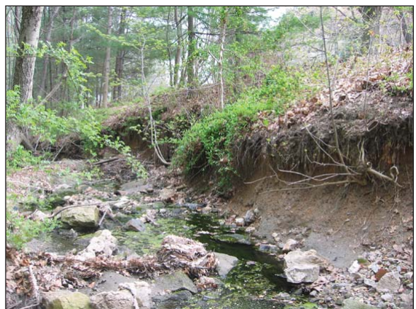
Increased stormwater runoff can increase stream channel erosion, degrading stream water quality and habitat.
