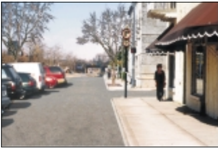
This simulation shows how Lower Elkridge might appear if redeveloped as a Corridor Activity Center.
