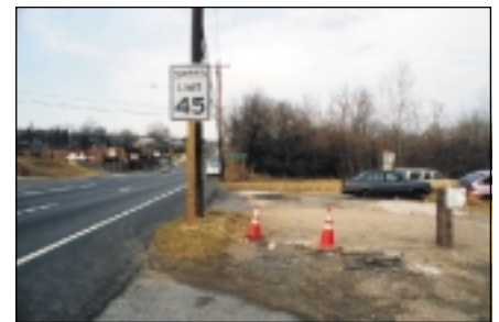
Undefined existing roadway edge that lacks amenities.
