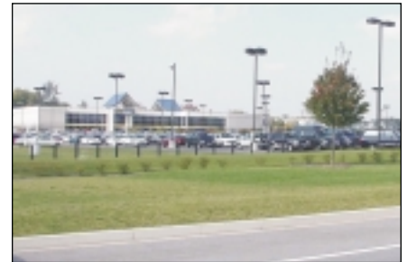
Single story uses are prevalent in the corridor's business parks.
