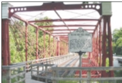
The color and historical industrial design character of the Bollman Bridge is the inspiration for street furniture along Route 1.
