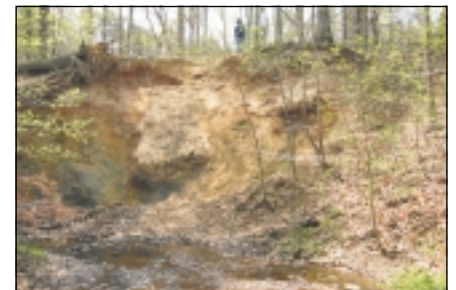
Watershed studies can target severely eroded streams for stabilization and restoration.
