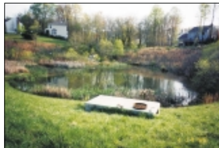
SWM facilities help reduce flooding and improve storm drainage.
