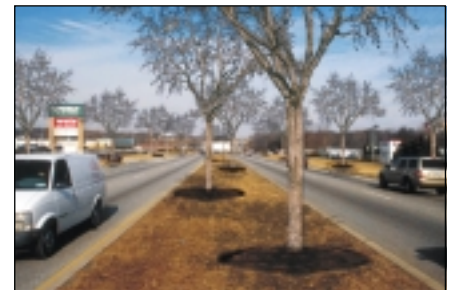
Desirable median and defined roadway edge with plantings.
