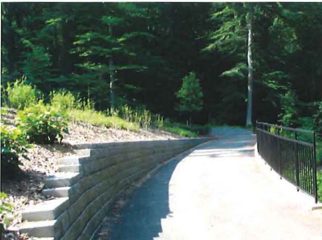
Segmented Concrete Retaining Wall Source: TDG Library
