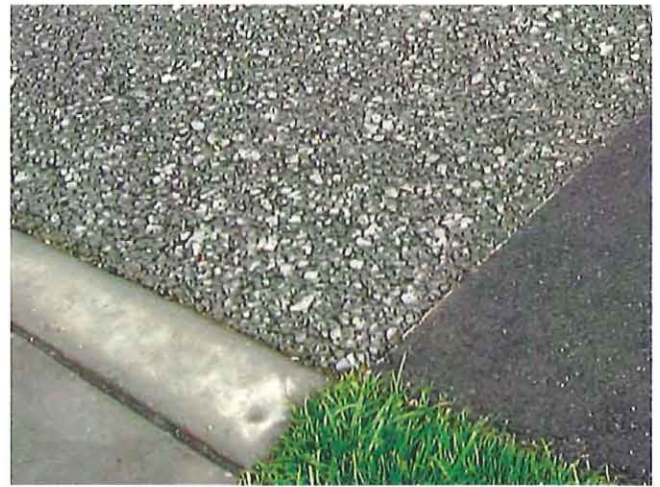
Permeable Concrete Source: Concrete Network
