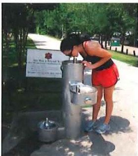
Drinking Fountain Source: TDG Library
