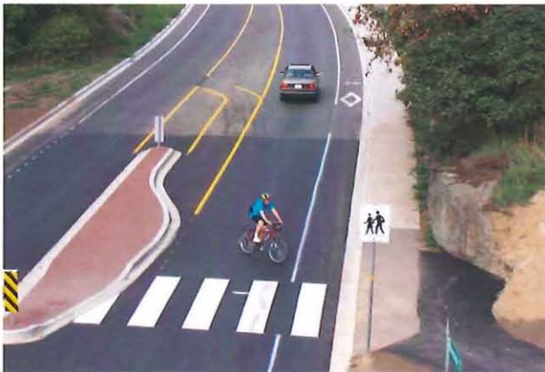
Intersection Crossing Source: TDG Library
