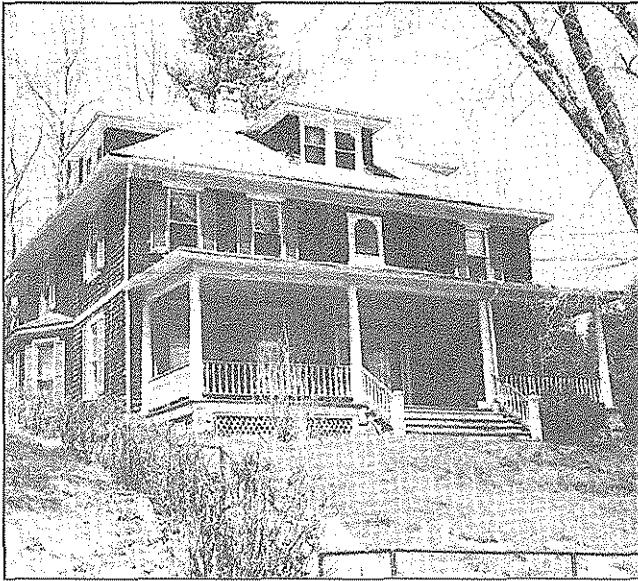
This porch displays Classical Revival influence in its columns and turned balusters.
