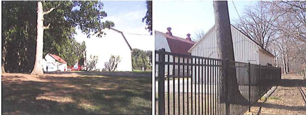
Barn structures along north edge of Merriweather.
