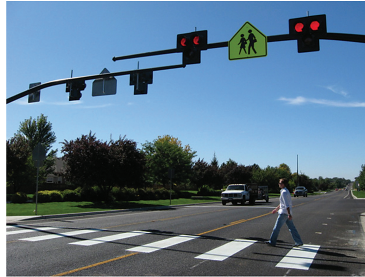
A pedestrian activated beacon could be installed along Route 108 east of Great Star Drive.
