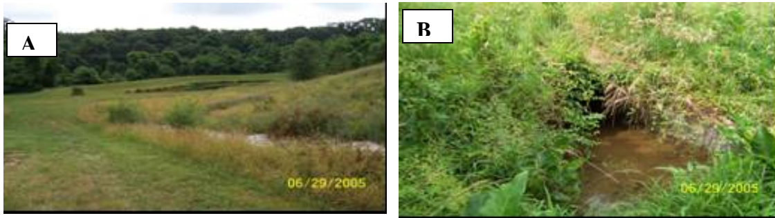
A) Overview of extended detention dry pond. B) View of outfall.
