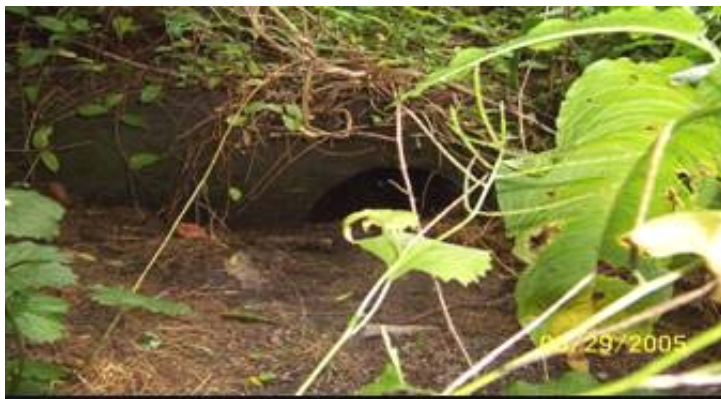
View of culvert and sediment.
