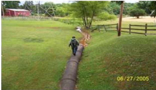
View of piped stream with no buffer zone.
