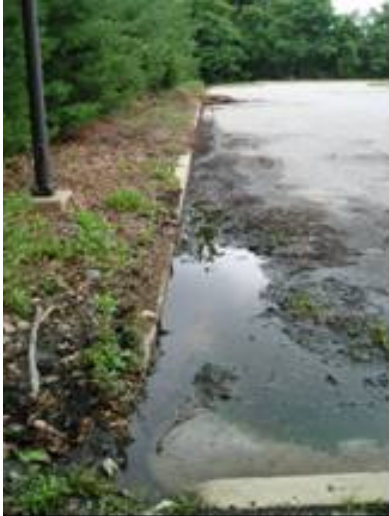
View of curb on Elkridge Elementary School Parking lot.
