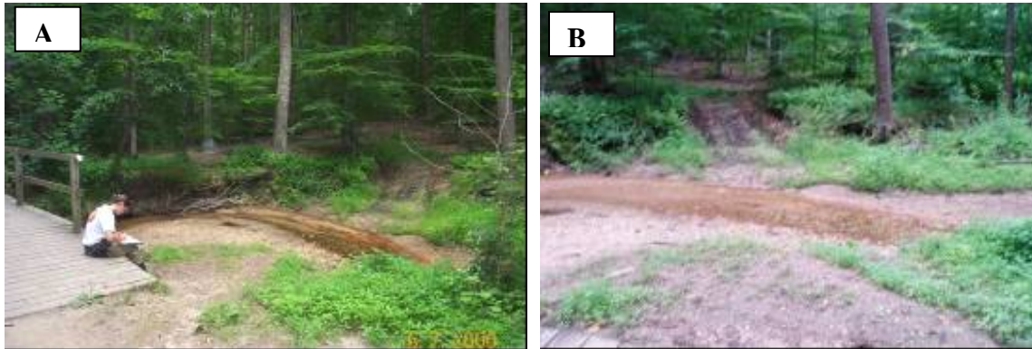
A) Bridge and trail crossing B) Close-up of trail crossing.
