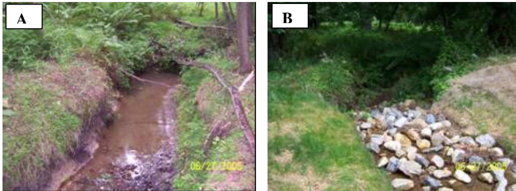
A) View of downcutting. B) View of sewer crossing.
