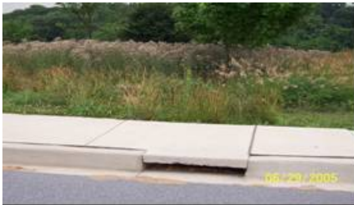
View of parking lot runoff drain and grassy area.
