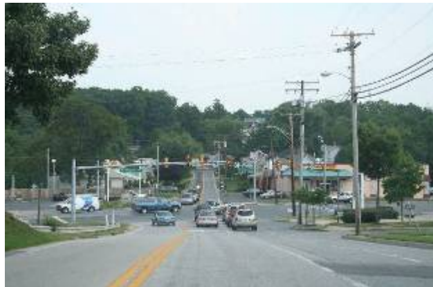
Collectors and arterials, like Montgomery Road, can be improved with pedestrian and bicycle accommodation to increase connectivity and safety for all travelers.
