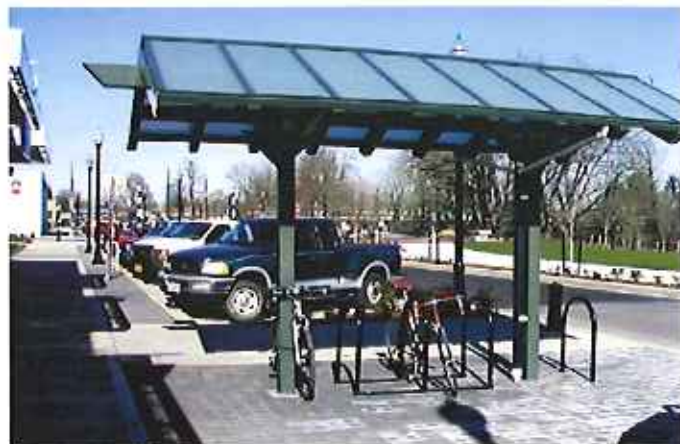
Covered Shelter Bicycle Parking
