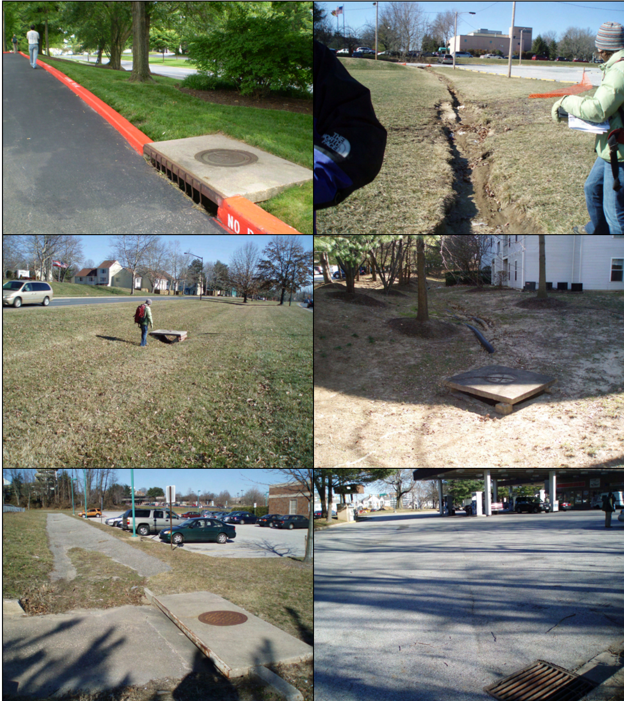
Figure 2-1: Retrofit opportunities include: creating a bioretention practice along the perimeter of a parking lot (top left); converting an eroding drainage channel into a bioswale (top right); installing a bioswale in a road median (middle left); installing a bioretention practice to treat rooftop runoff (middle right); converting a paved drainage channel into a bioswale (bottom left); and installing perimeter sand filter to treat runoff from a gas station (bottom right).
