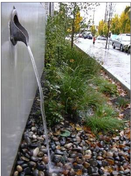
Rooftop Stormwater Treatment
