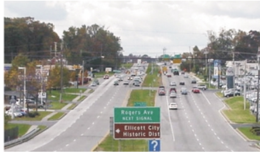
Figure 26: Typical Route 40 suburban boulevard section.
