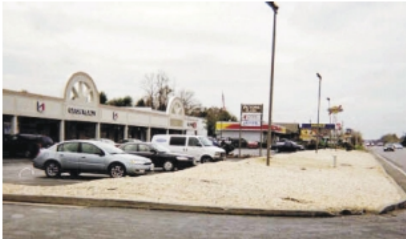
Figure 23: Sidewalks and landscaping are missing in parts of the corridor.
