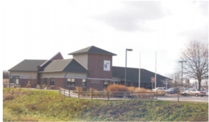
Figure 21: Improving pedestrian and transit connections to the Ellicott City Senior Center and Miller Library is an important corridor transportation goal.
