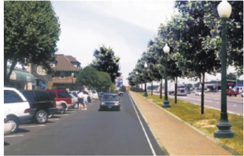
Figure 28: Parallel service roads are a typical feature of super boulevard road sections.
