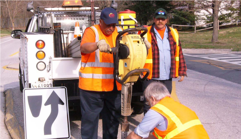
Bureau of Highways employees insert a post in a median strip on a county road in preparation to install the directional traffic sign on the left in the photo.
