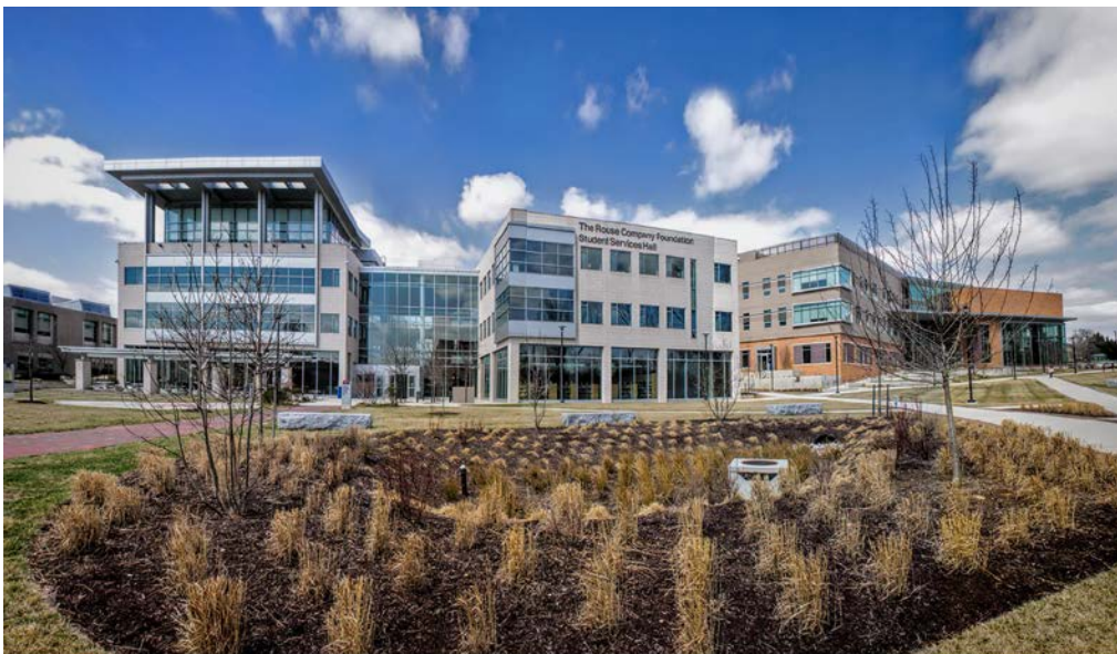
This rain garden at Howard Community College collects and filters stormwater preventing runoff and thereby helping to improve the health of Chesapeake Bay.
