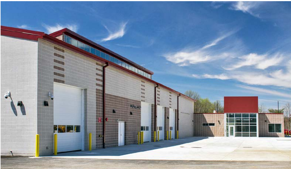
Regional Transportation Agency of Central Maryland (RTA) buses and transit vehicles will be serviced and maintained at this new facility in Annapolis Junction.
