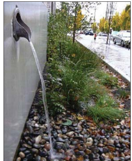
Small treatment facilities, such as this stormwater planter, will become more prevalent with Environmental Site Design.
