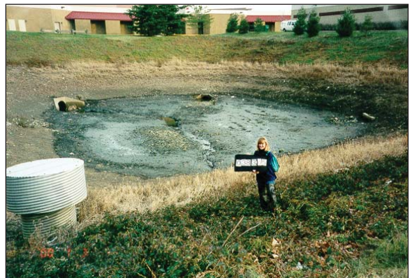
Environmental Site Design uses small treatment facilities, such as rain gardens (above), rather than large ponds (below).
