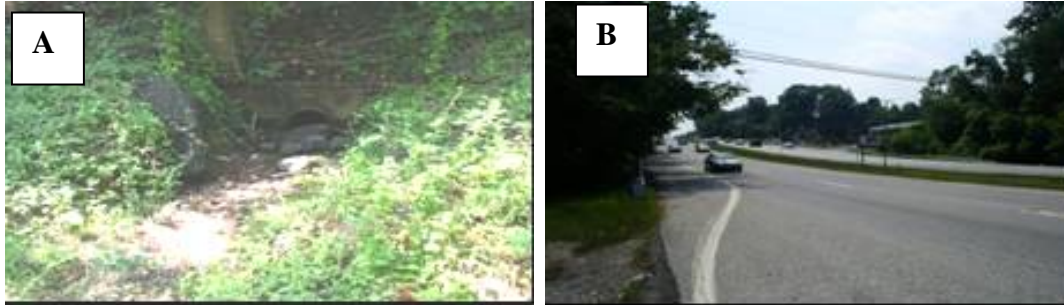
A) View of storm drain outfall. B) View of Route 40, where inlet is located.
