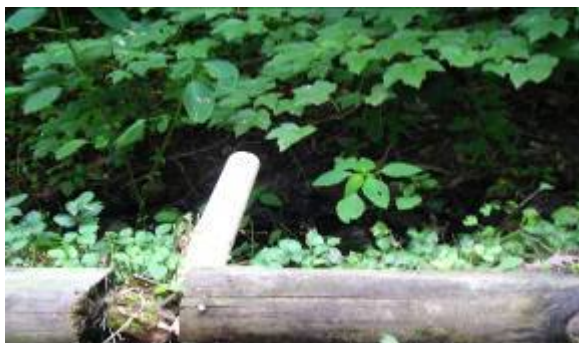
View of residential swimming pool outlet.
