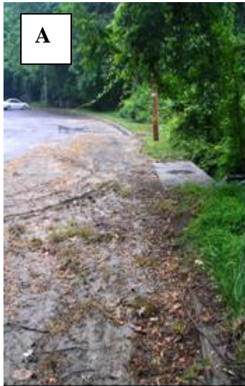
A) View of clogged drain inlet. B) View of road leading to clogged inlet.
