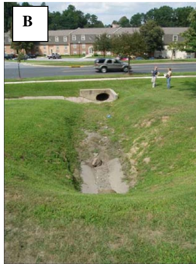
A) View of broken channel. B) Different view of same broken channel and erosion.
