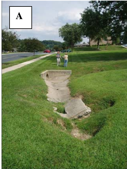
A) View of broken channel. B) Different view of same broken channel and erosion.
