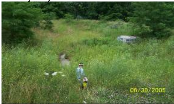
View of concrete low flow channel in stormwater pond.
