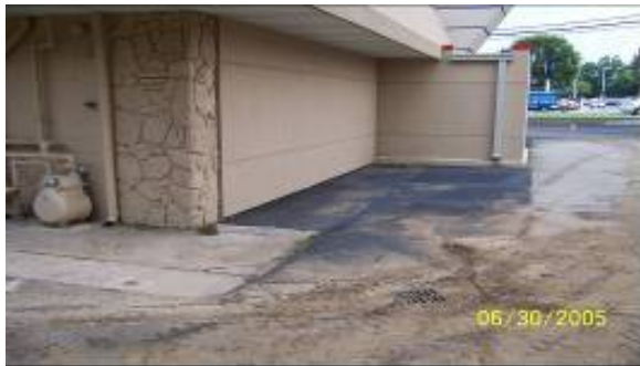
View of newly constructed building, with new storm drain.
