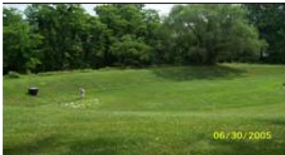
Overview of stormwater pond.
