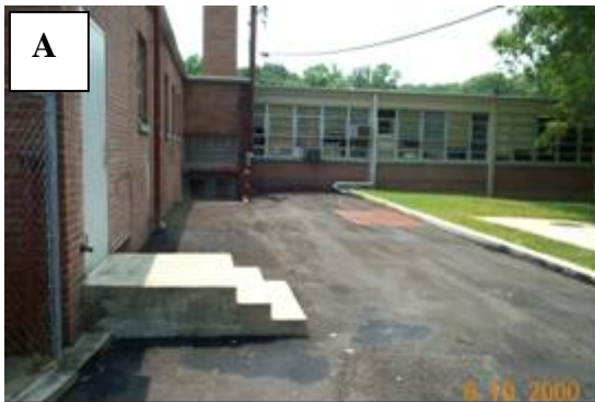
A) View of roof discharging to pavement, B) View of driveway with erosion along edge of paving
