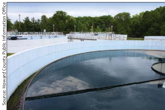
The Little Patuxent Water Reclamation Plant treats wastewater for about 70% of the County served by public sewer.
