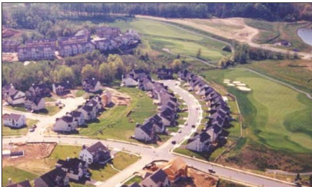
Impervious cover in the County is projected to increase from 13% in 2007 to 15% in 2030.
