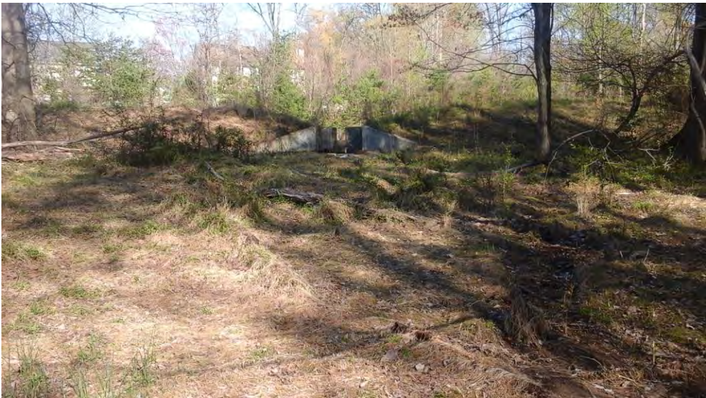
Looking west toward the weir structure from the downstream side.
