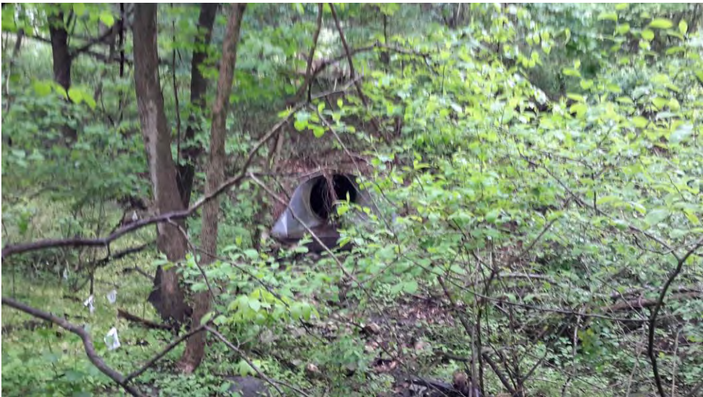
Pond inflow looking south.
