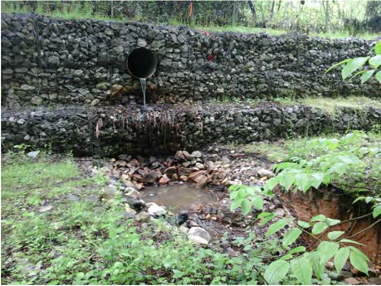
Facing upstream toward outfall and gabion.
