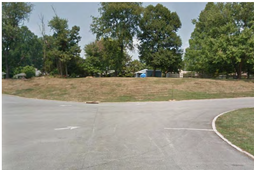
Looking west toward the downstream inlet the bioswale underdrain should tie into.
