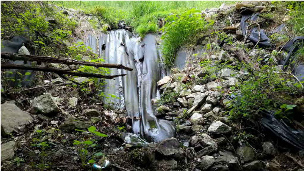
View facing upstream outfall channel at confluence with stream.
