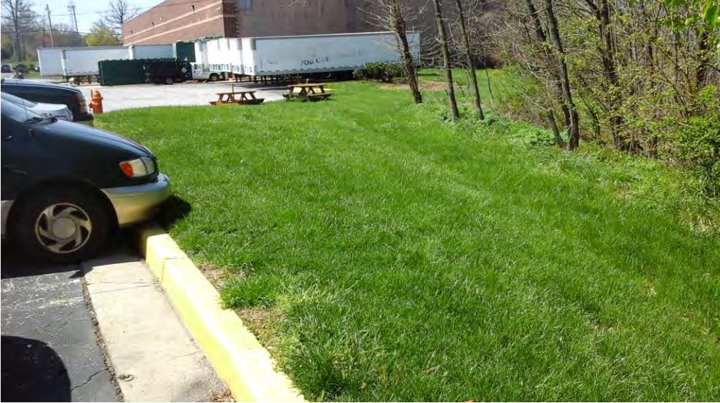
Looking west toward the upstream area of the existing swale.
