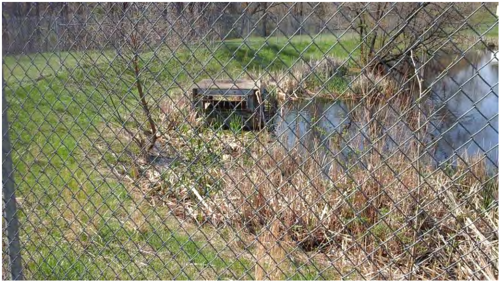
Looking west toward the riser structure and embankment.
