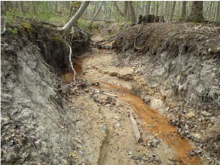
Typical erosion on both banks.
