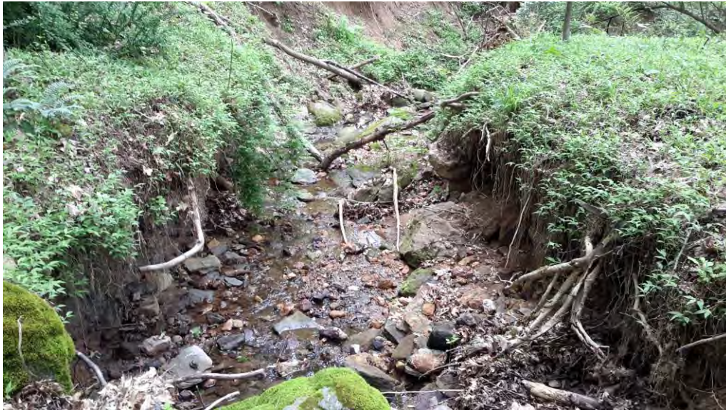
Facing downstream showing typical erosion in the site
