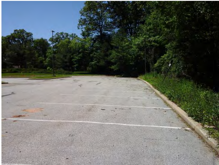
Parking space along the back of the parking lot that can be removed for bioretention
