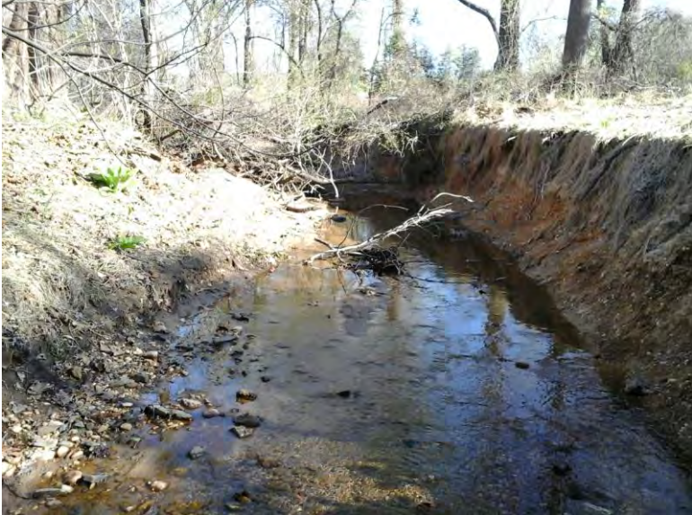
Typical erosion along the downstream extent.
