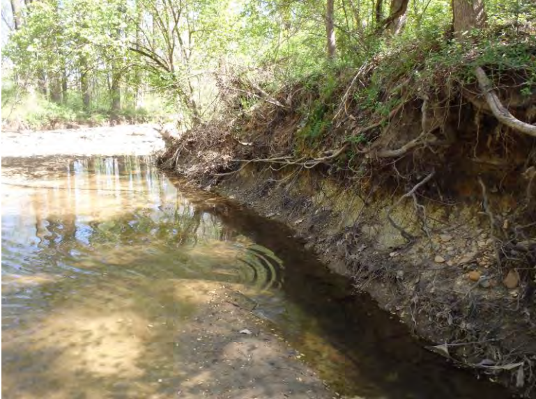
Moderate bank erosion.
