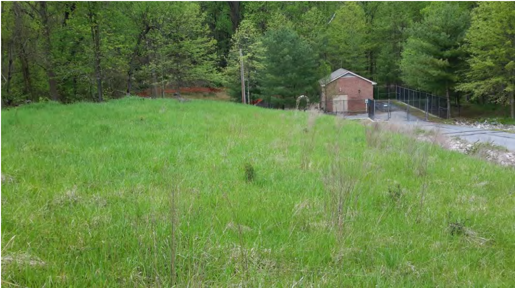
View facing west and downslope of open planting area and pumping station.
