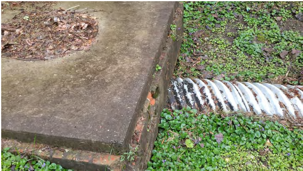
Existing riser structure and inlet.
