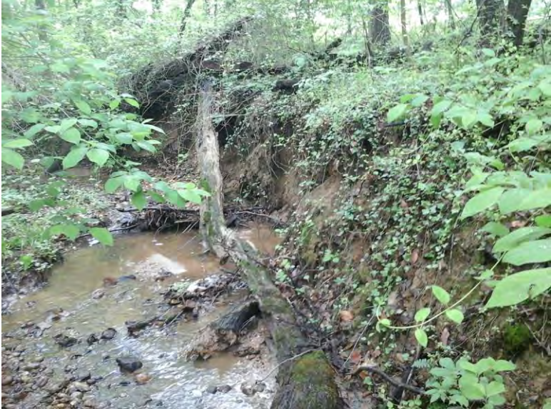
Looking upstream from downstream extent toward typical bank erosion.
