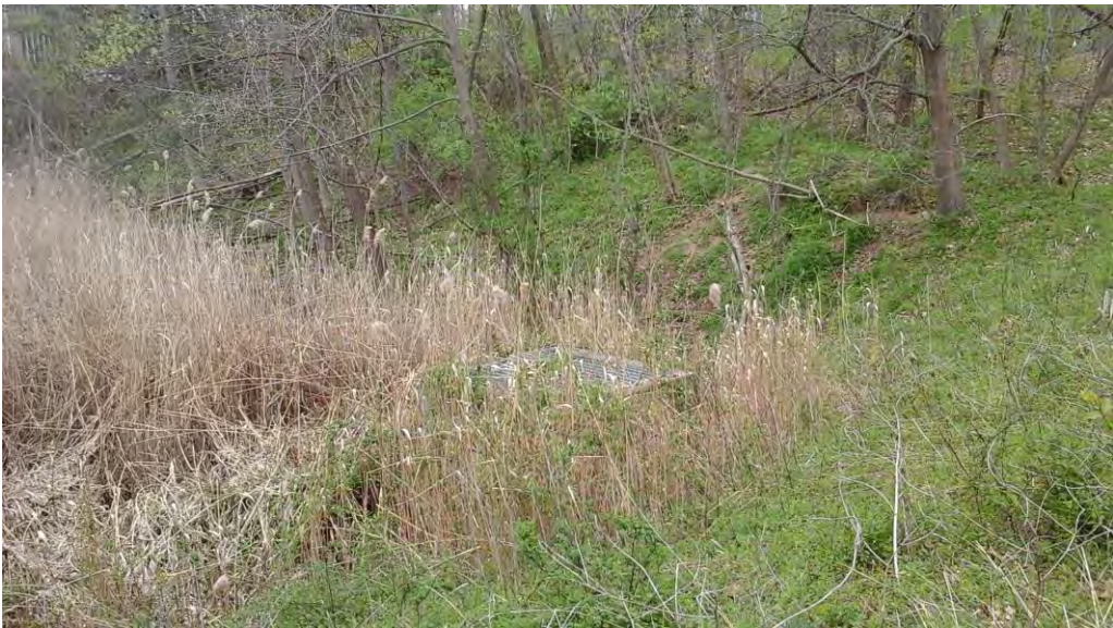
Looking northwest at the riser structure from the embankment.
