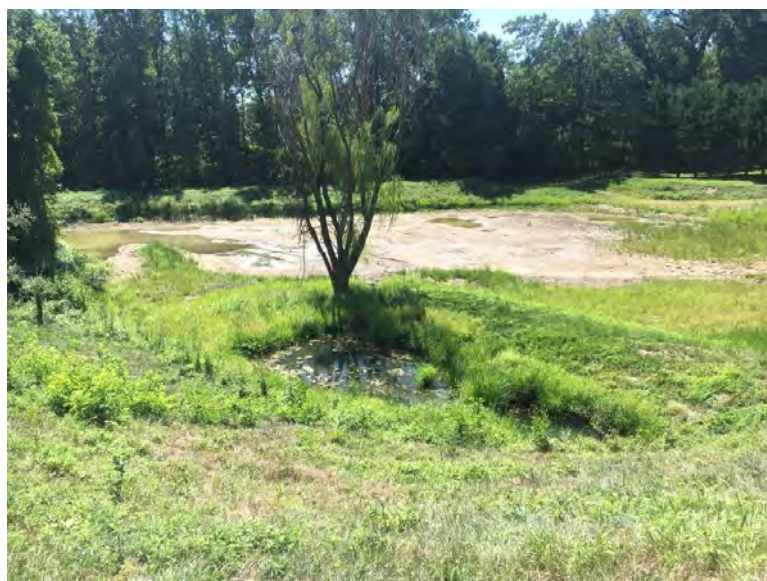
Forebay and pond view from Karas Walk.
