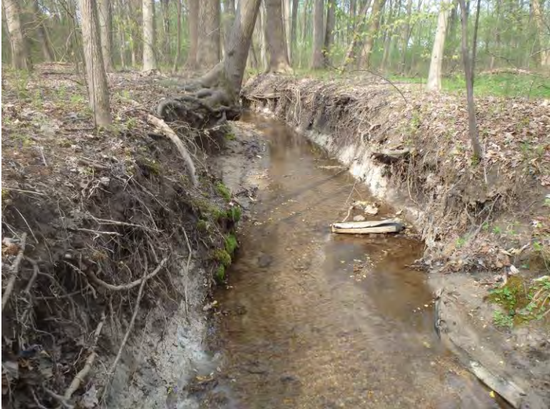
Typical erosion throughout project site.
