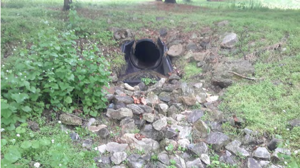
View of outfall pipe structure.
