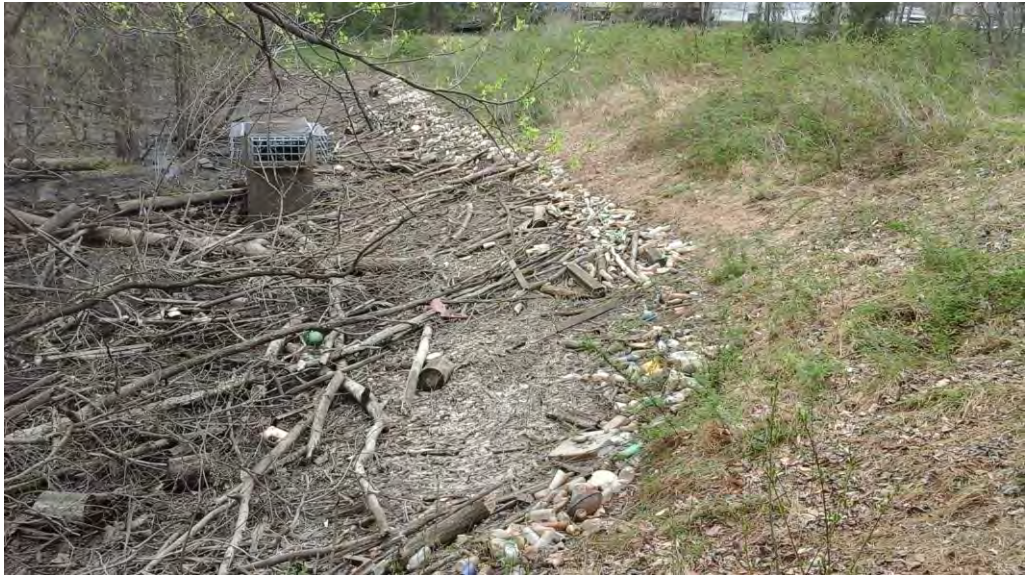
Looking north along the embankment toward the riser structure.
