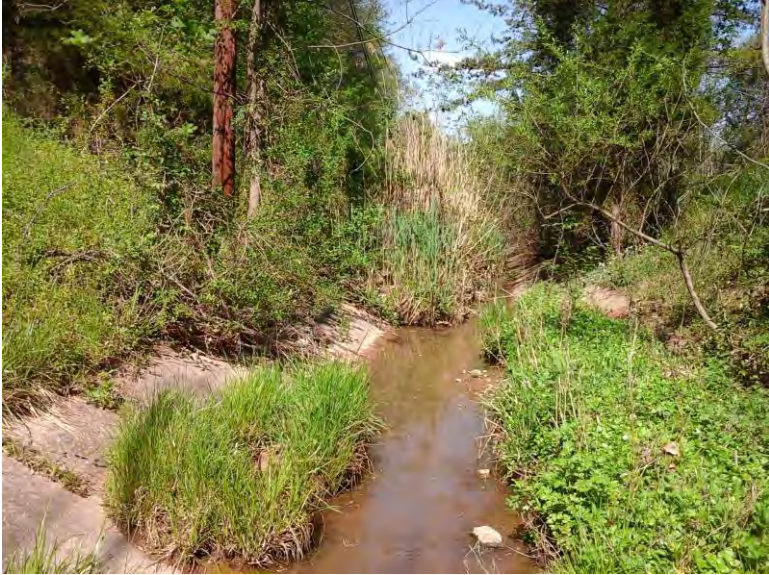
Concrete channelization with wetland vegetation.
