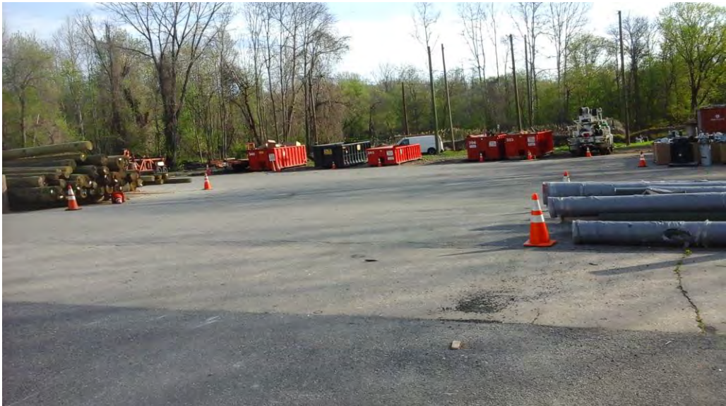
Looking northeast toward the back of the property from the parking lot (LNB-NB-502A).
