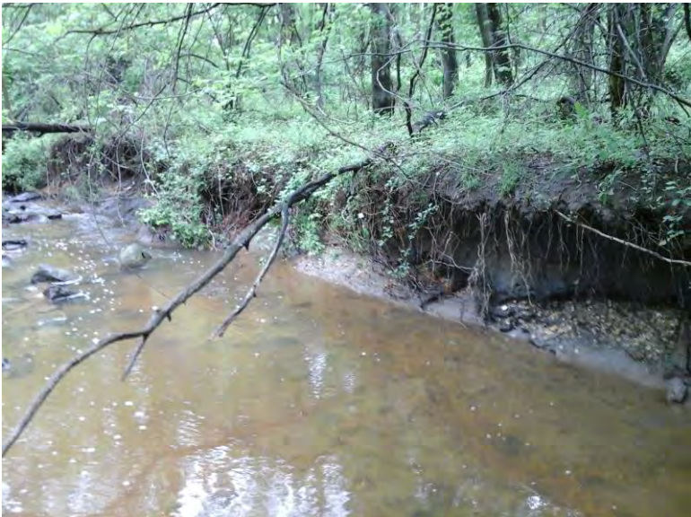
Typical erosion at upstream extent of site.
