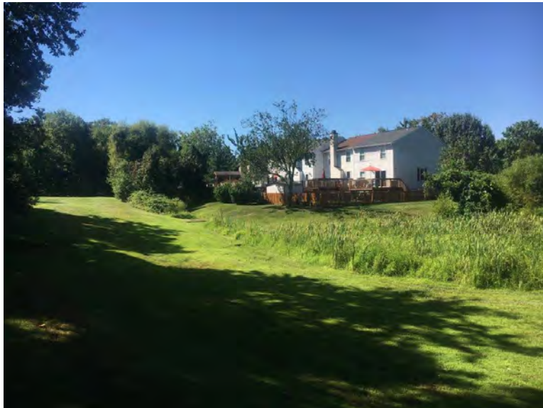
Pond view from downstream berm.
