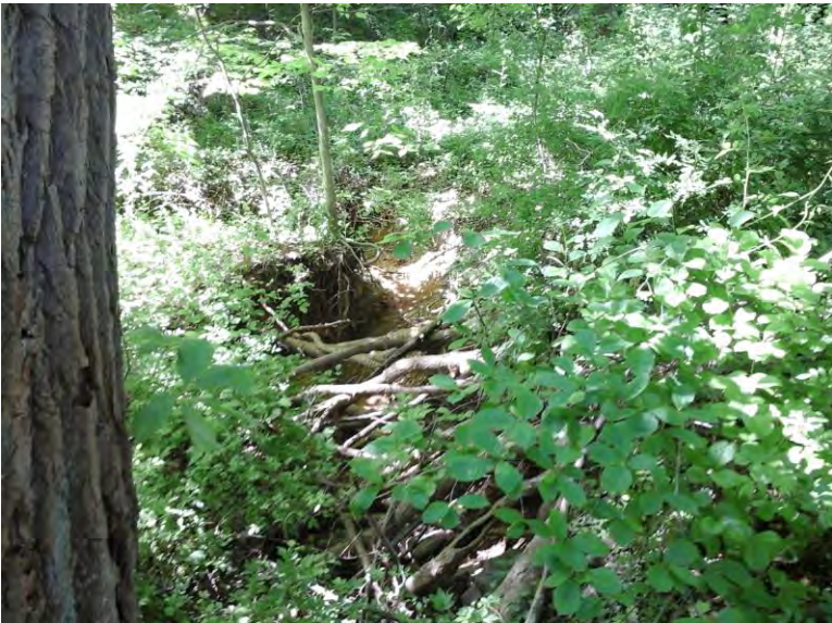
Eroded channel at site LNB-NB-F609a
