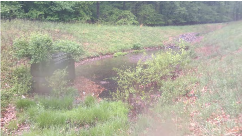
Overview of pond and riser structure looking southeast.
