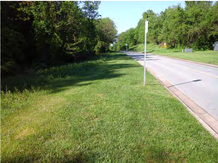
Existing grass area for proposed swale, LNB-NB-F607d
