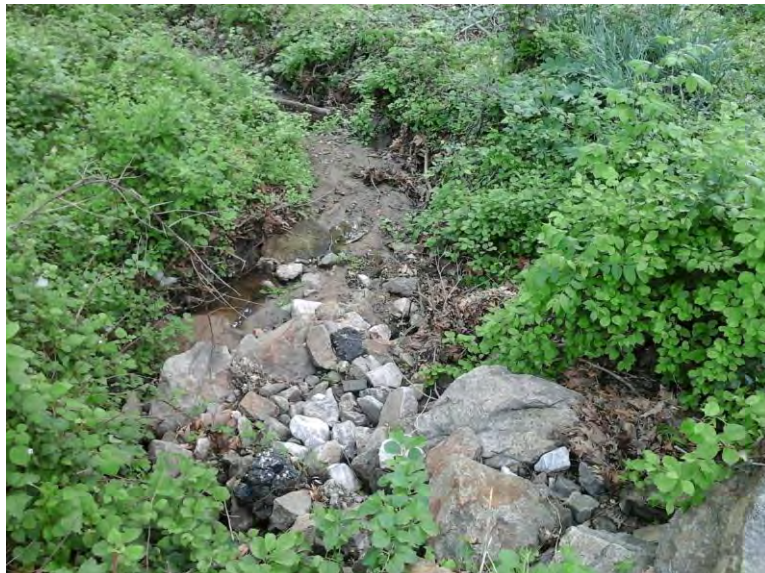
Facing downstream toward end of riprap stabilization in outfall channel.
