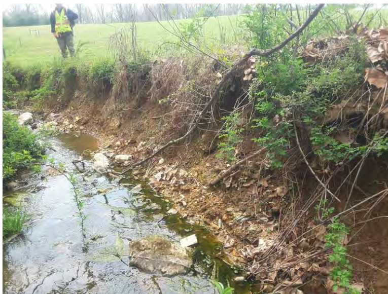
Photo facing downstream at left bank showing moderate erosion with no riparian forest buffer.
