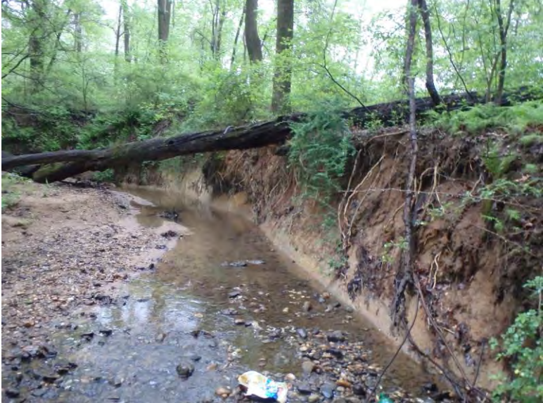
Erosion in east reach.
