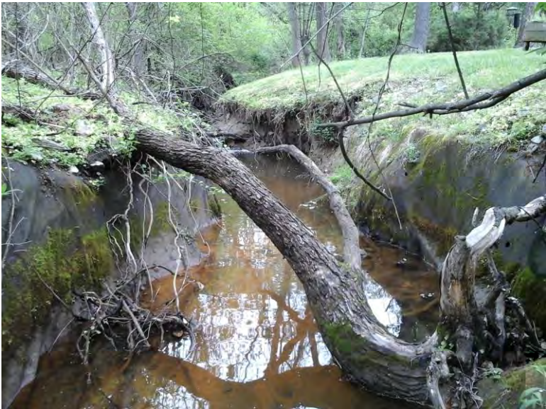
Downcutting threatening sewer crossing and private property.
