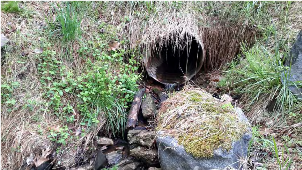
View facing upstream pipe outfall.
