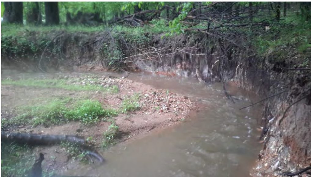
Typical stream bank erosion in the middle portion of the site
