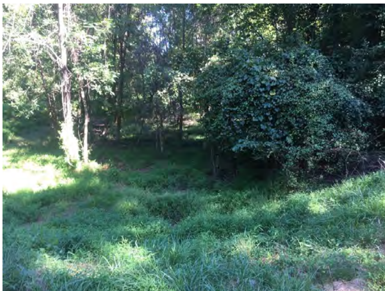
Upstream view of pond inflow ditch.
