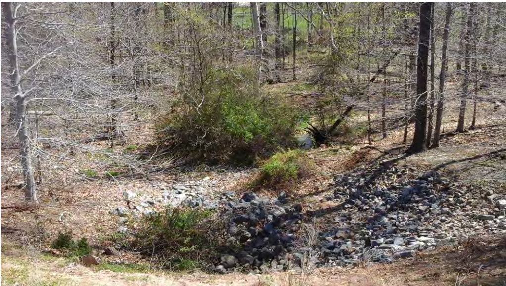
Looking east at the pond outfall from the embankment.
