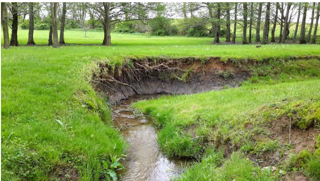
Facing the right bank, significant erosion cutting into a bank along an outside meander, showing tree roots are not fully capable of stabilizing the banks.
