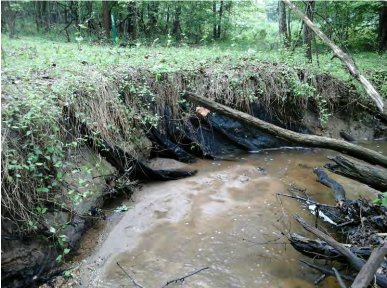
Typical erosion in downstream extent.
