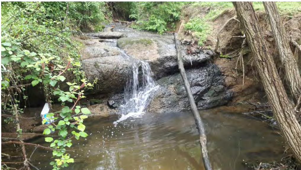
Facing upstream a cascade over bedrock near the downstream end of the site
