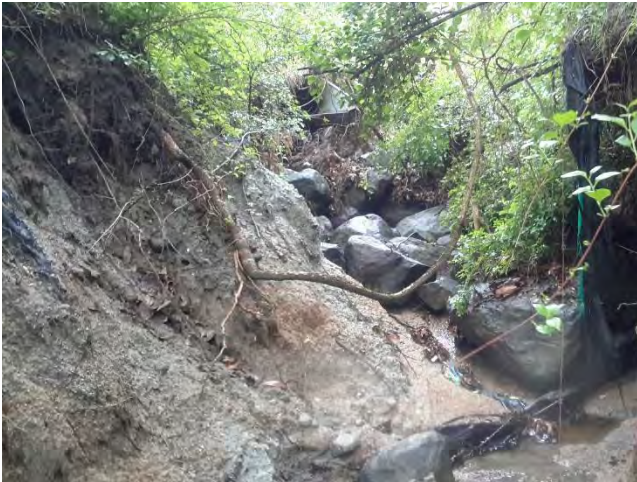
Figure 17. Typical outfall stabilization recommendation sites
