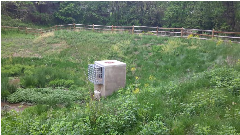
Pond riser structure looking north.
