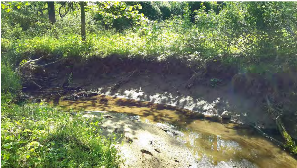
Typical eroding banks, facing right bank
