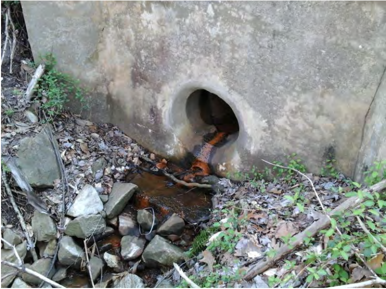
Facing upstream toward outfall.
