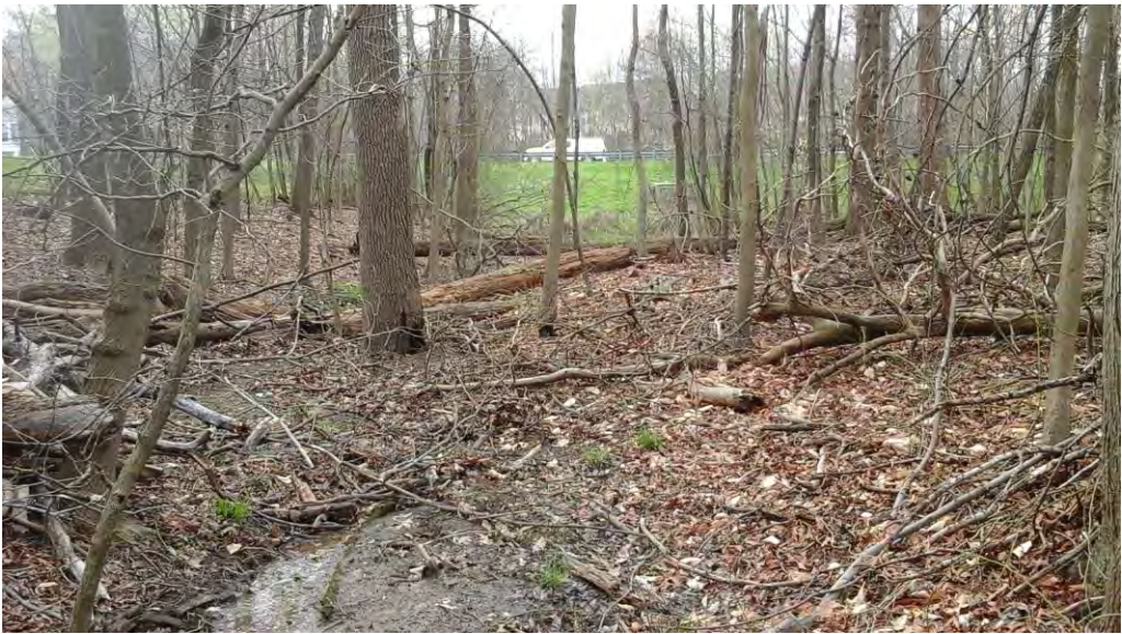
Looking south toward the riser and embankment (Greenmount Drive) from inside the facility bottom.
