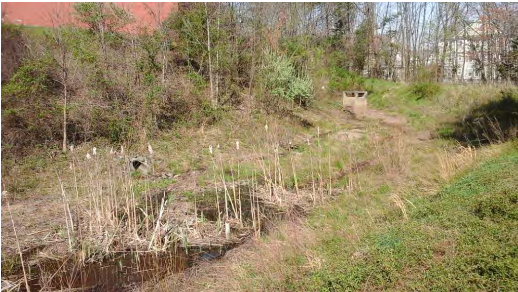
Looking north toward the riser structure and embankment.
