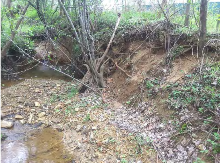
Photo facing upstream at 3.5' headcut showing the left bank erosion as a result of the headcut.
