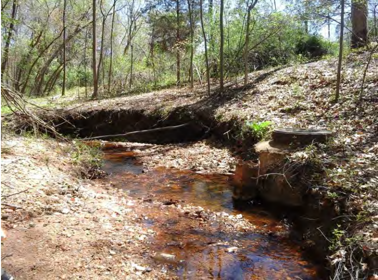
Threatened manhole in southern reach.
