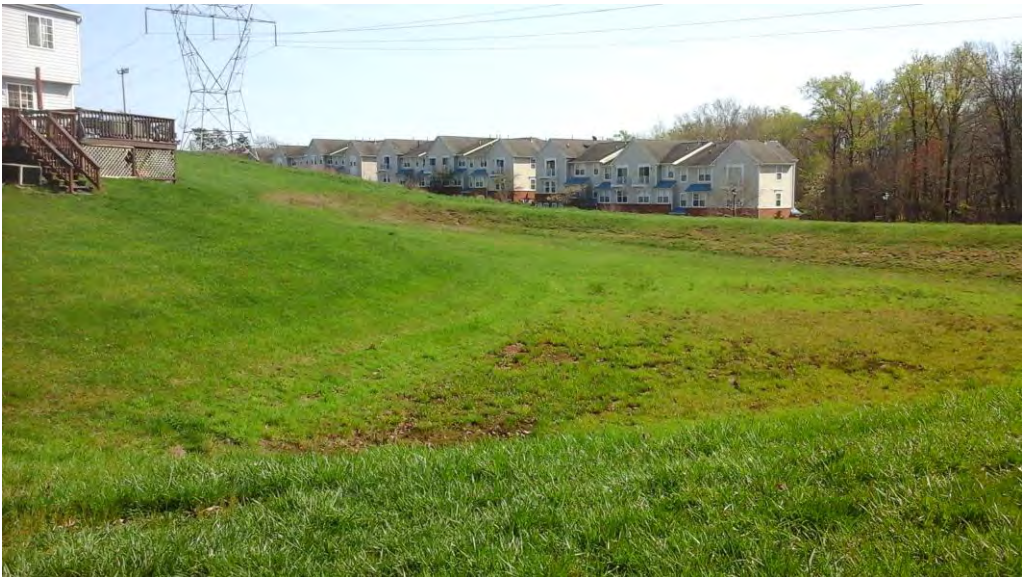
Looking southeast toward the pond area, inflow swale, and embankment from the outfall end section.
