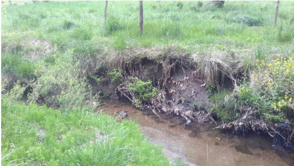
Typical stream bank erosion on the left bank
