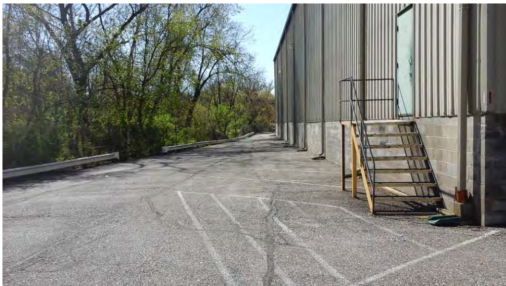
Looking south along the back of the building at the roof drains that will be connected and directed into the proposed facility.
