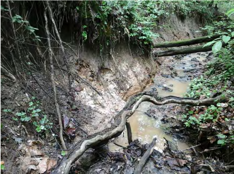
Erosion and headcutting at the upstream extent of the site.
