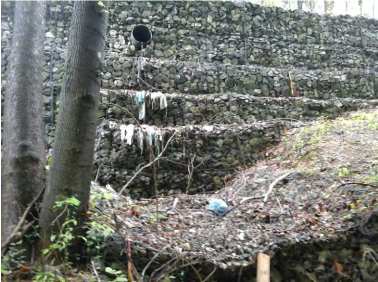
Facing upstream toward outfall and gabion.
