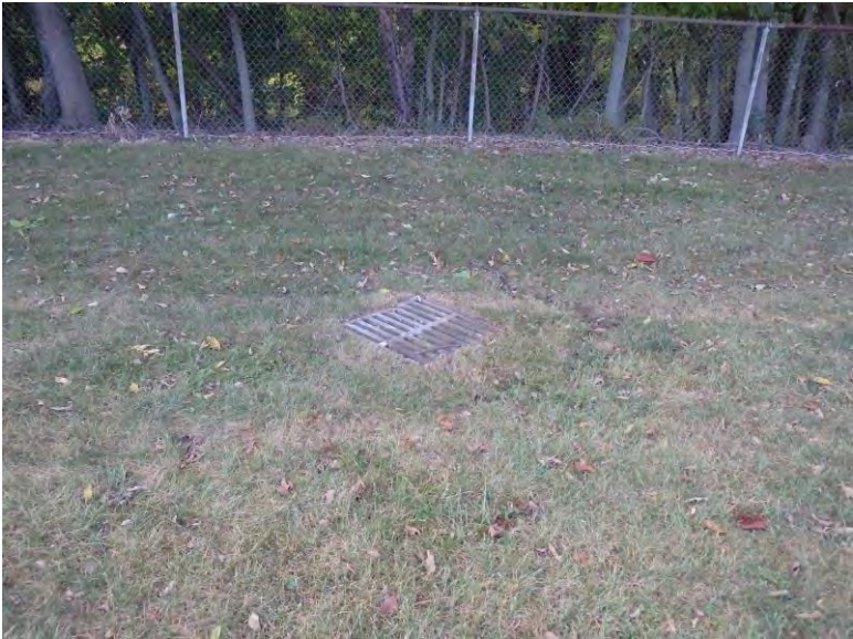
Looking northwest toward the existing inlet.
