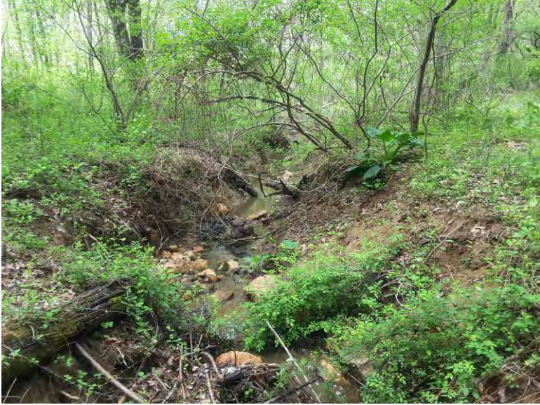
Downstream view of the channel from the outfall.
