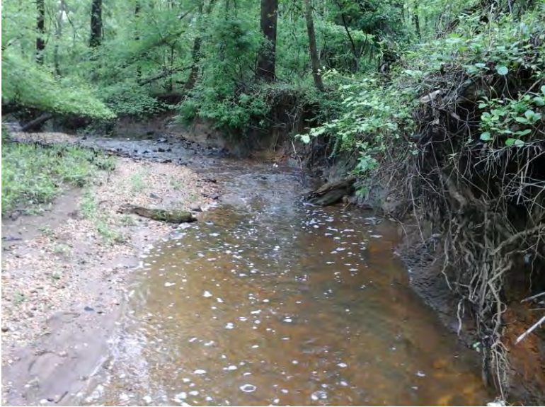
Typical erosion at upstream extent of site.
