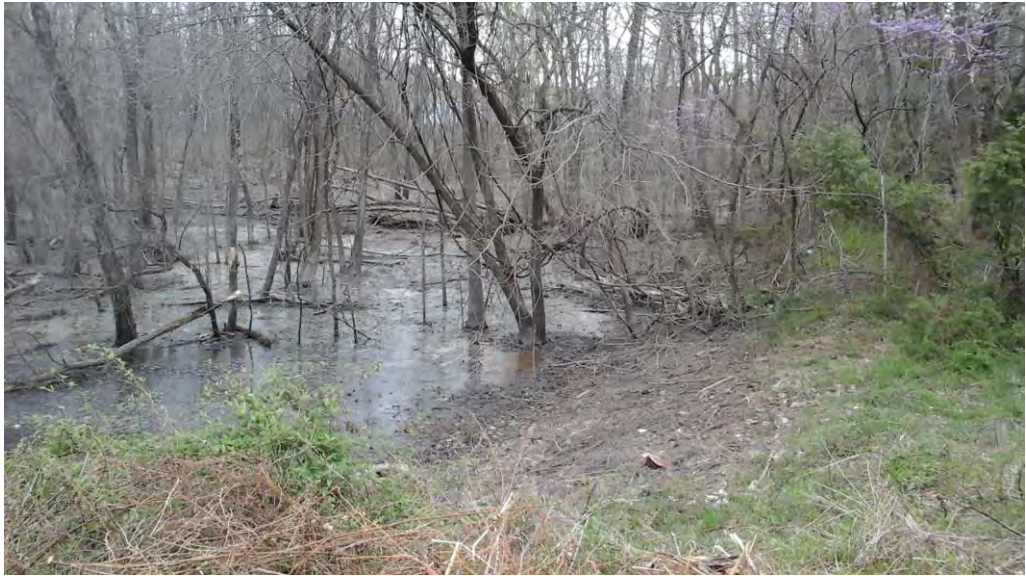
Looking west toward the pond area from the emergency spillway/embankment.
