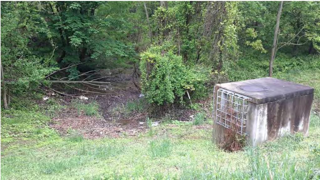
Overall view of pond with riser looking west.
