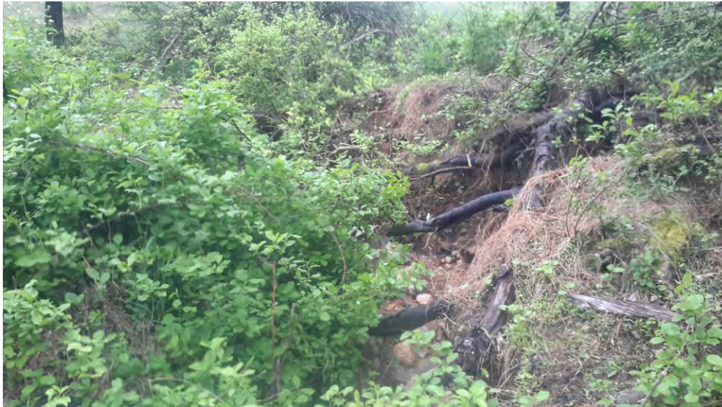
View facing downstream at headcut.
