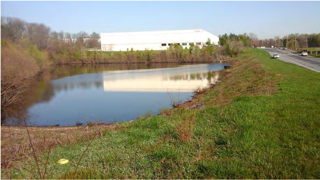
Looking northwest along the embankment toward the riser structure.
