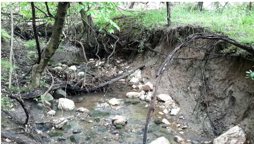
Typical stream bank erosion in upstream portion of site
