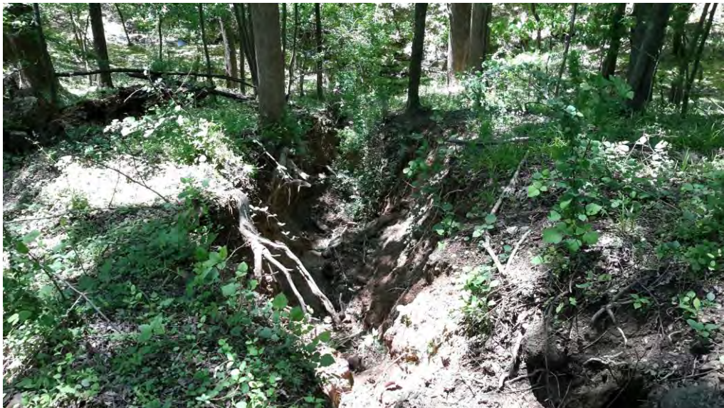
View facing downstream of eroded channel.
