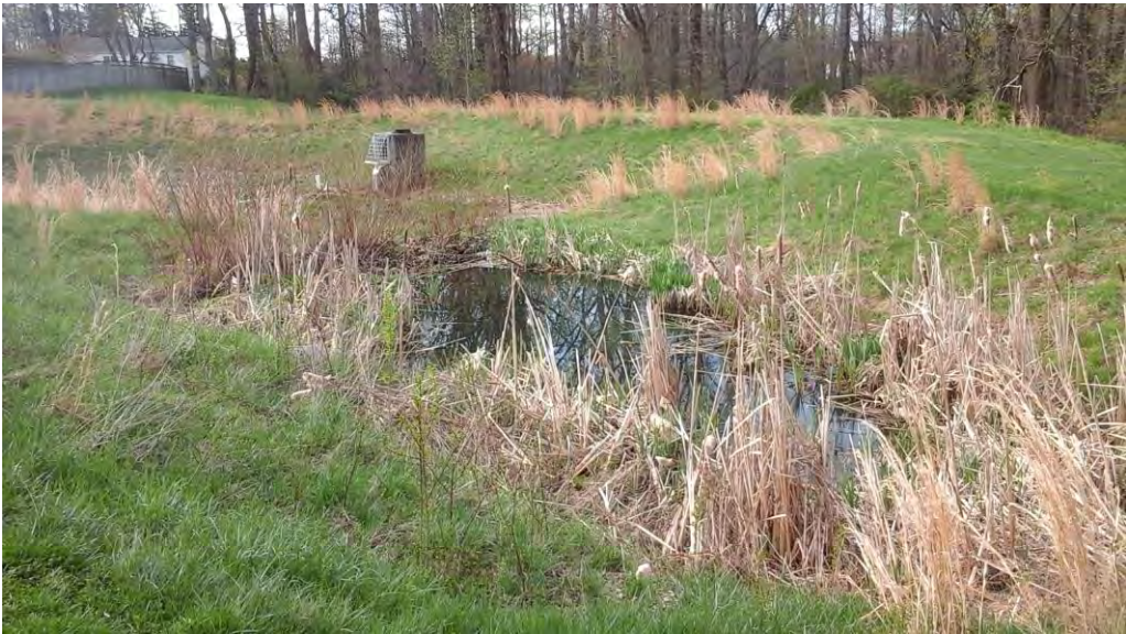
Looking southeast toward the inflow forebay, riser structure, and embankment.
