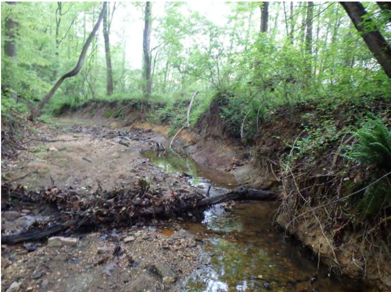
Erosion in west reach.
