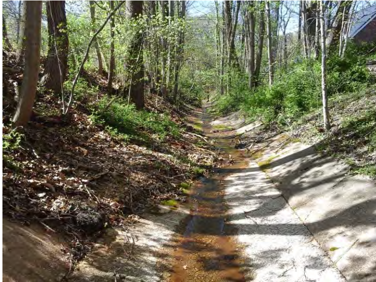
Concrete channel at downstream extent.
