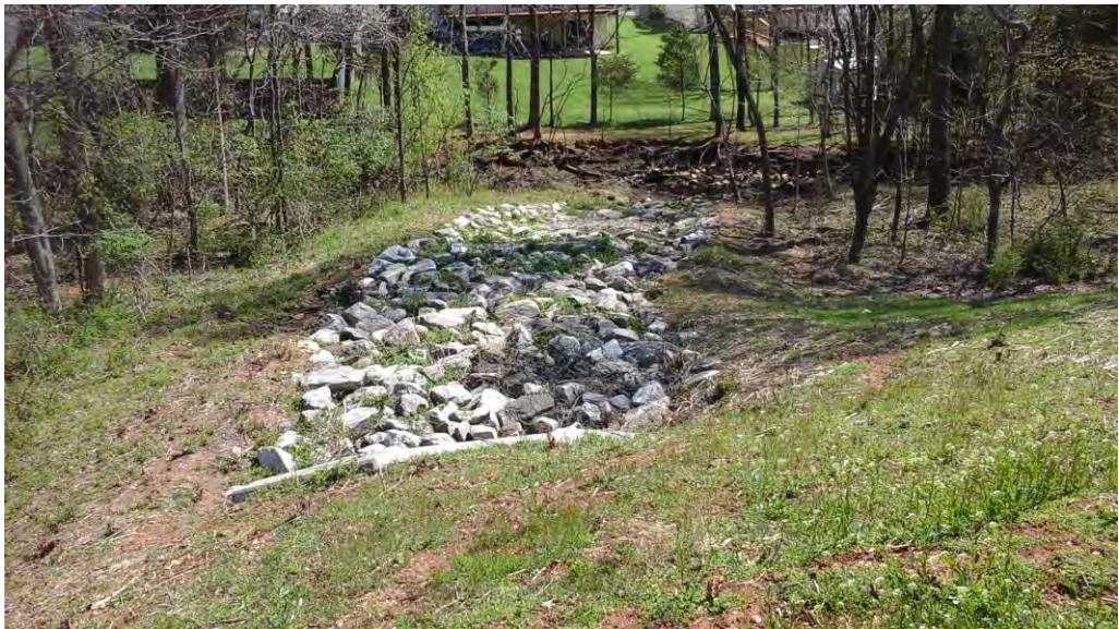
Looking east at the outfall gabion weir channel from the embankment.
