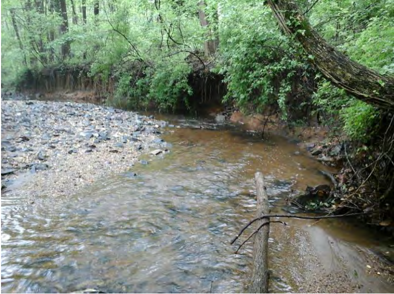
Typical erosion pattern at site.
