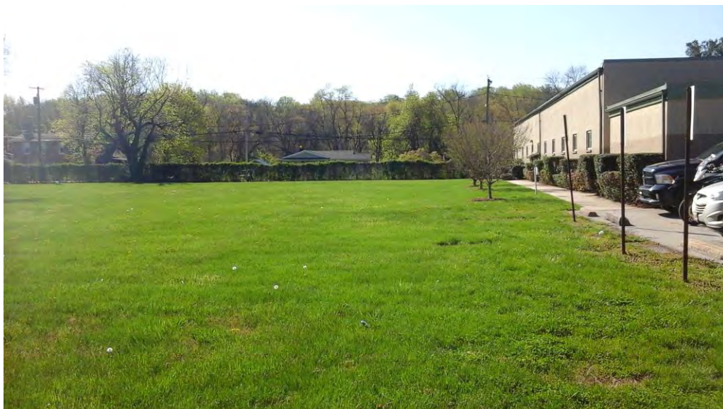
Looking southeast toward the building, roof drains, and grass open space for the proposed facility (LNB-NB-503B).
