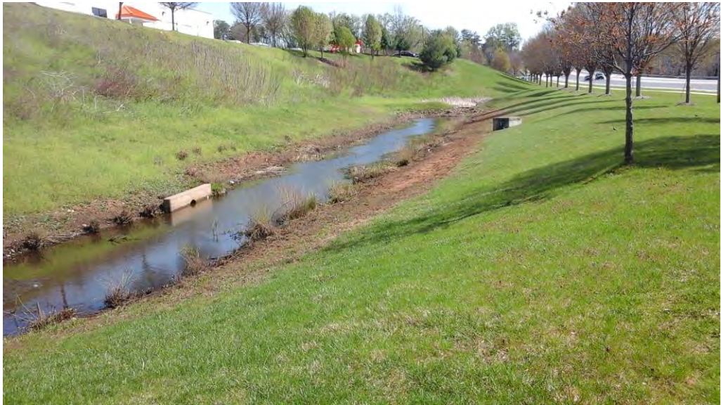
Looking northeast toward the facility showing one of the inflows and one of the riser structures.
