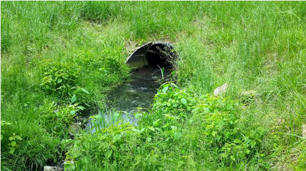
View of outfall pipe.
