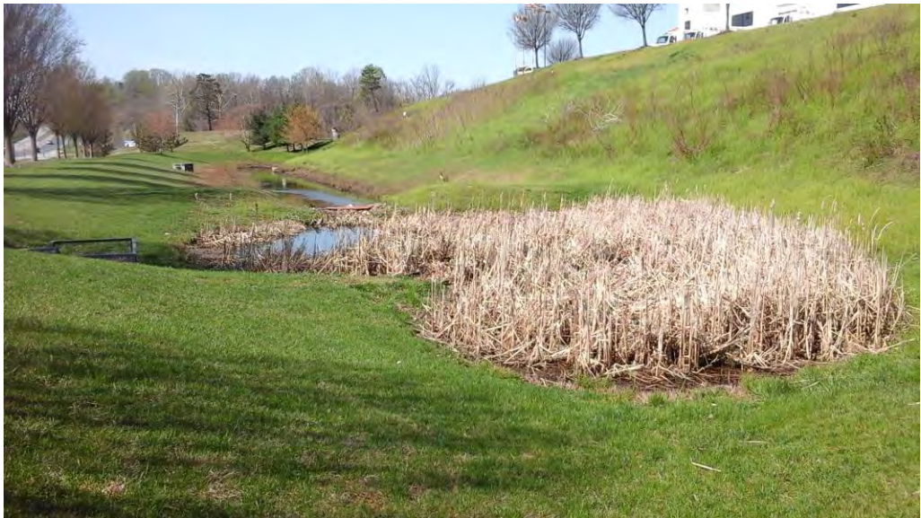
Looking southwest toward the facility showing a second inflow and riser structure.
