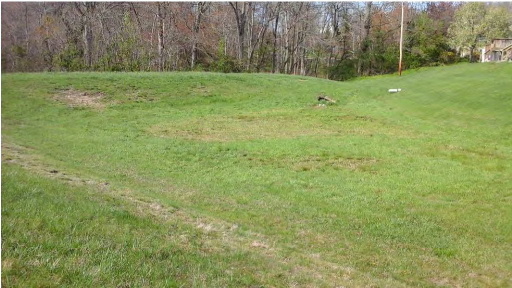
Looking west toward the pond area, embankment, and outfall end section structure.
