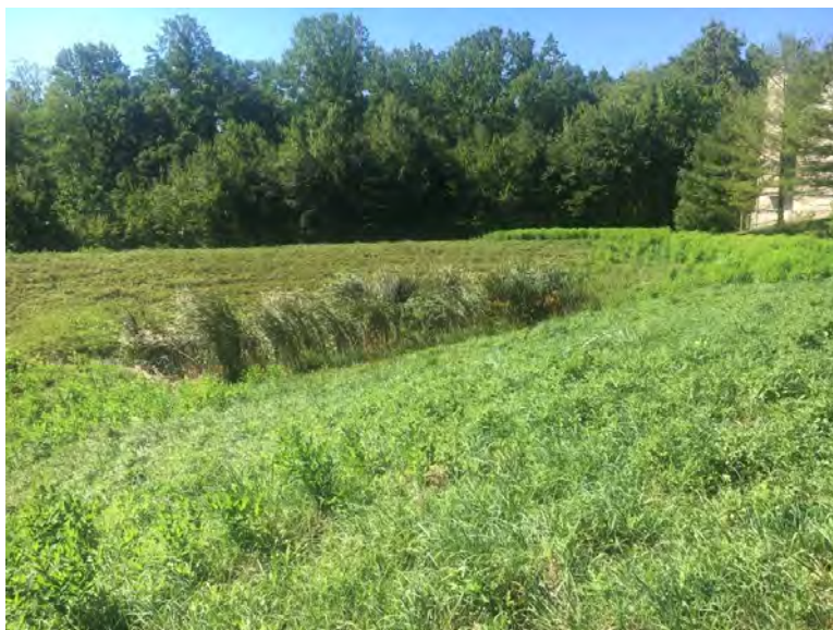
Pond forebay from upslope bank.
