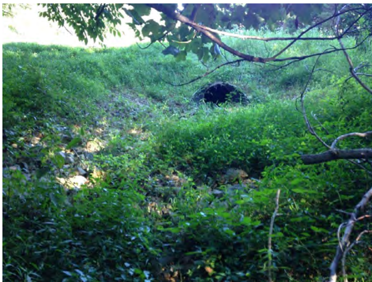
Upstream view of outfall channel.
