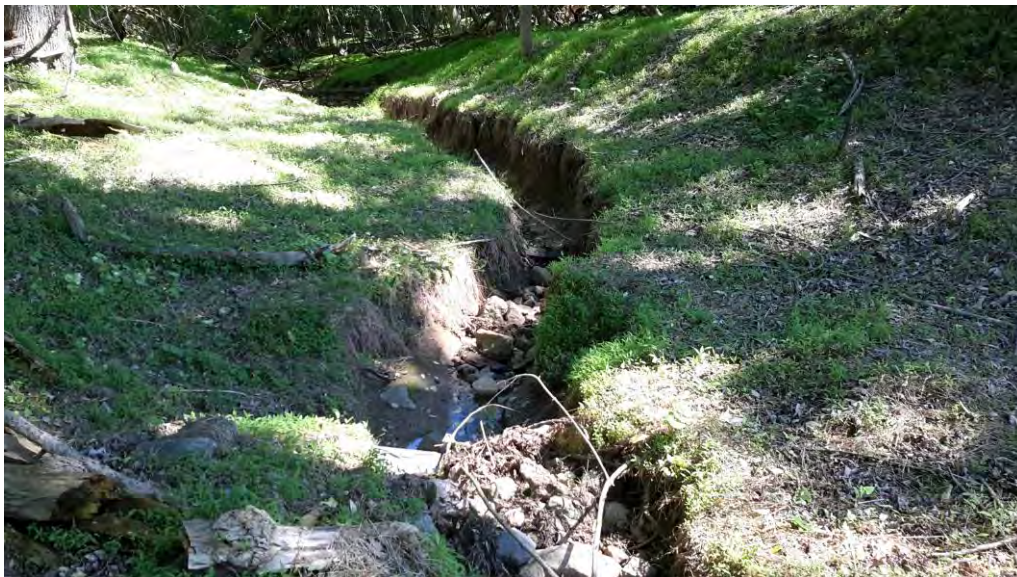
Typical downcutting and bank erosion facing downstream from upstream extent of site
