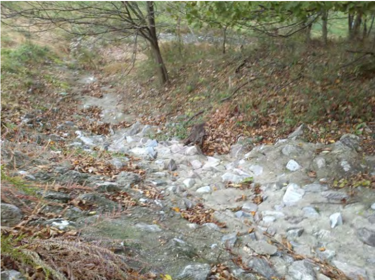
Facing downstream toward grouted riprap outfall channel.
