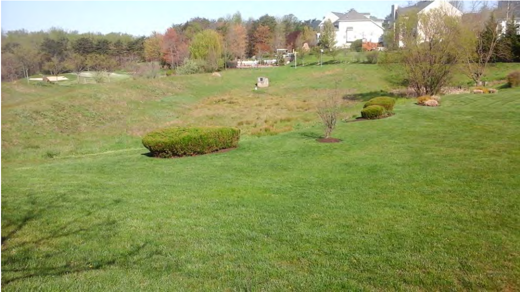
Looking northwest toward the pond from the access path with the inflows and forebay to the right, riser in the center, and embankment on the left.
