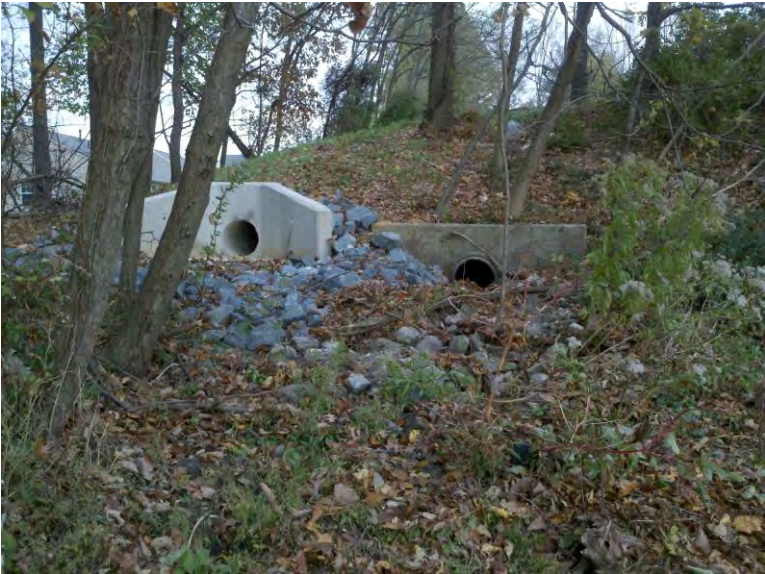
Facing upstream toward stormwater outfalls and headwalls.
