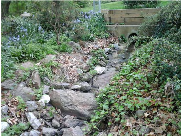
Facing upstream toward outfall.
