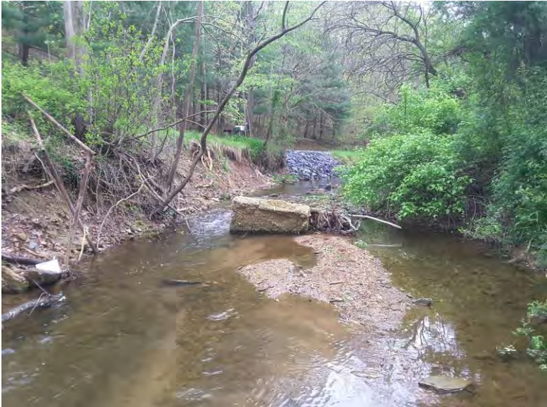
Facing upstream at riprap armored bank.
