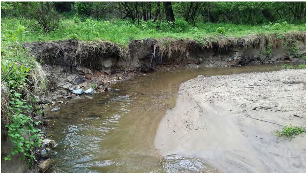
Typical erosion along the right bank
