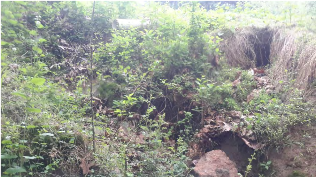
View facing upstream of outfall pipe of center channel.
