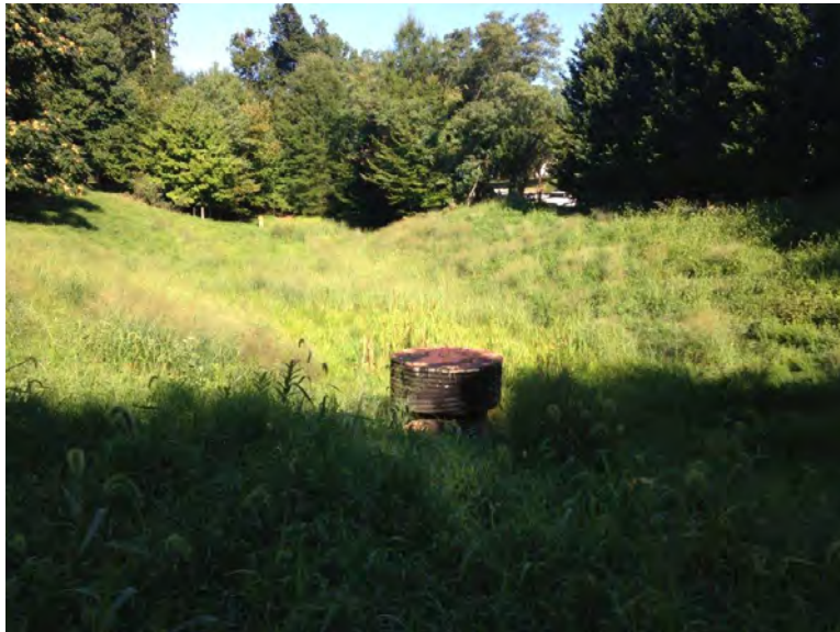
Pond view from riser side berm.
