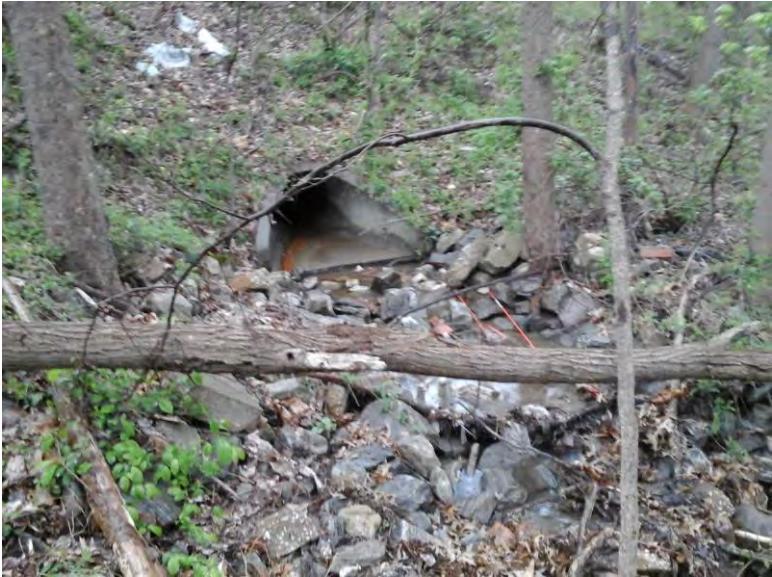
Facing upstream in outfall channel toward pipe.
