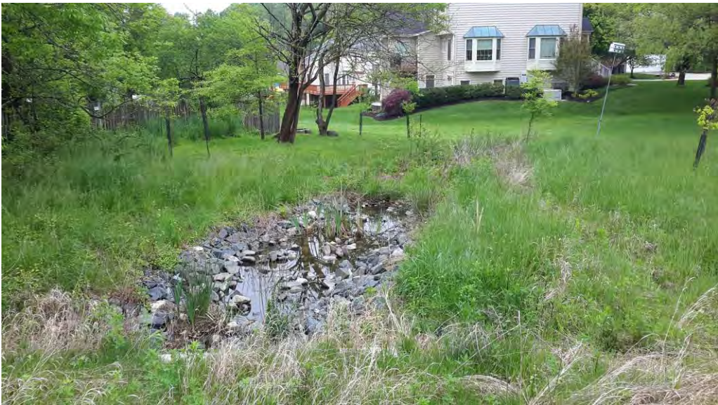
Pond outfall looking north.
