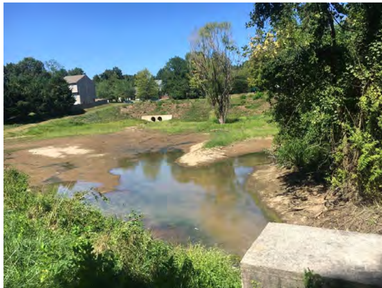
Overall pond view from outlet structure.
