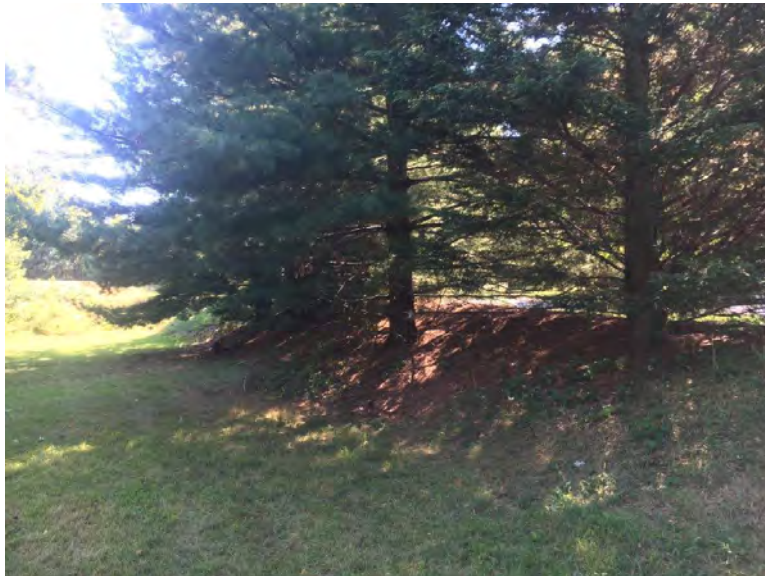
Downstream view of earthen berm.
