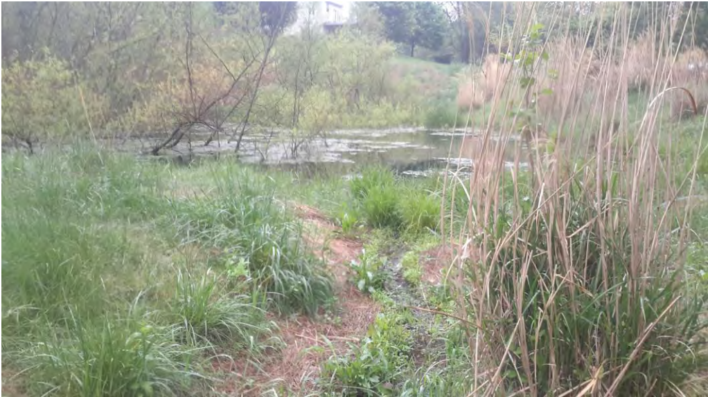
View of spillway with erosion facing south.
