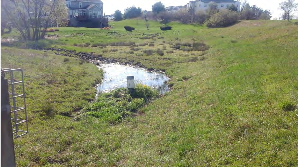
Looking southeast toward the access path, pond area, and low flow standpipe from the riser structure.
