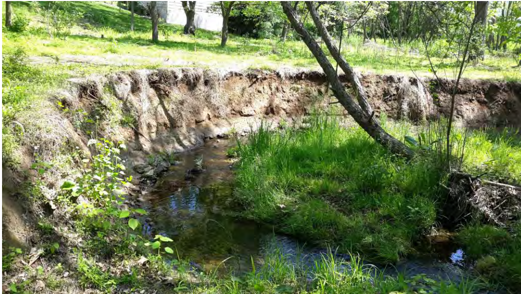
Typical eroding banks, facing left bank
