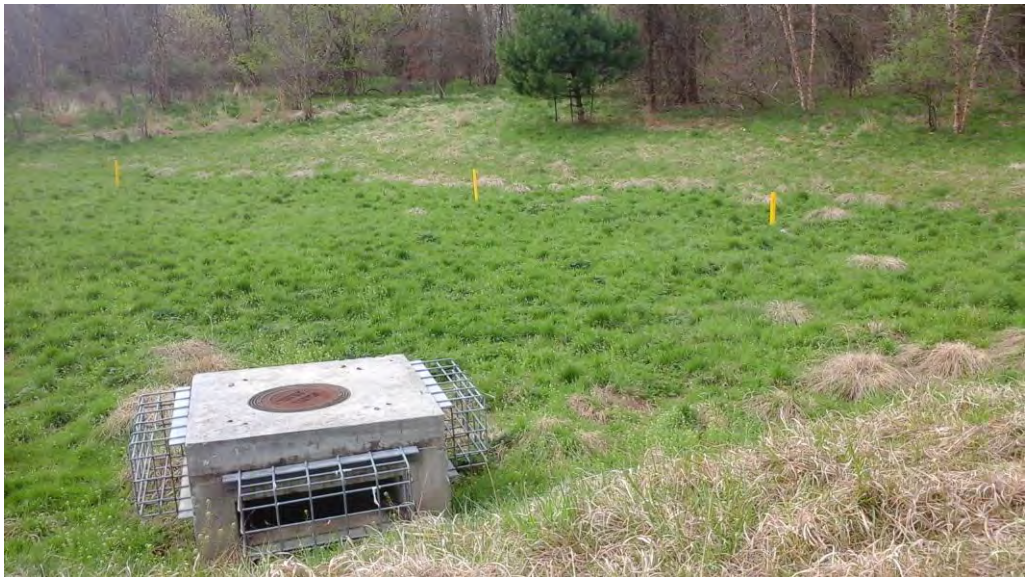
Looking south toward the riser, upland area of the pond, and riser structure from the embankment.
