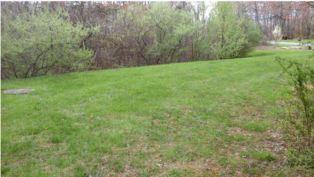
Looking south toward the pond and Meadowridge Road from the embankment near the outlet structure manhole.
