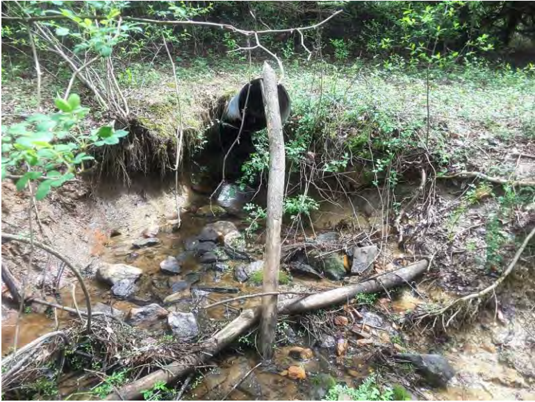
Upstream view of 12 in. CMP outfall barrel.
