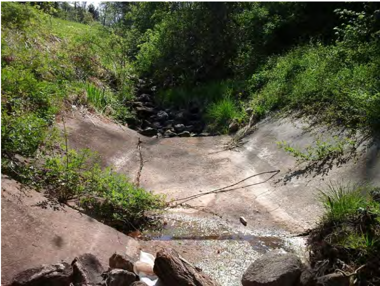
Concrete and riprap channelization at downstream extent of site.
