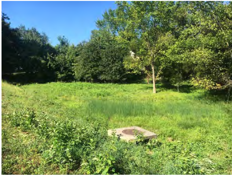
Overall pond view from berm.
