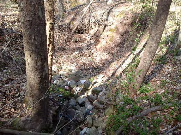
Facing downstream toward outfall channel.
