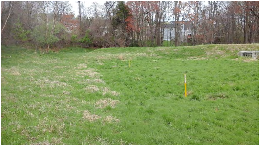
Looking north toward the emergency spillway (left), embankment, and riser structure.
