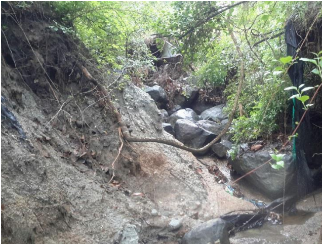
Figure 18. Typical outfall stabilization recommendation sites
