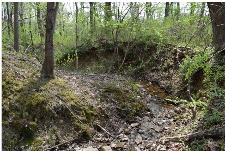
Severe bank erosion on the outside of a meander bend in the highly sinuous portion near the middle of the project reach.
