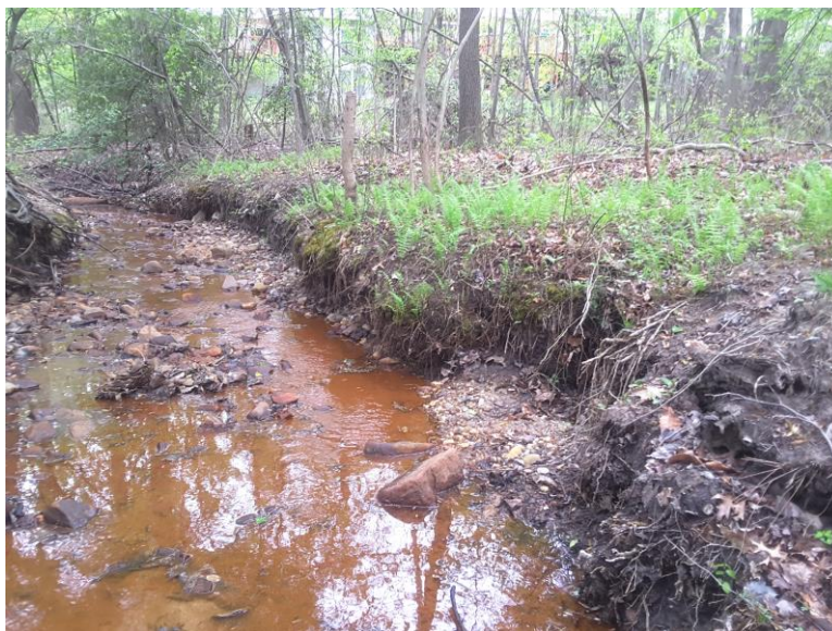
Photo facing downstream of minor bank erosion along the left bank. Forest and vegetative protection helping stabilize the bank.
