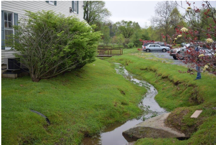
Upstream view of receiving stream with footprint beyond bridge on right bank of stream.
