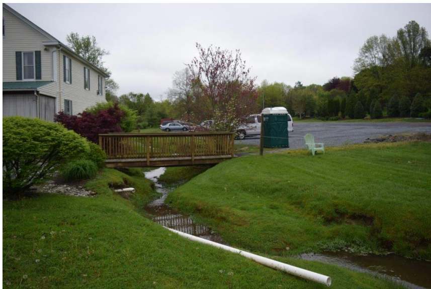
Footprint area, looking north, between gravel lot and stream beyond wooden bridge.
