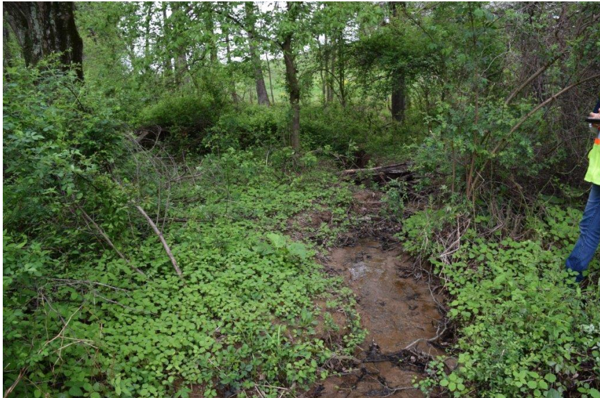
Outfall channel below riprap apron.
