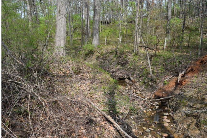
Bank erosion and exposed bed material near the downstream end of the project reach.
