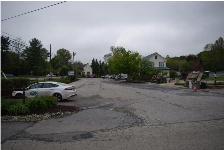
Existing site conditions looking north with Route 97 on the left.
