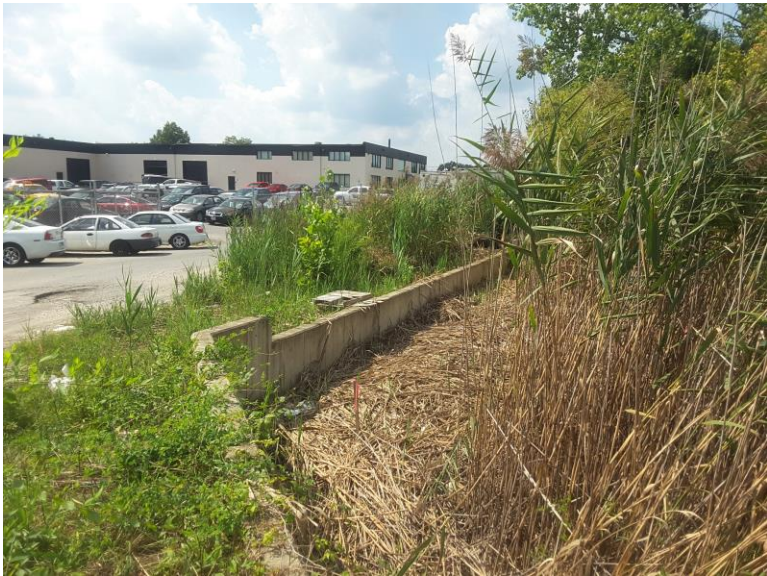
Existing pond weir and concrete embankment
