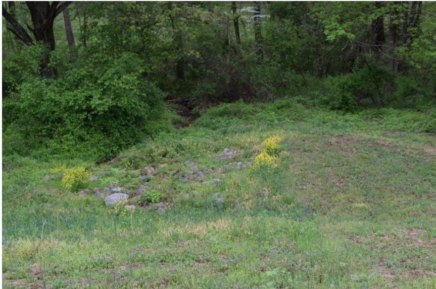
Downstream view of outfall channel from BMP berm.
