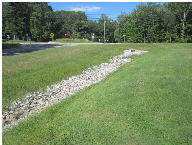
Receiving riprap ditch.
