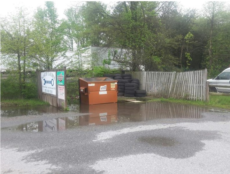
Potential micro-bioretenion site with ponding evident
