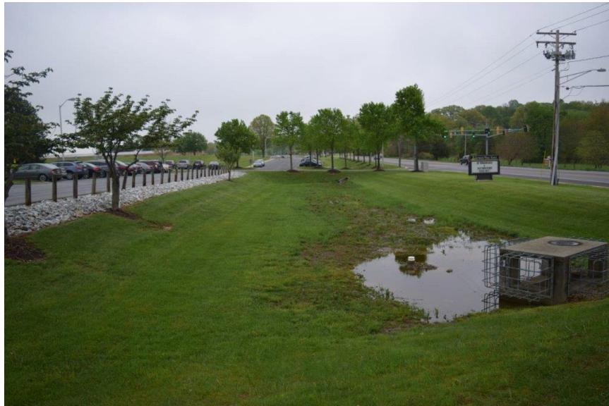
Overall pond view from south berm.
