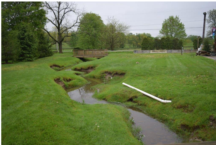
Downstream view of receiving stream.
