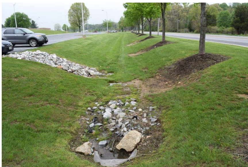
Upstream ditch discharging to pond.
