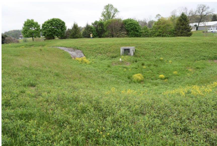
Overall pond view from south.
