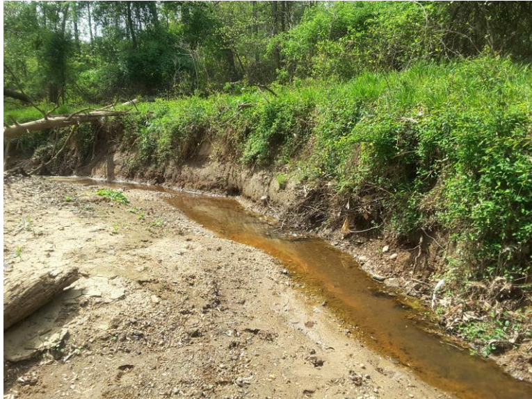
Photo facing upstream showing raw left bank around tight meandering bend.
