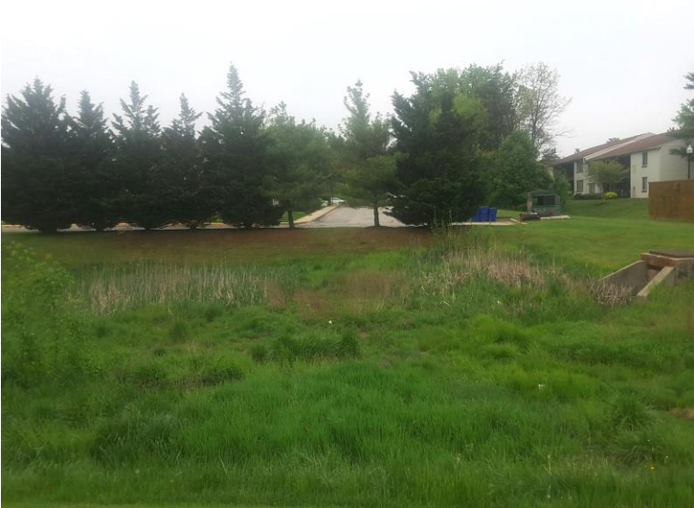
Overview of the facility, including outlet riser structure, looking northwest
