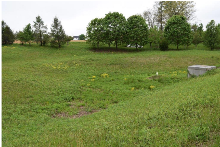
Pond view from emergency spillway.
