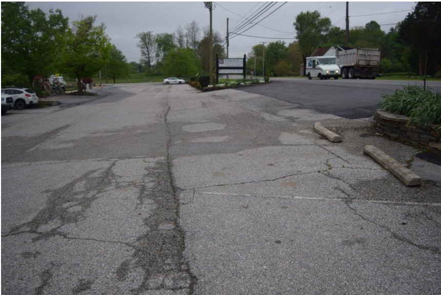
Existing site conditions looking south with Route 97 on the right.
