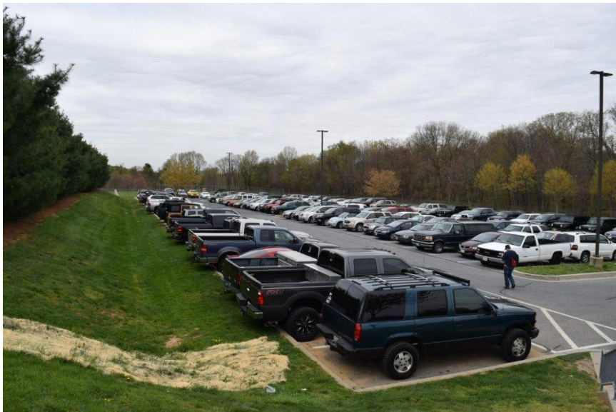
Parking lot draining to existing BMP concept footprint located in back corner of lot.
