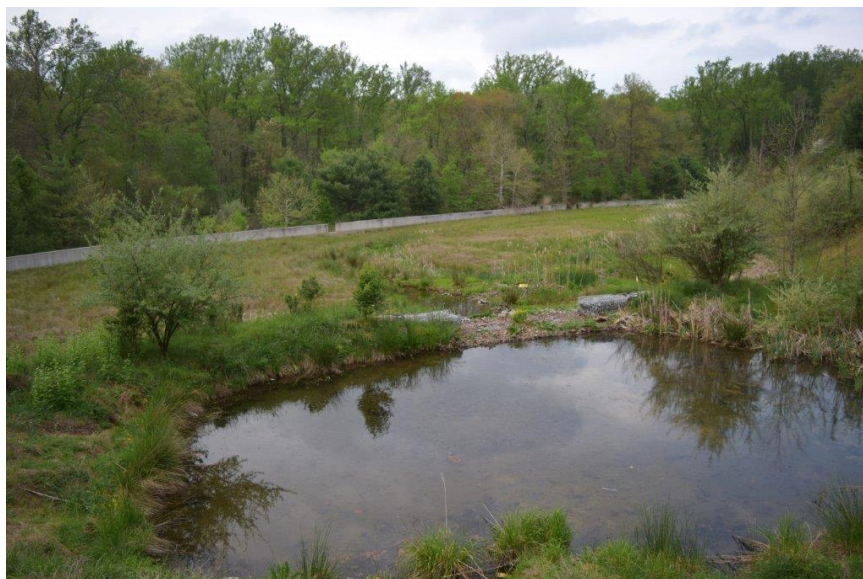
Pond view from forebay bank.
