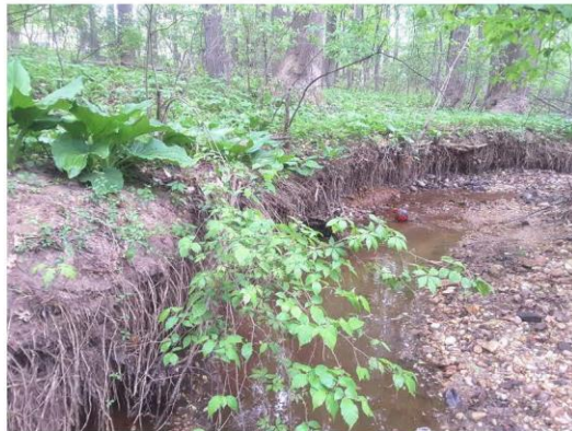
Photo facing upstream assessing the right bank and depicts a typical stream bank within the upstream limits of the assessed stream.
